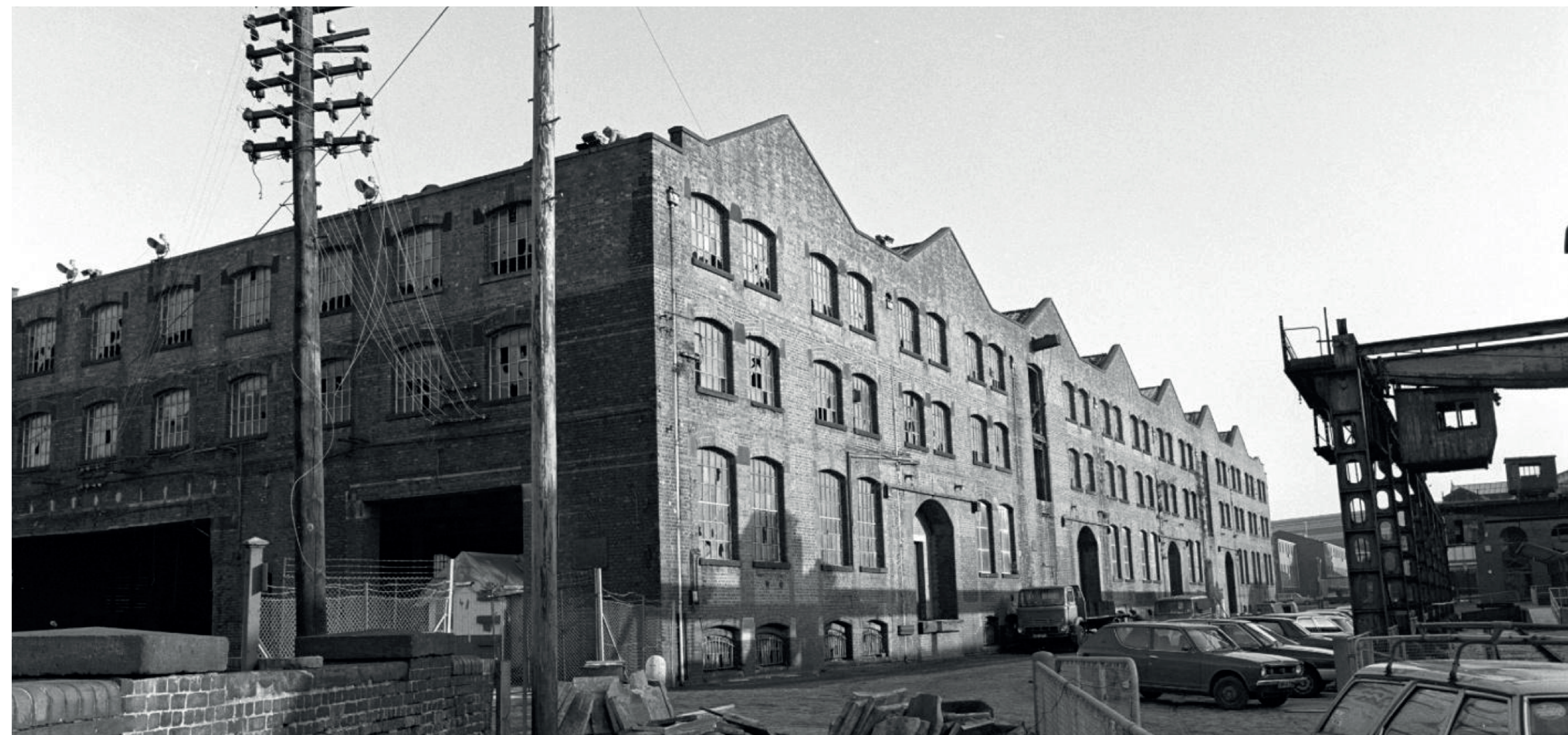
Archive image of the New warehouse c. 1984
