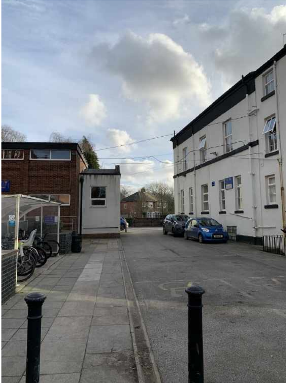
Photograph 5 View south across the eastern part of the site with the Sunbury building in the right of the picture and the neighbouring Xavier Building in the left of the picture.
