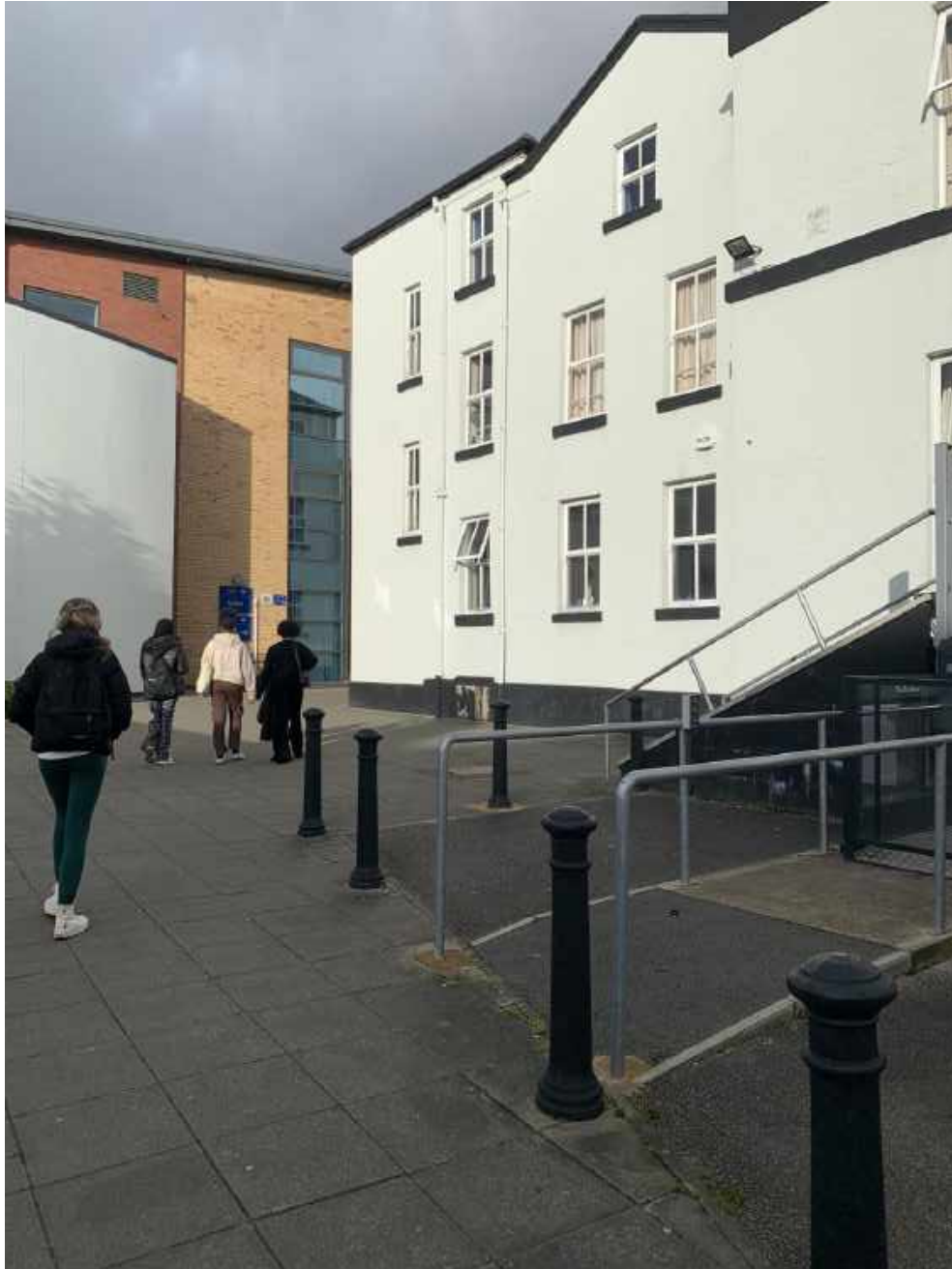
Photograph 3 View north-east towards the western elevation of the existing two / three storey Sunbury Building.
