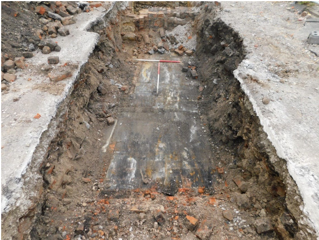
Plate 7: General shot of Trench 4 and York Stone flagged cellar surface {408} to the Welsh Harp pub, looking south-east, scale: 2 x 1m.
