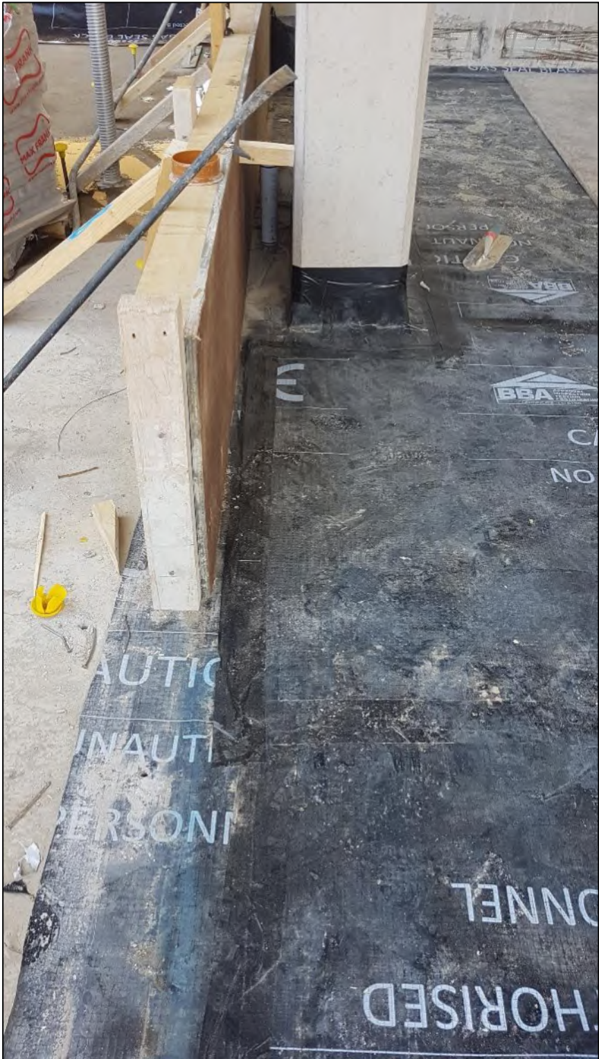
Figure 4: Membrane installation along building edge and columns
