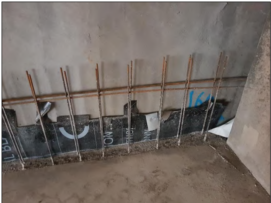
Figure 6: Photo after concrete slab cast in eastern part of building
