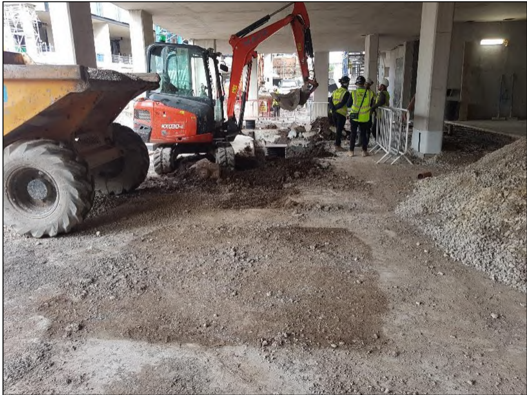
Figure 5: Photo showing area prior to installation
