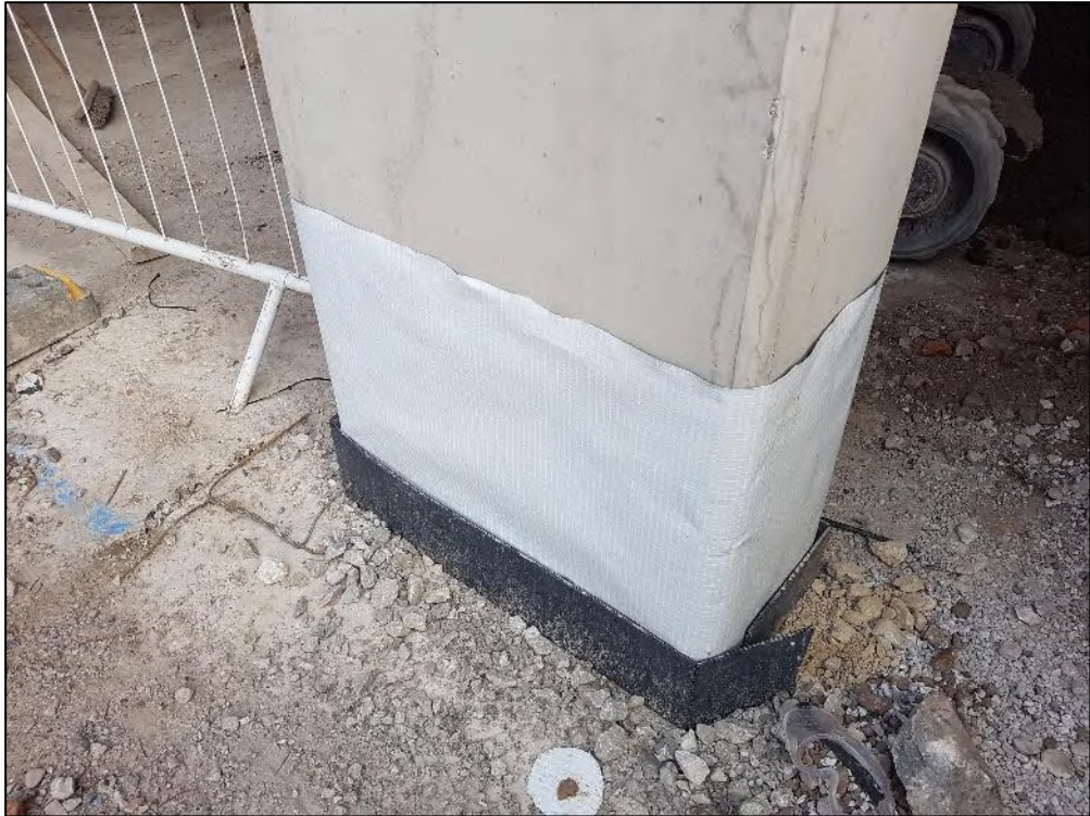
Figure 3: Photo showing area prior to installation
