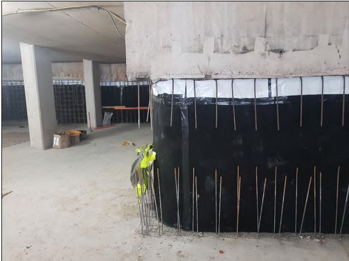
Figure 19: Membrane installation on central corner of config wall which needed repair.
