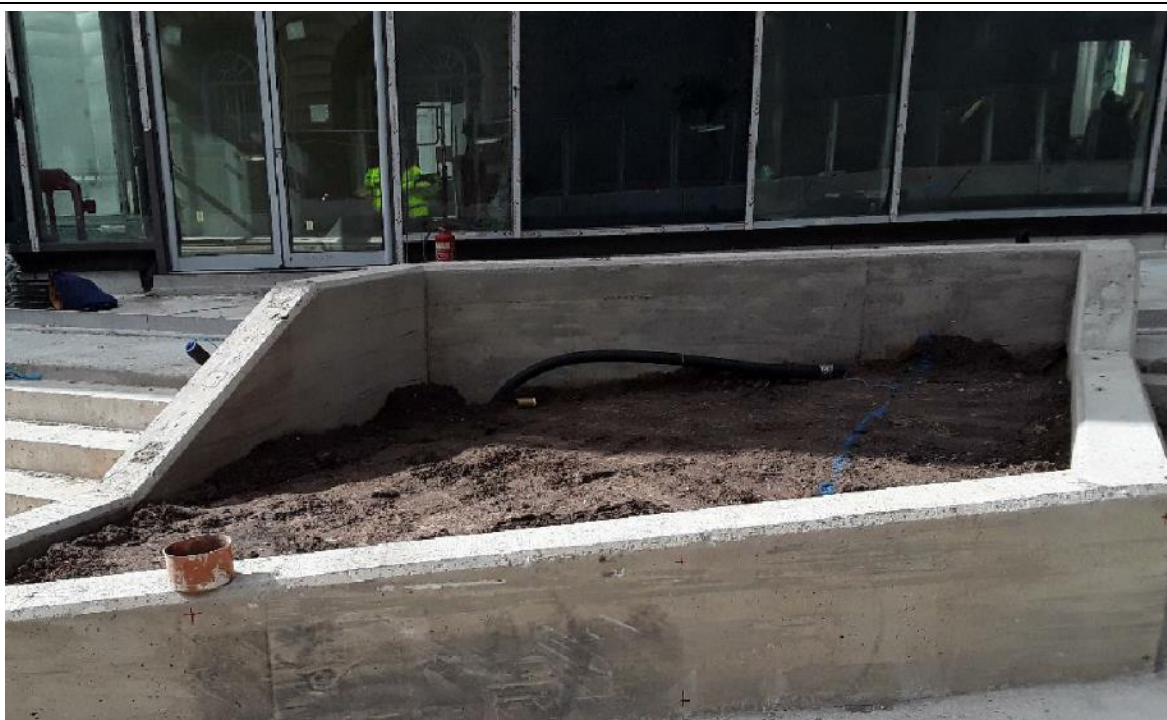
After topsoil installation
