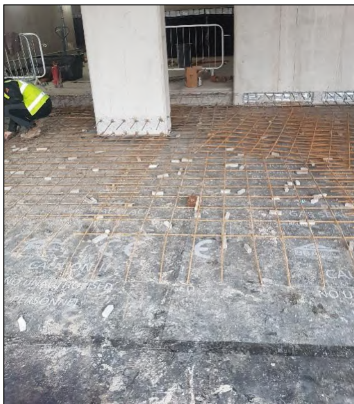
Figure 13: Membrane installed prior to concrete slab casting (central west) – no sharp objects although membrane not completely clear. No tears were noted.
