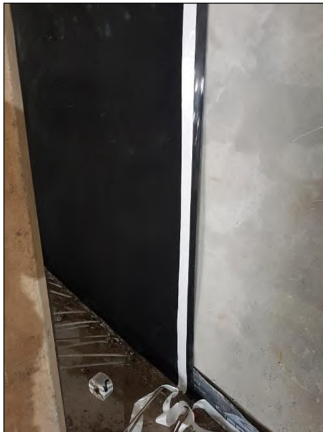
Figure 8: Membrane along contig pile wall in NE part of the site.
