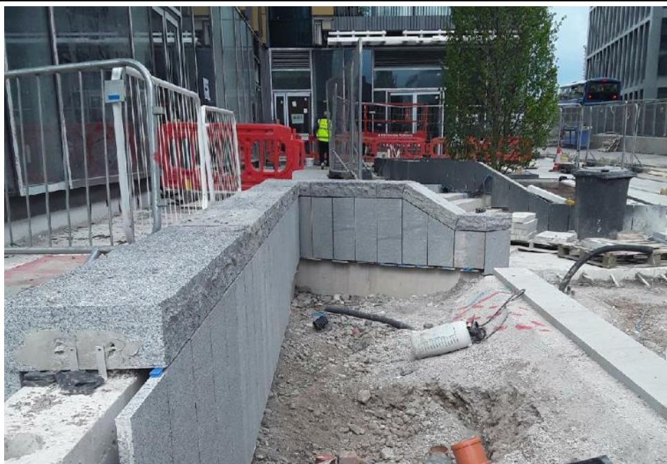
Before topsoil installation
