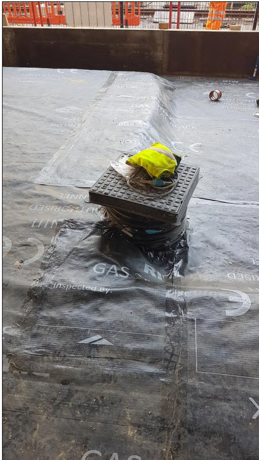
Figure 8: Membrane installation with manhole penetrations
