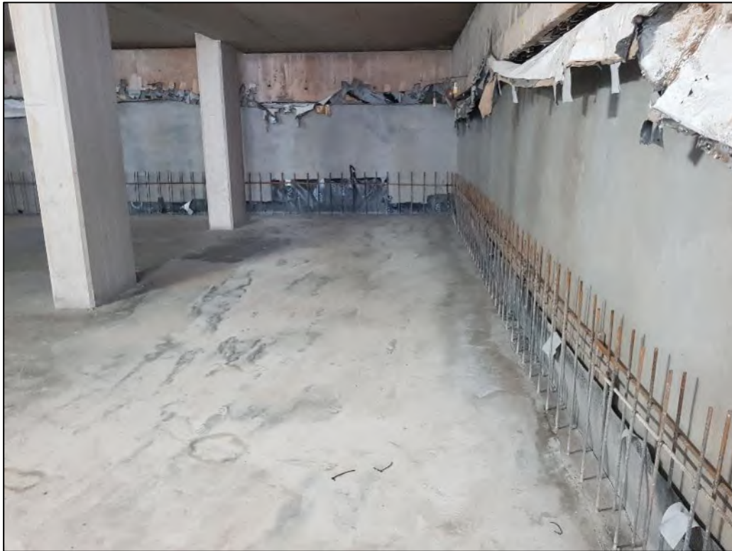
Figure 7: After concrete slab cast
