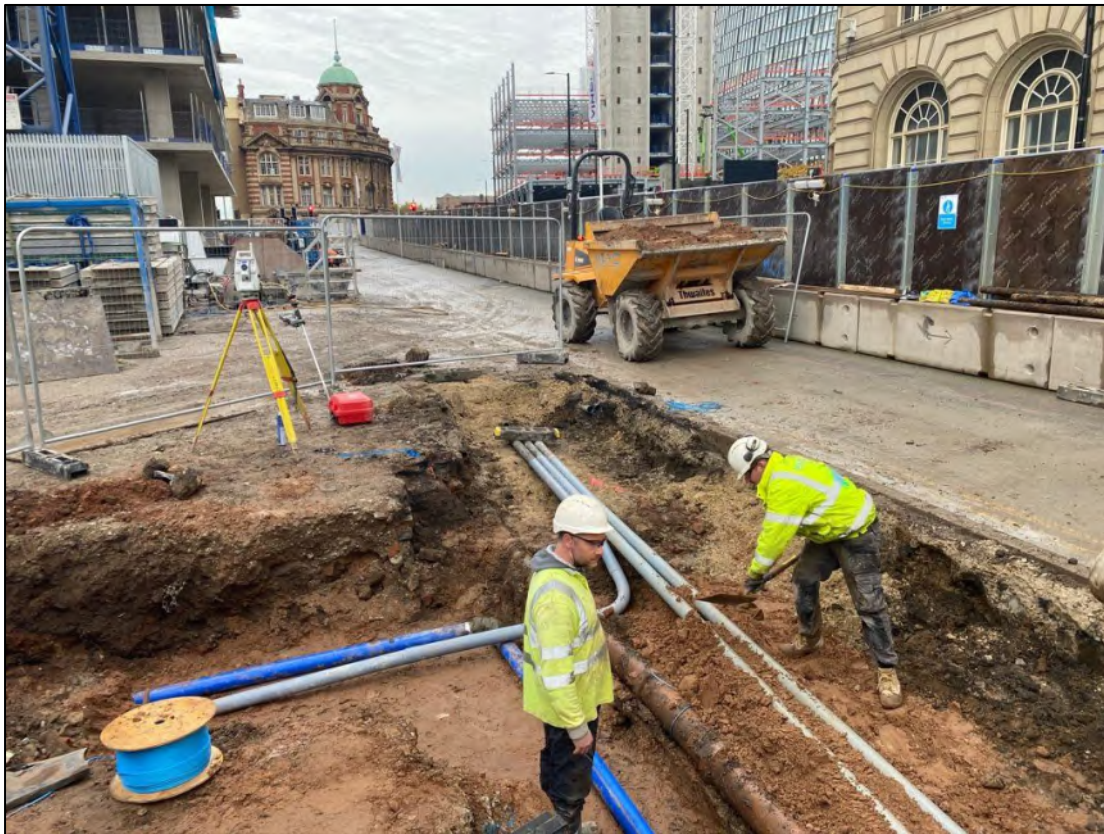
New water pipe installation
