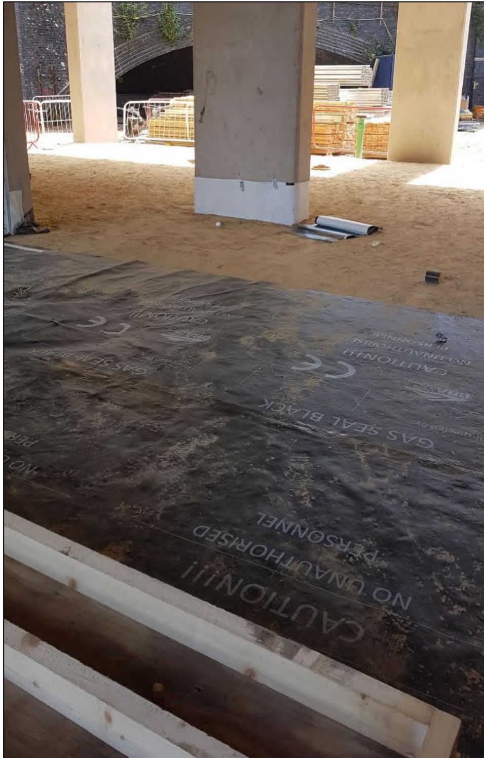
Figure 2: Photo showing the extent of membrane installation at time of visit
