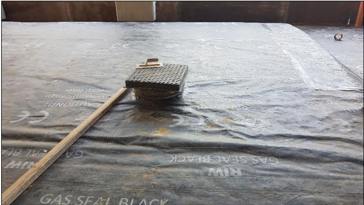
Figure 9: Membrane installation with manhole penetrations
