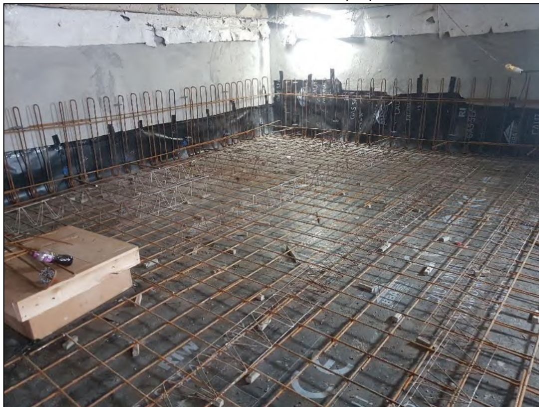
Figure 11: Membrane installed prior to concrete slab casting (SE corner)
