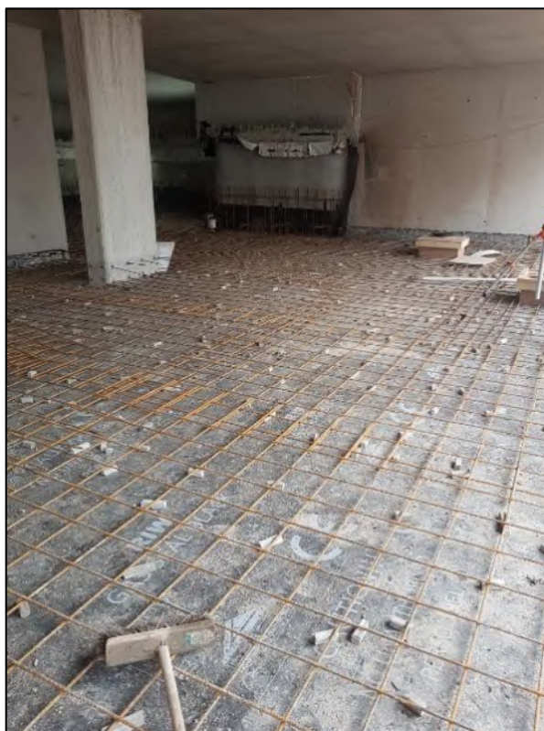
Figure 15: Membrane installed prior to concrete slab casting (looking to SE corner)
