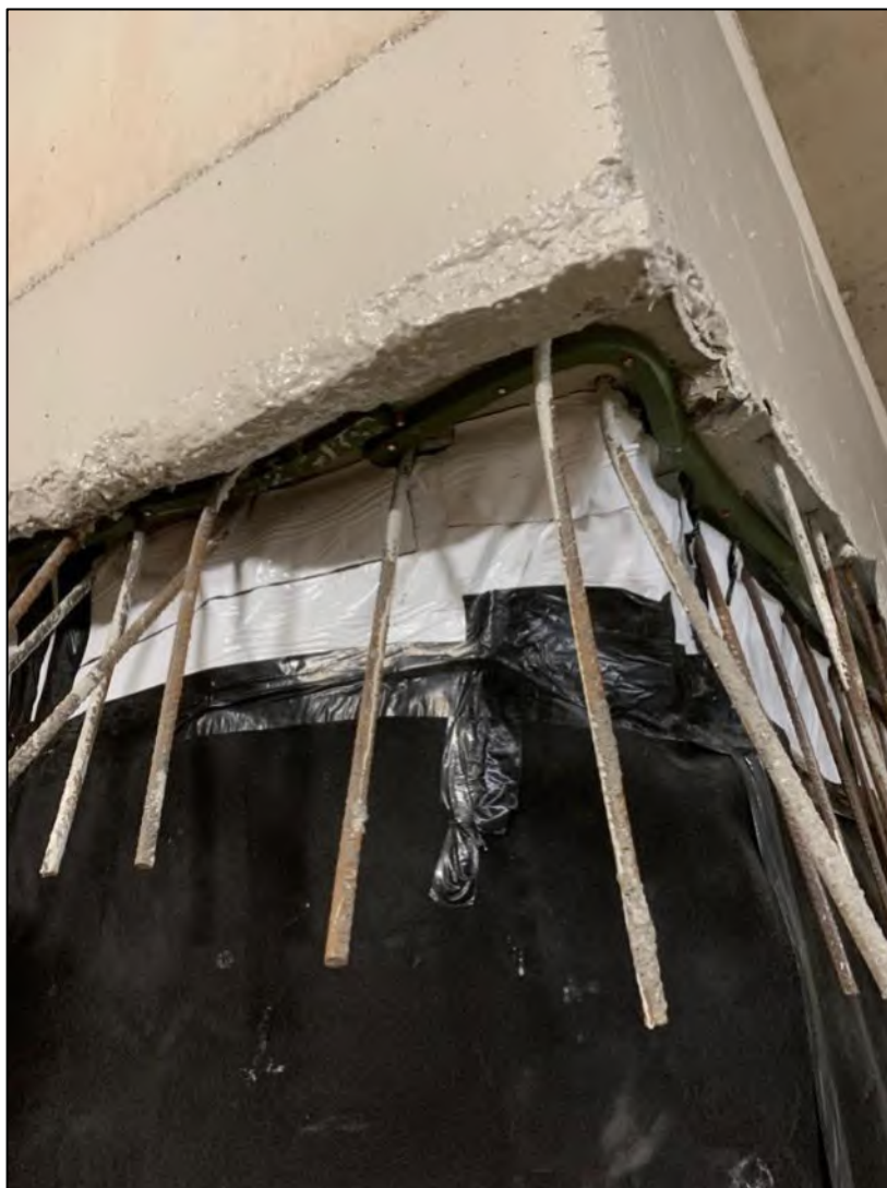
Figure 21: Photo showing the repair (23/11/21). It is understood that the RIW liquid membrane and foil tape has been used to patch the damage. Details of the repair were designed by RIW and drawings will be provided.
