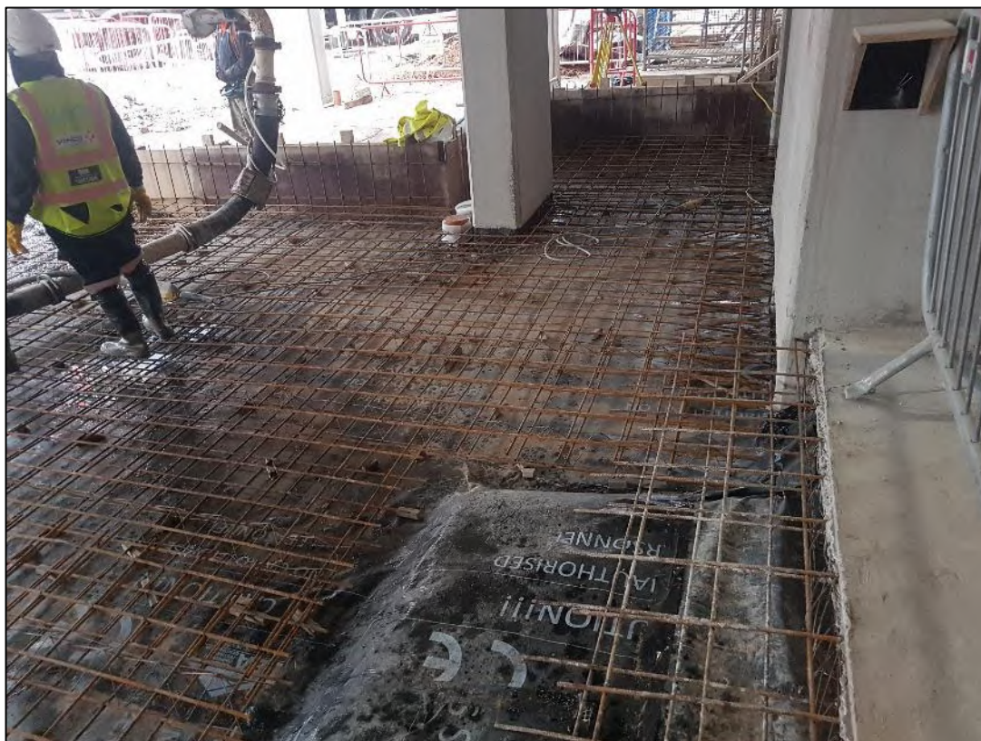
Figure 17: Membrane installed during concrete pour (central west area)
