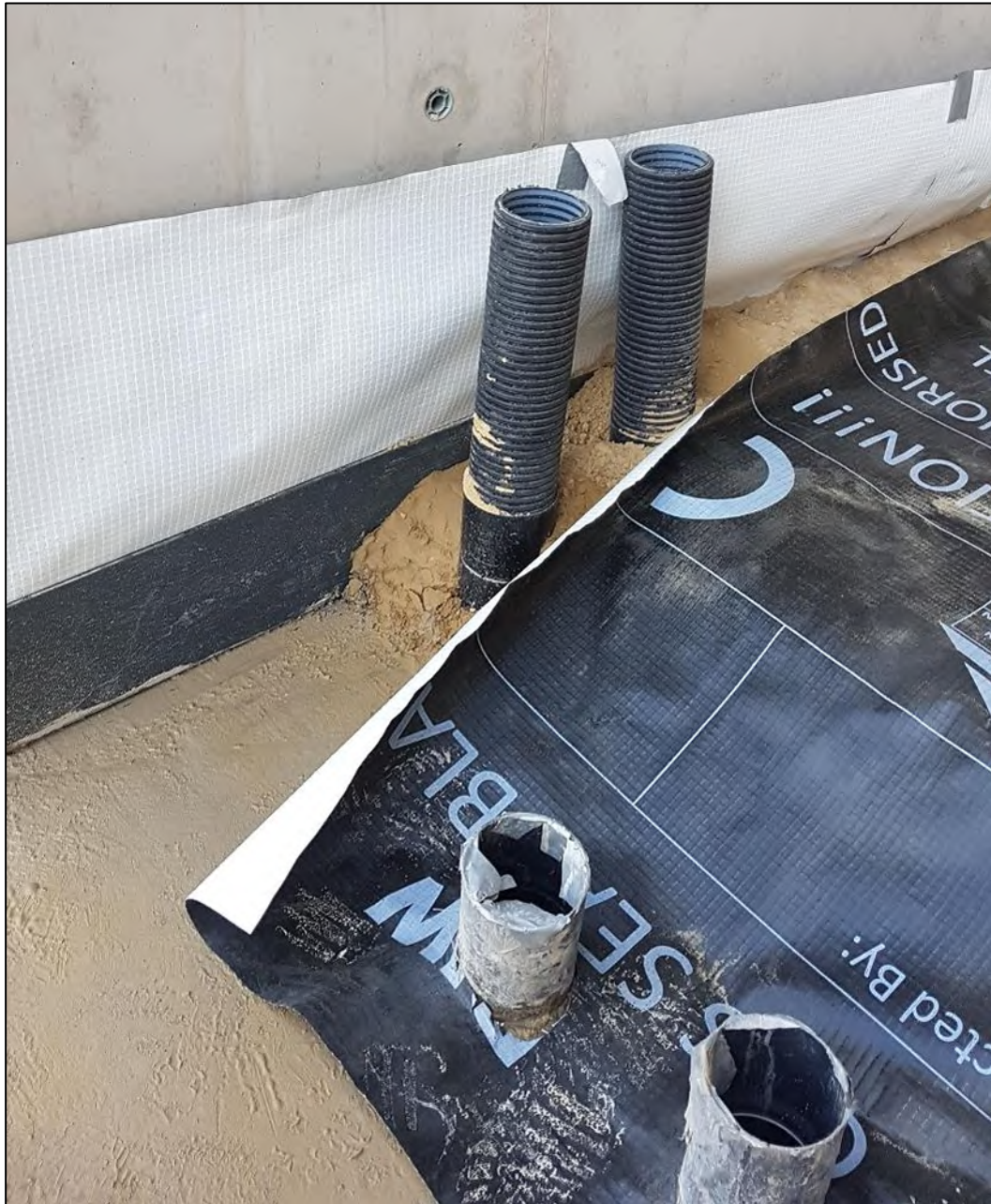
Figure 3: Photo showing sand blinding and service penetrations and overlapping along membrane prior to sealing
