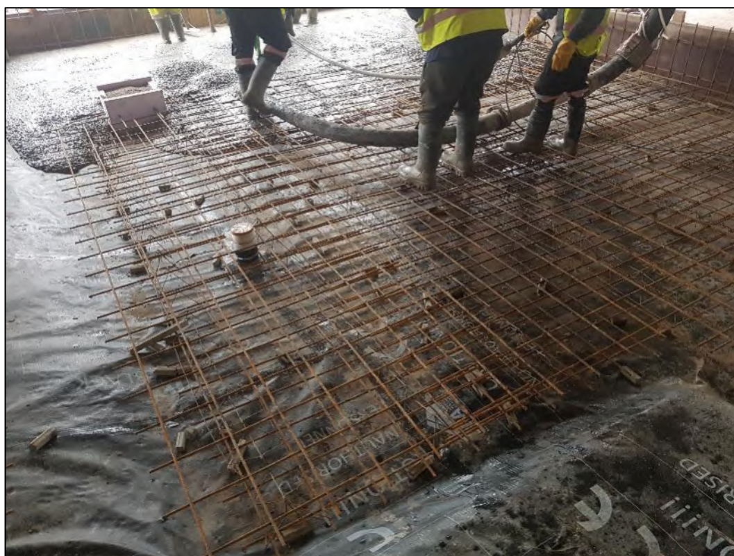
Figure 18: Membrane installed during concrete pour (central west)
