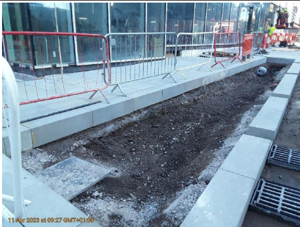
Area 3 before installation of subsoil and topsoil
