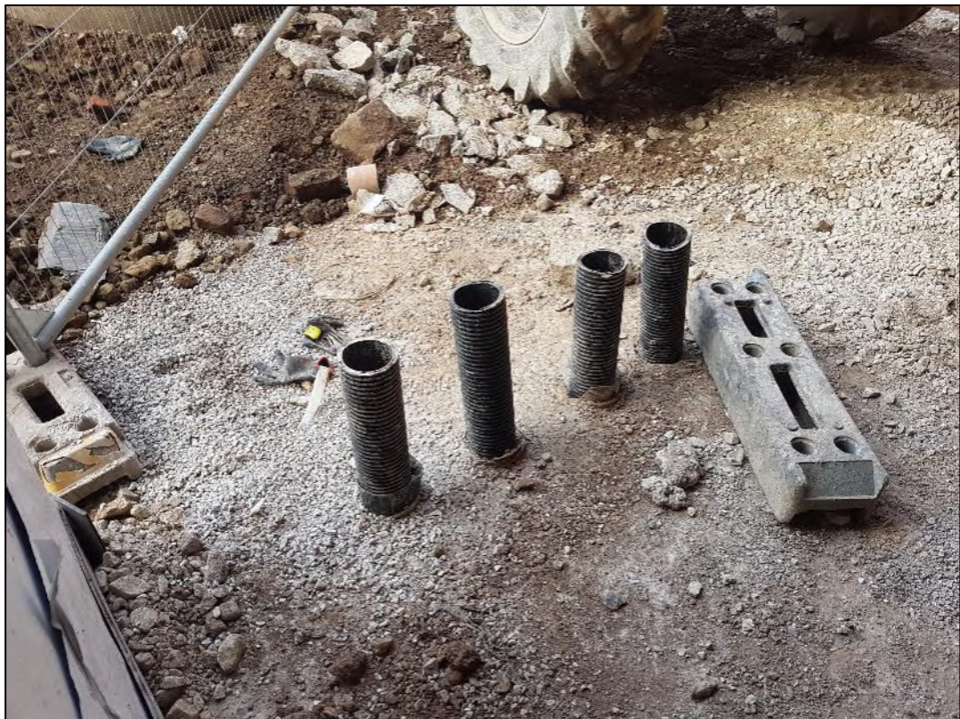
Figure 4: Service ducts prior to installation
