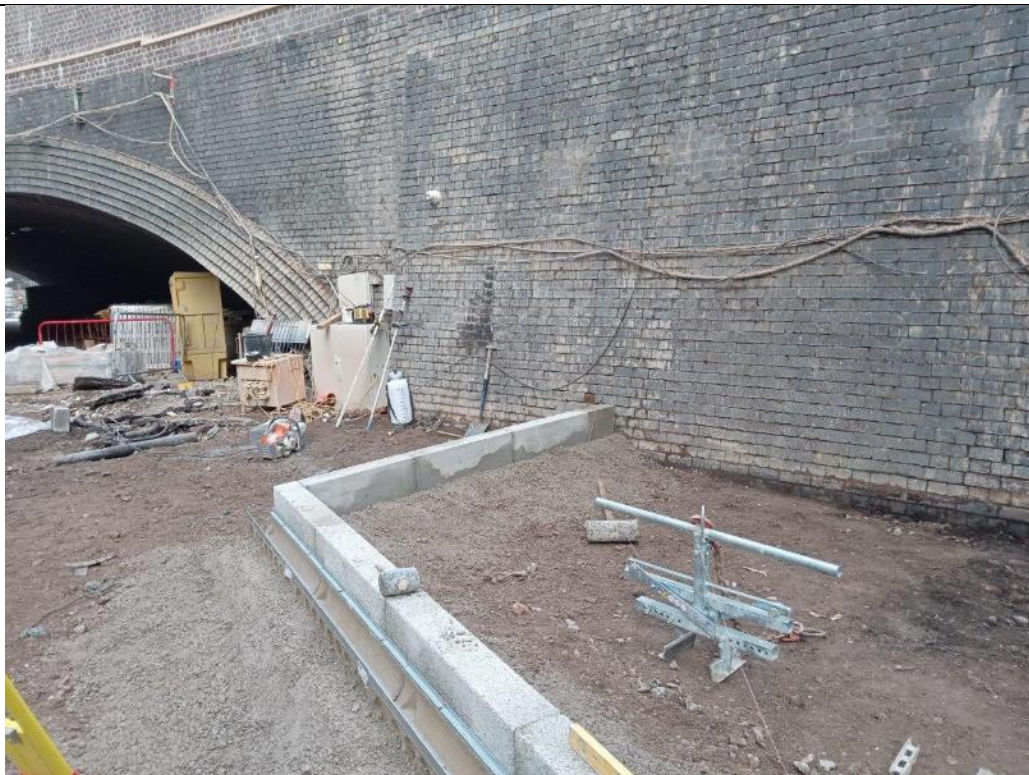
Area 2 before installation of topsoil
