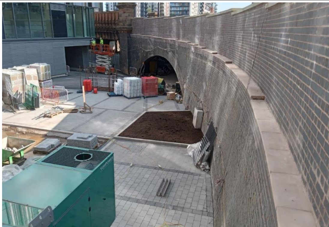
Area 2 after installation of topsoil
