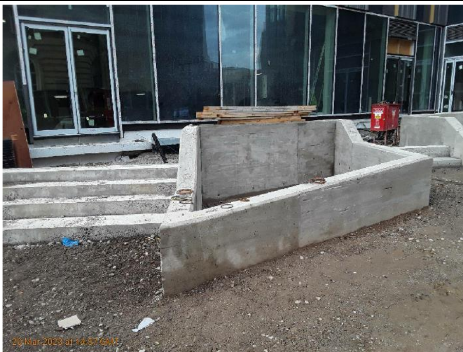
Before topsoil installation
