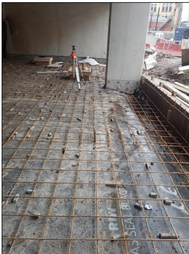
Figure 16: Membrane installed prior to concrete slab casting (South west corner)
