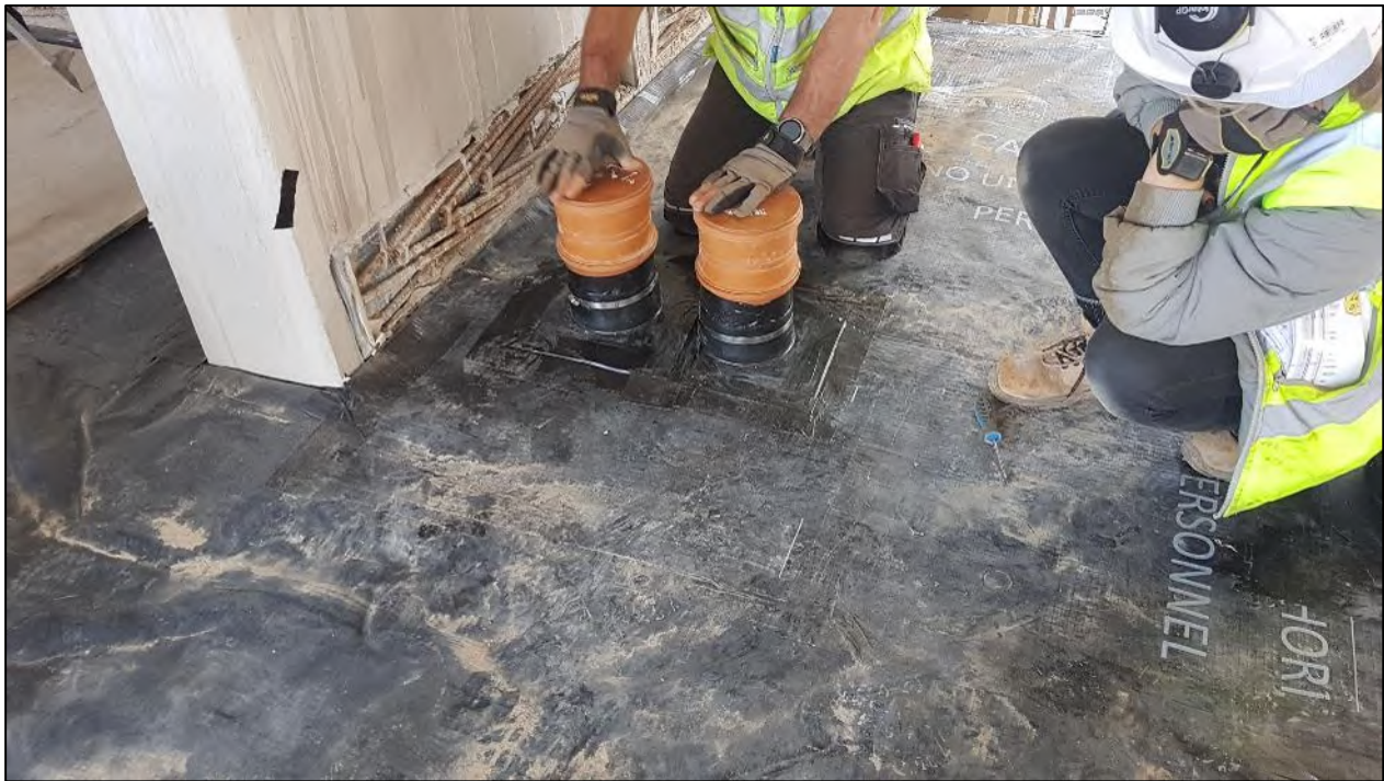
Figure 10: Membrane installation with service penetrations completed
