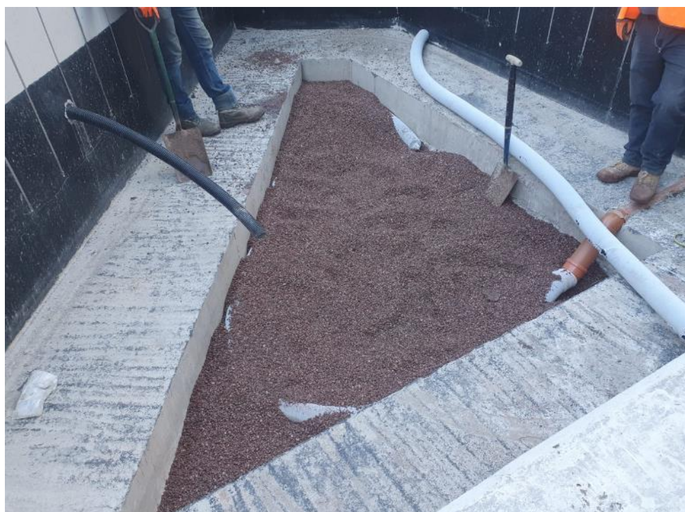
Area 6 before installation of subsoil and topsoil
