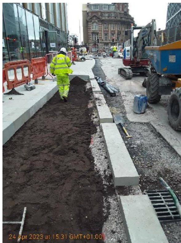
Plot 3 after topsoil installation
