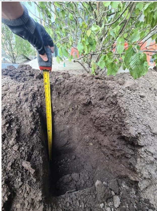
After topsoil installation
