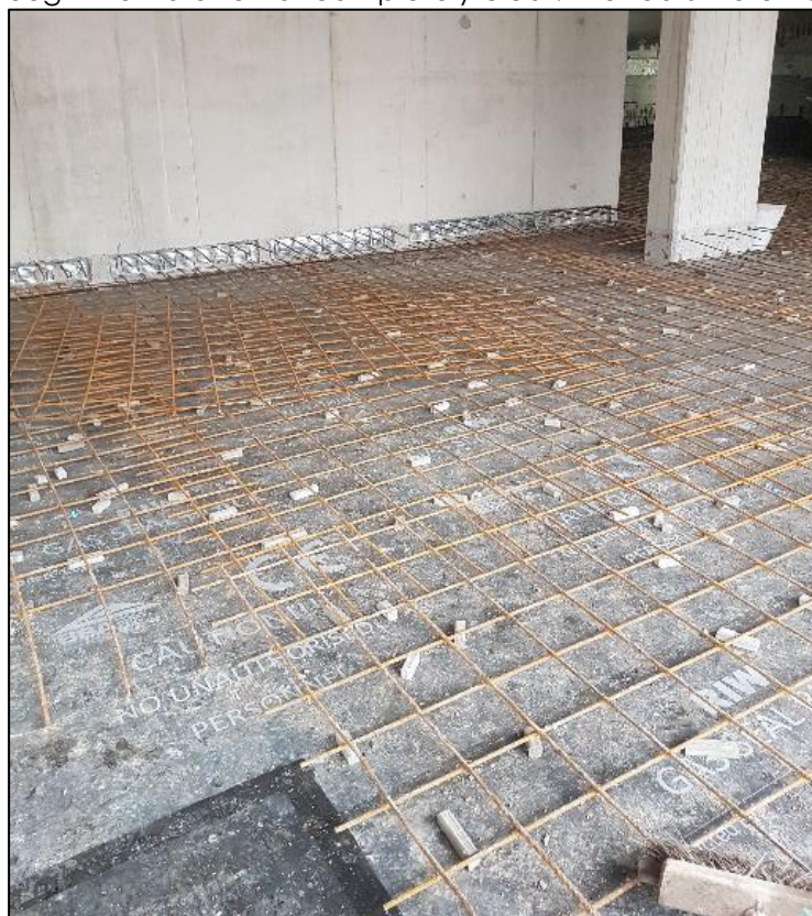
Figure 14: Membrane installed prior to concrete slab casting (central west)
