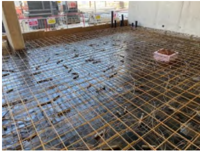
Gas seal black applied under steel reinforcement prior to slab been poured.
