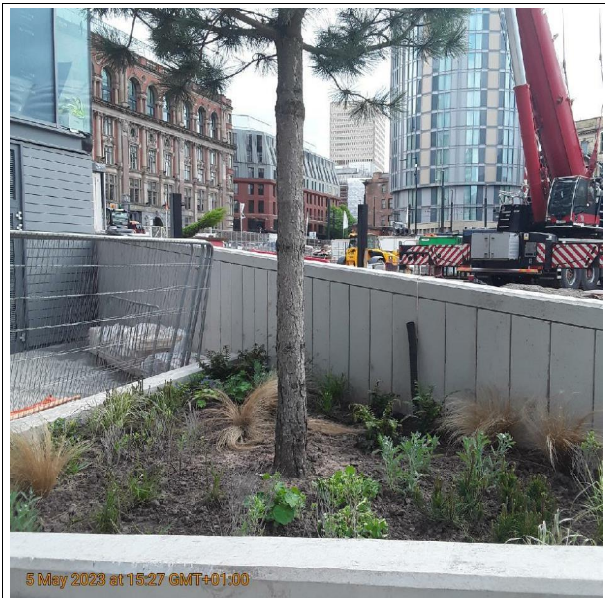
Plot 6 after instation of topsoil and semi-mature tree
