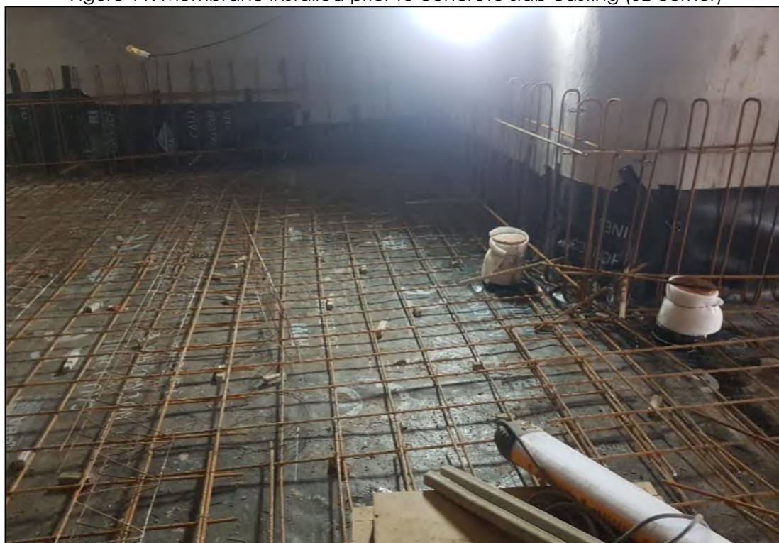
Figure 12: Membrane installed prior to concrete slab casting (SE corner)
