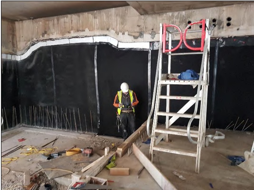
Figure 9: Membrane installation along contig pile wall
