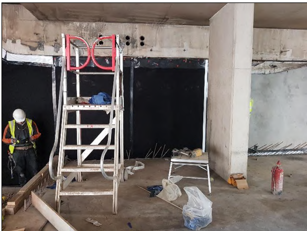
Figure 10: Membrane along contig pile wall
