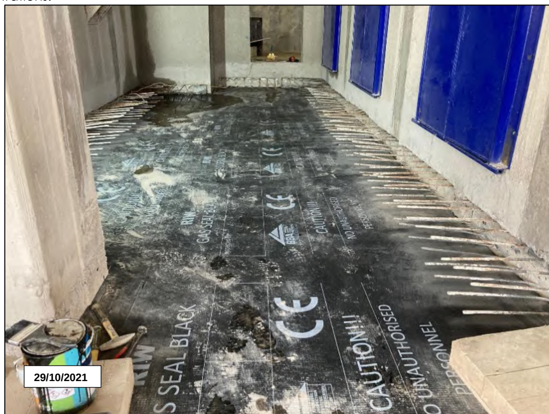
General Photos showing membrane installation and showing detail around columns and pipe penetrations.
