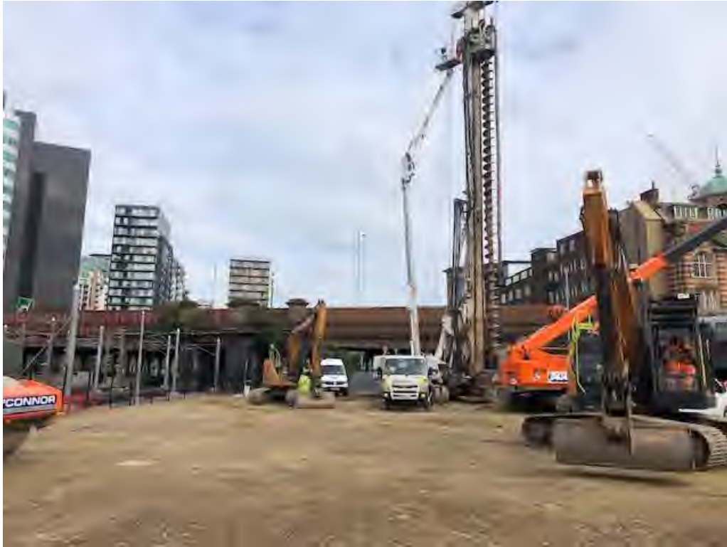
PLATE 7 WORKING PLATFORM CONSTRUCTED WITH MPORTED 6F2
