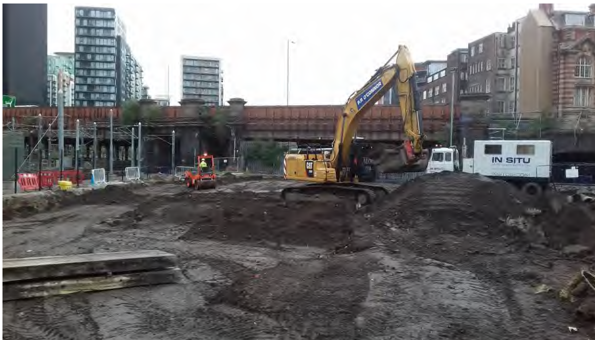
PLATE 4 EXCAVATION, BREAKING OUT AND PROCESSING
