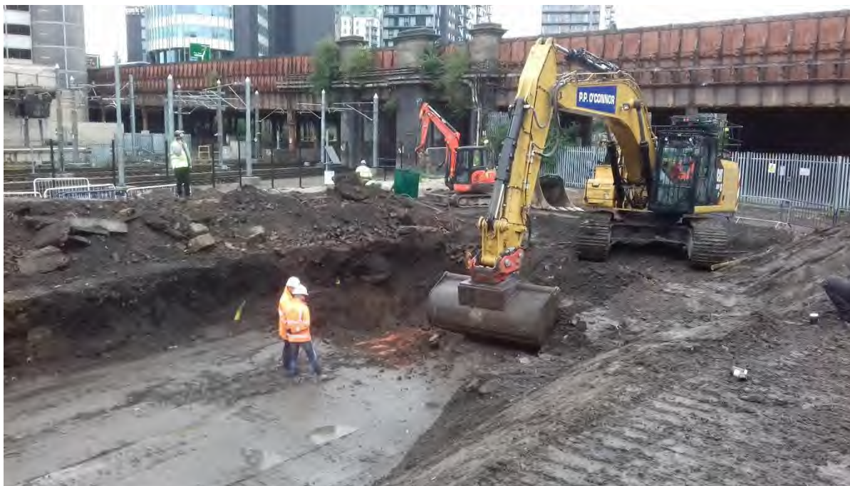
PLATE 2 EXCAVATION, BREAKING OUT AND PROCESSING
