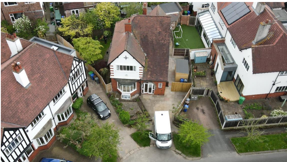
Figure 2: Drone photo of front elevation
