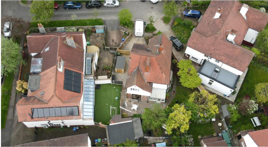
Figure 3: Drone photo of rear elevation
