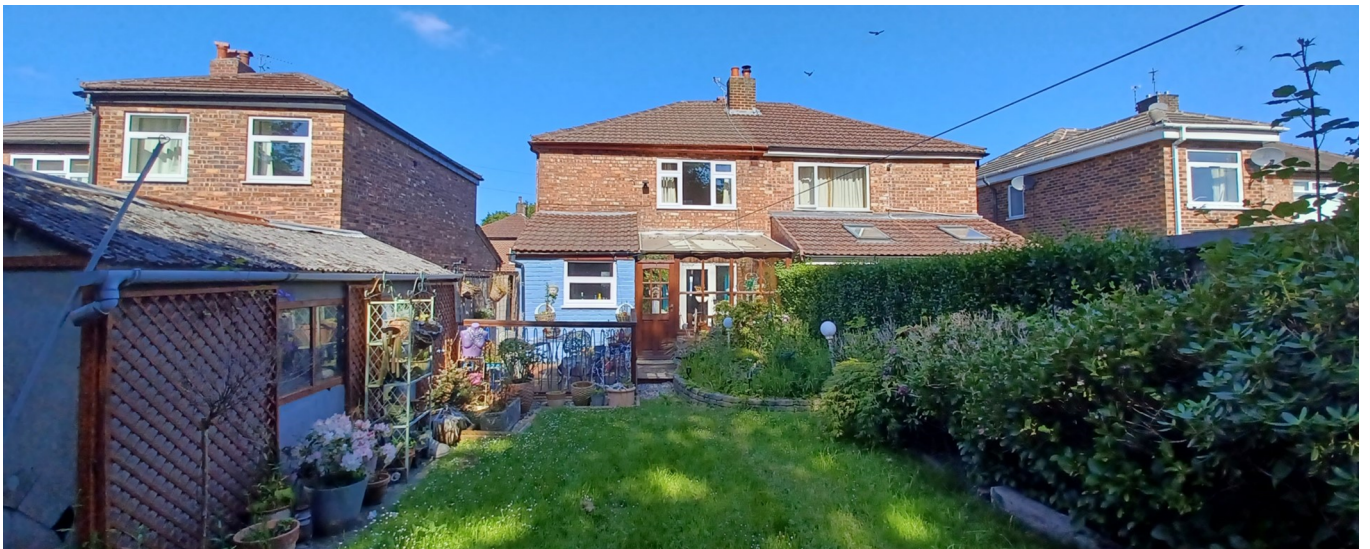
Figure 3. Rear of property.
