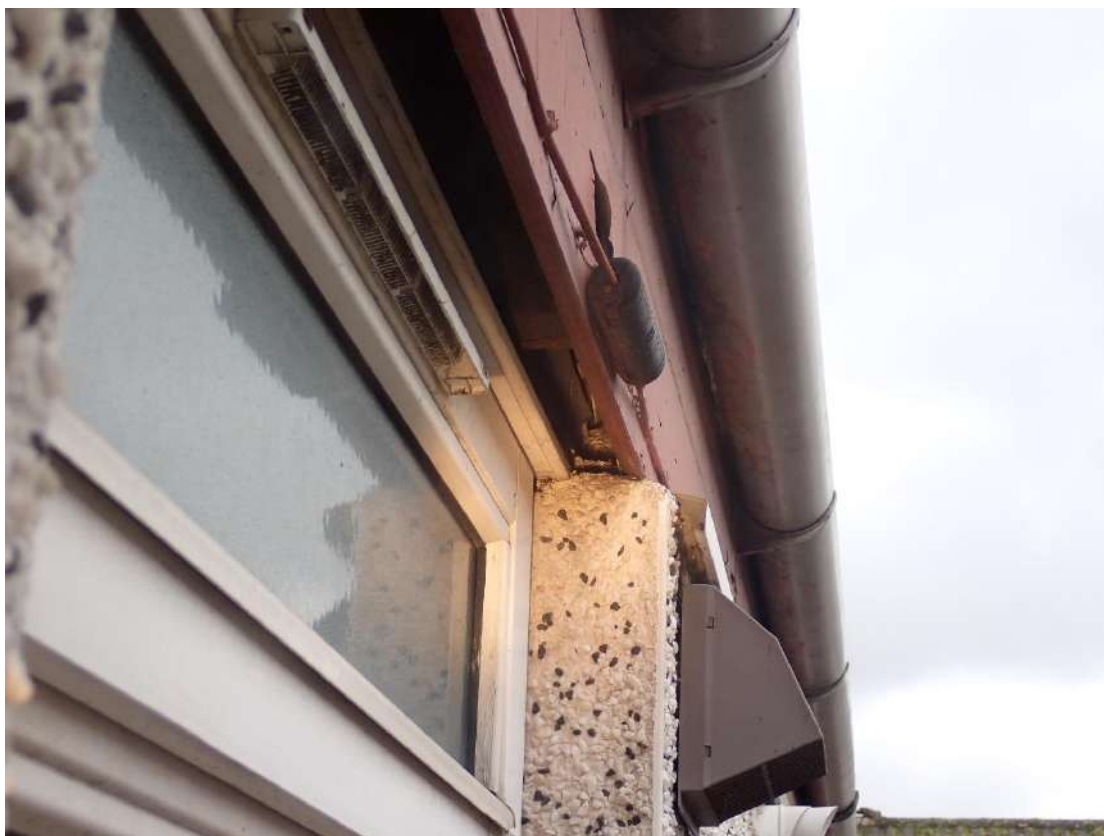
Photograph 7. The bird's nest and gap under the barge board on the eastern aspect of Flat 13.
