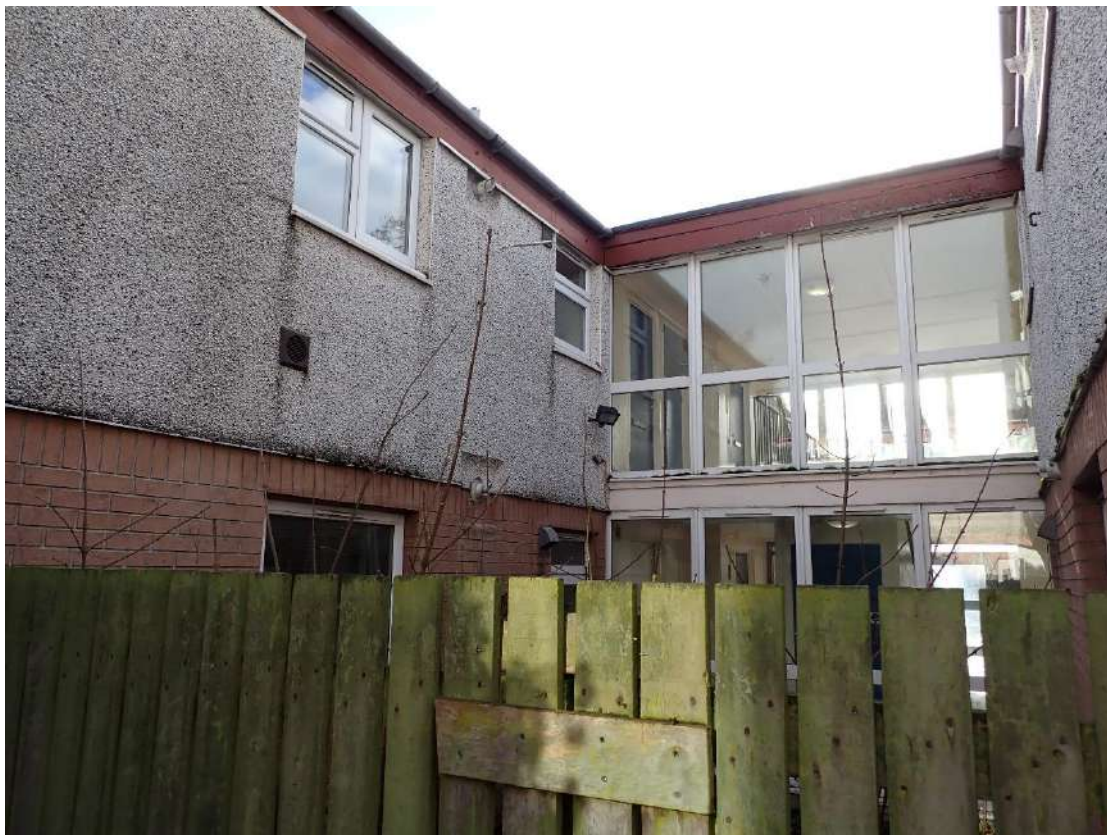
Photograph 2. The northern aspect of the central corridor.
