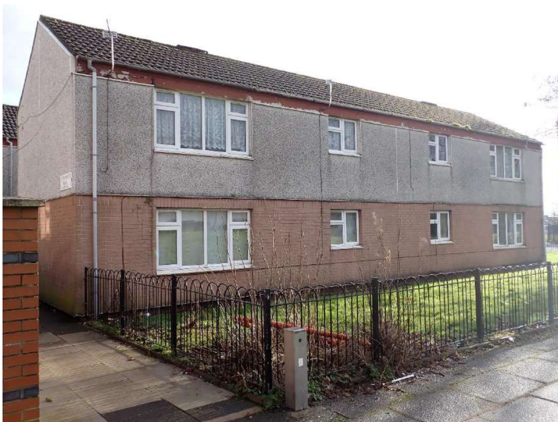
Photograph 3. The western aspect of the building.
