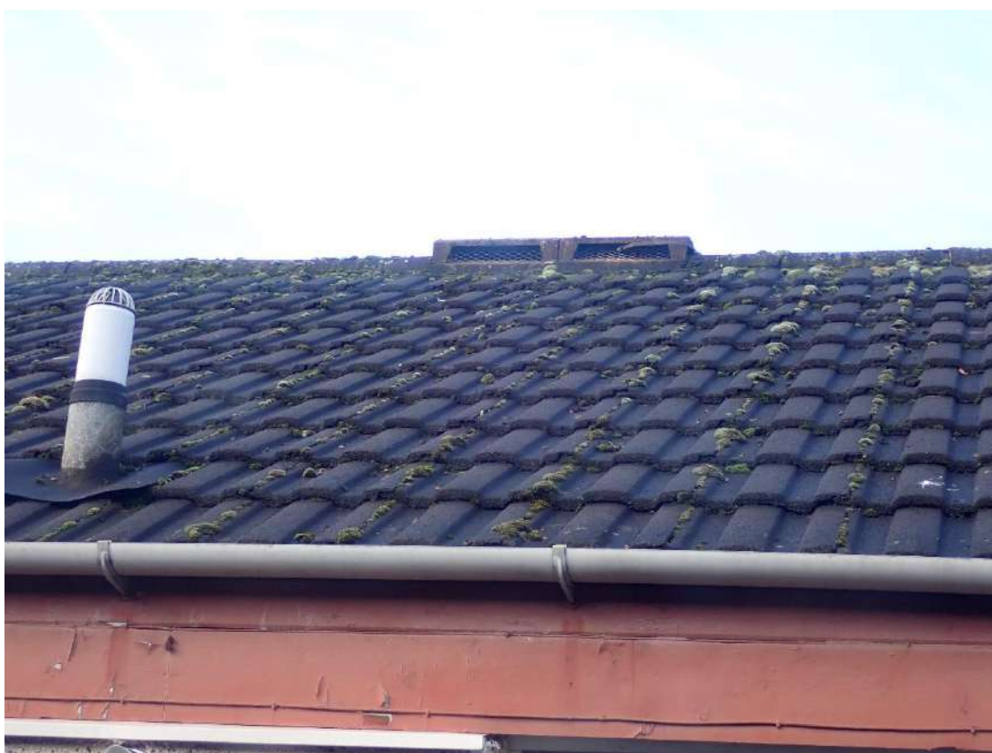
Photograph 4. The grills covering the ventilation shaft above Flat 13.
