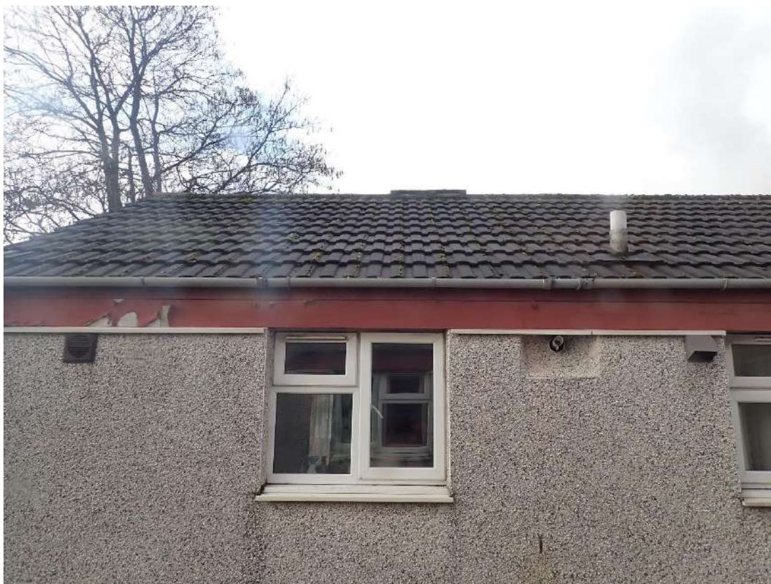
Photograph 5. The cover over the ventilation shaft above Flat 15, the eastern aspect of the building.
