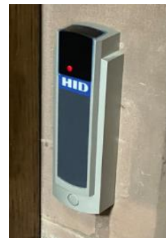
Typical proximity Card reader
