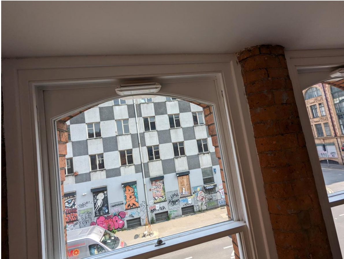
Figure A.2: First-floor Living Room Glazing and Ventilators
