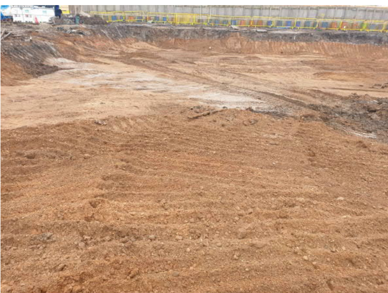
Photograph 14. Site-preparation, cut levels
