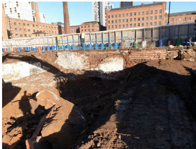
Photograph 8. Former basement area to the east
