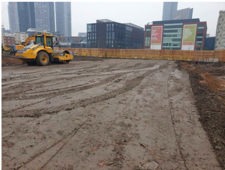
Photograph 15. Surface preparation for piling mat
