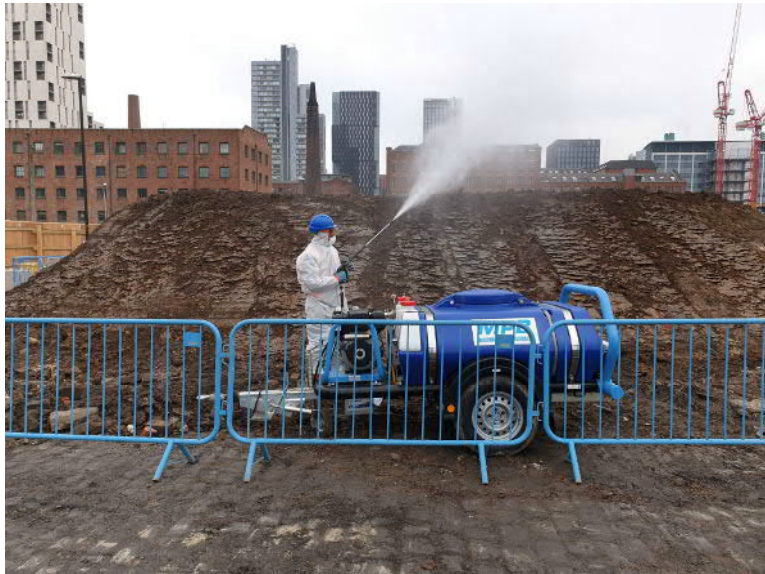
Photograph 9. Dust-suppression measures to dampen stockpiles
