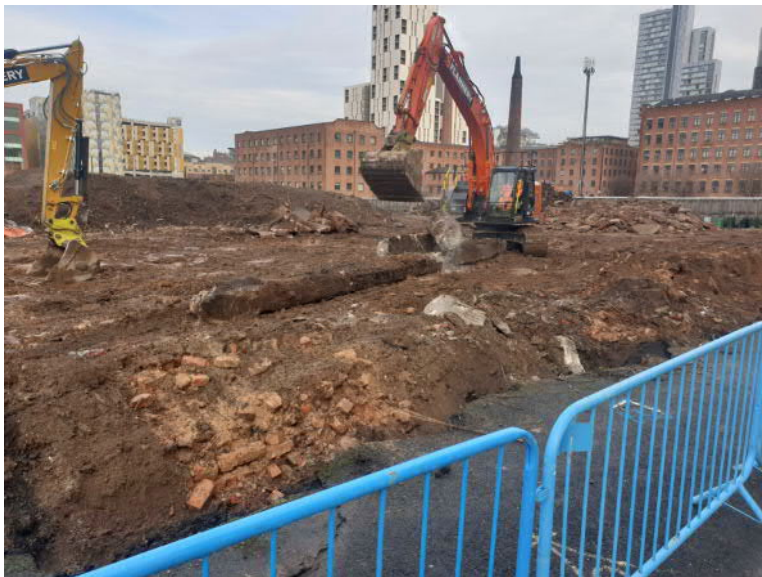
Photograph 3. Site Preparation Works
