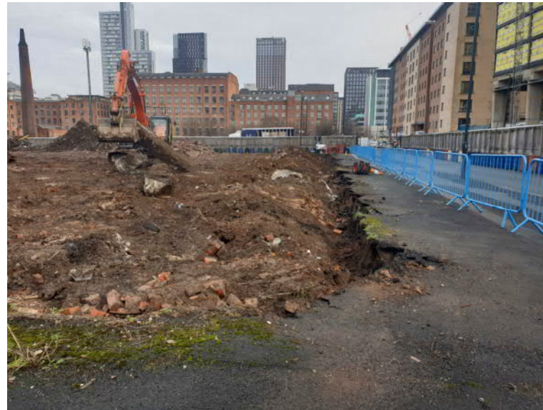
Photograph 2. Site Preparation Works
