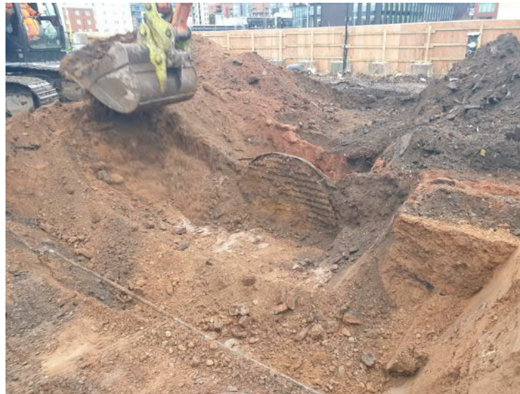
Photograph 6. Remnants of former air-raid shelter
