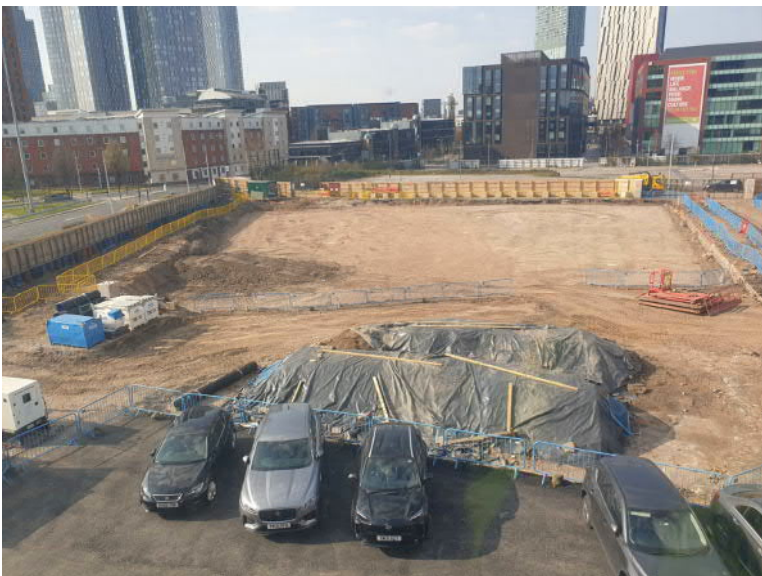
Photograph 12. Sheeted stockpile prior to off-site disposal
