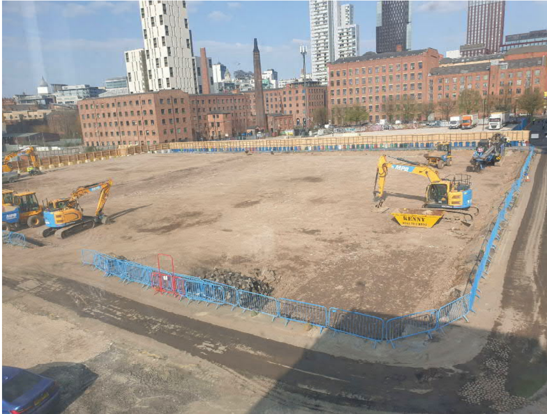
Photograph 13. Site overview - completed site works
