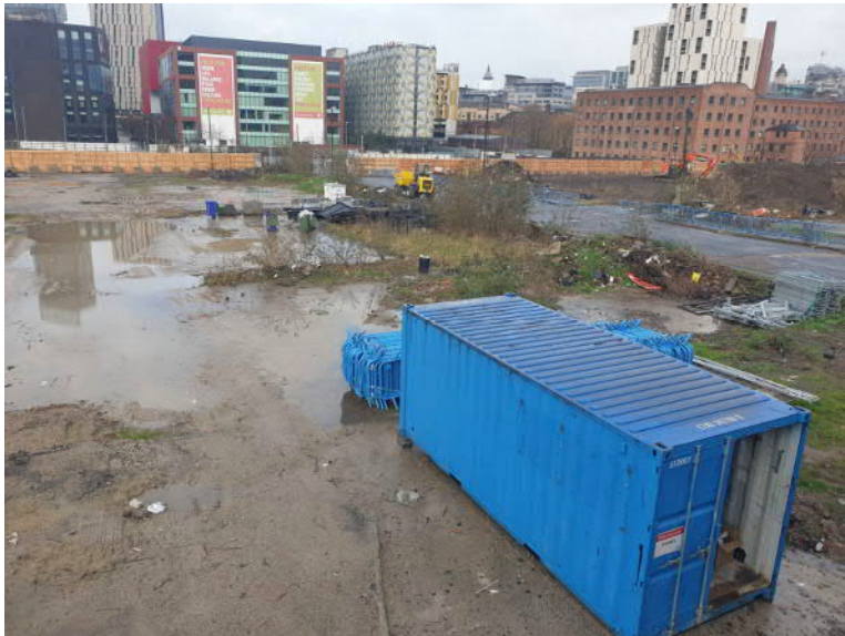
Photograph 1. Site overview – pre site works
