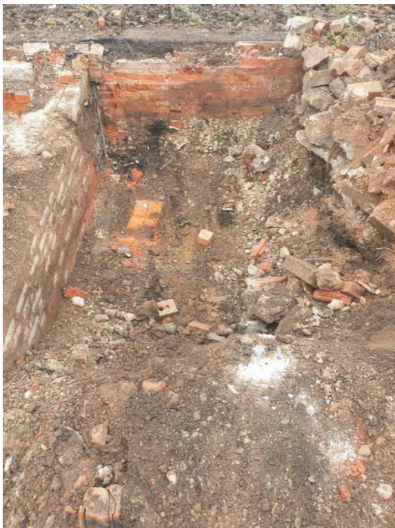
Photograph 7. Former basement area to the east
