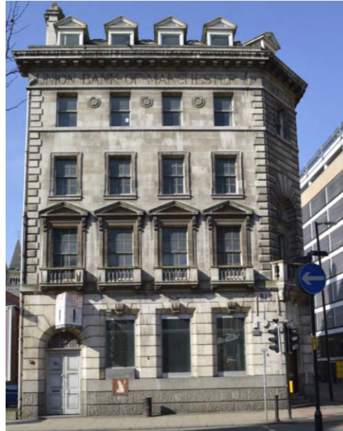
Piccadilly elevation with historically significant listed façade.
