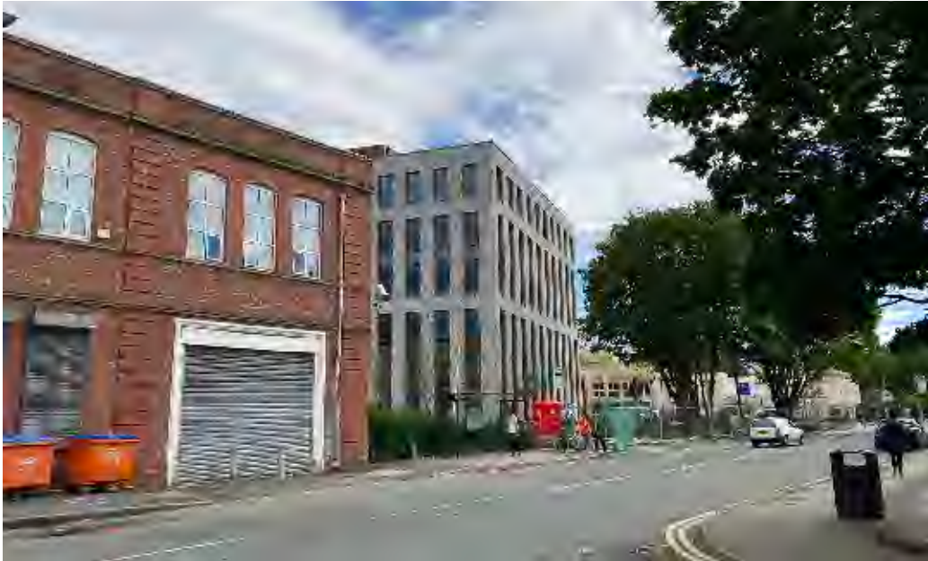
4 - View from Greenheys Lane - BASE Building
