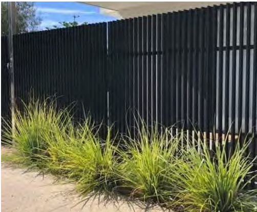
Vertical flat bar Railing, 2400mm high, security fence for service yard, visually softened by a double height hedge
