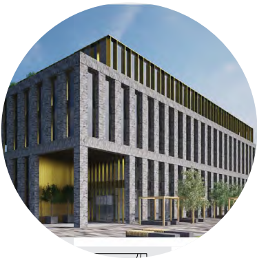
Adjacent BASE Building
