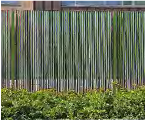
Vertical slatted louvred Railing, 2400mm high, green colour, for liquid nitrogen tank store
