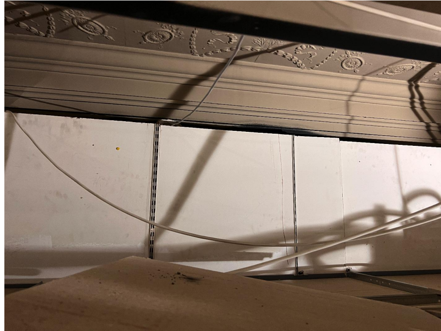
PHOTOGRAPH SHOWING EXISTING PLASTER CORNICE
