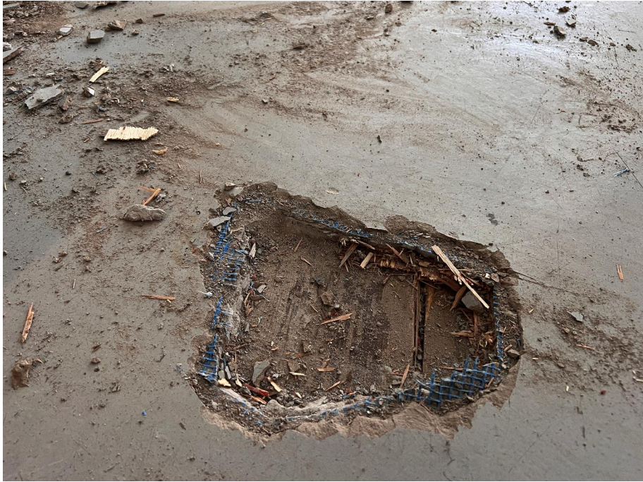
EXISTING RETAIL UNIT FLOOR FINISH - POURED RESIN OVER SCRIM MESH REINFORCEMENT, LAID OVER LEVELLING SCREED, OVER PLY SUBSTRATE FIXED TO ORIGINAL SOFTWOOD TIMBER FLOORBOARDS
