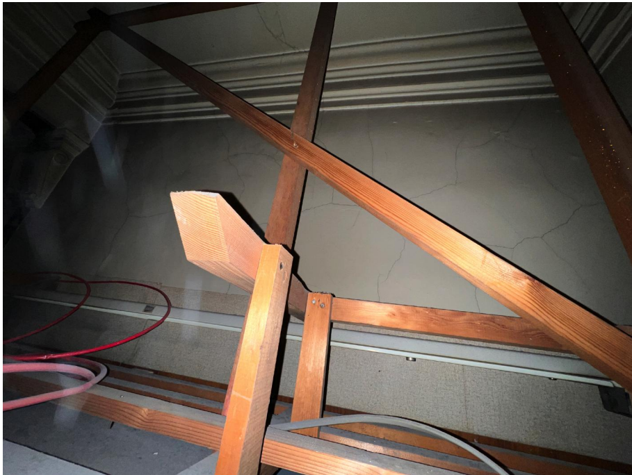
PHOTOGRAPH SHOWING EXISTING MASONRY WALL AND PLASTER CORNICE
