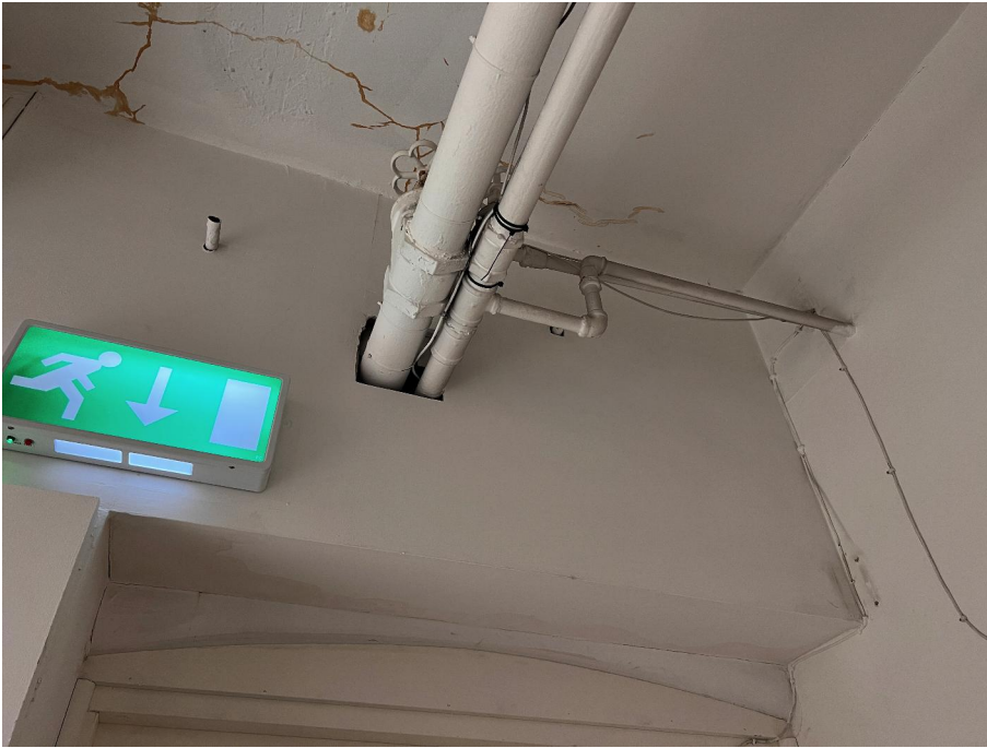
EXISTING PIPED SERVICES AND CABLES PASSING THROUGH EXISTING PENETRATIONS IN MASONRY WALL
