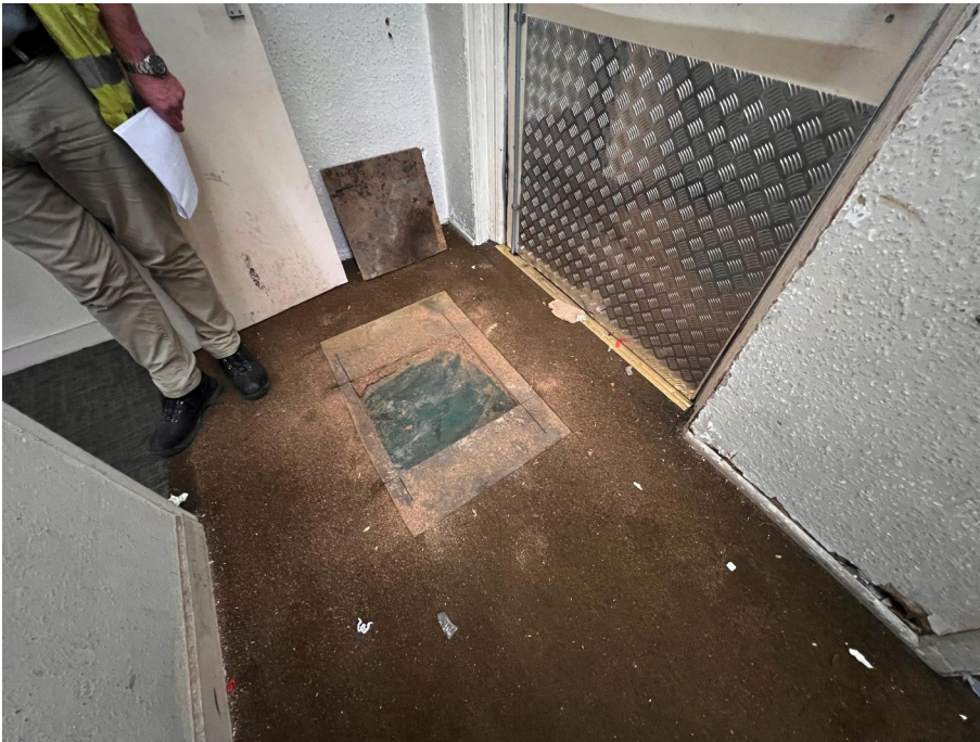
PHOTOGRAPH SHOWING AREA OF EXISTING FLOORING AND BOARDED BUILD-UP REMOVED TO REVEAL SUBFLOOR
