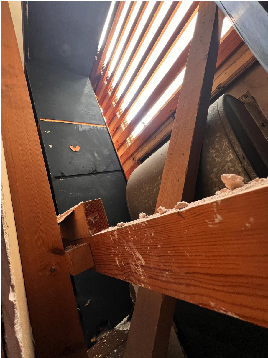
PHOTOGRAPH SHOWING EXISTING VENTILATION DUCTS RISING IN VOID SPACE AND FORMING CONNECTION WITH EXTERNAL GRILLE
