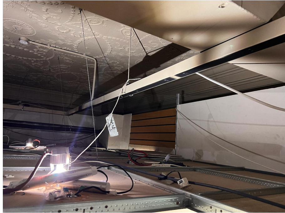
PHOTOGRAPH SHOWING SPACE ABOVE EXISTING LAY IN GRID SUSPENDED CEILING AND EXISTING WALL LININGS PROJECTING ABOVE
