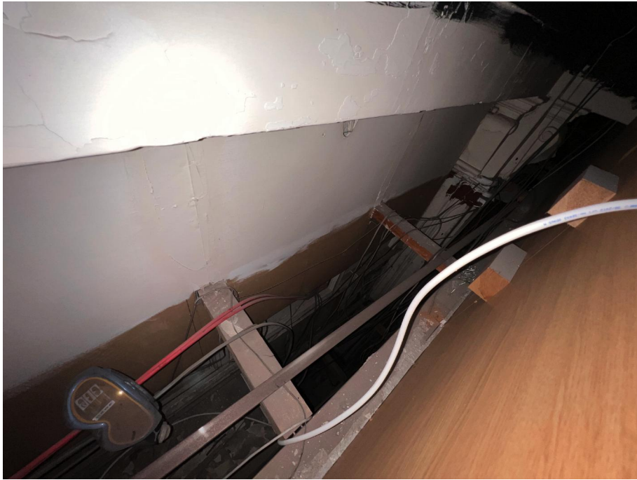
PHOTOGRAPH SHOWING EXISTING MASONRY WALL AND MASONRY BEAM BELOW CORNICE
