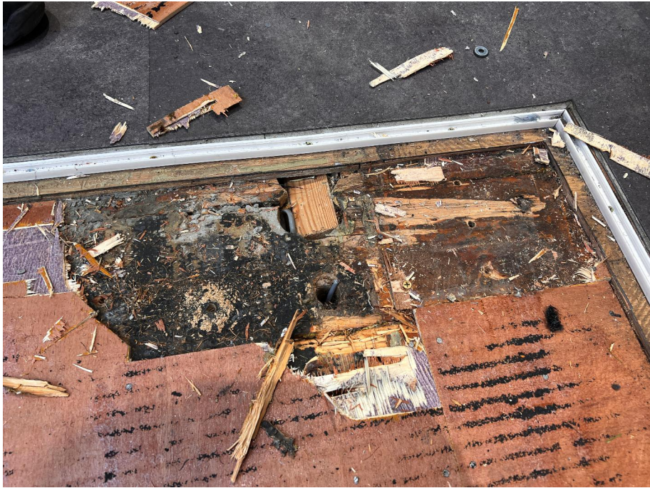
EXISTING ENTRANCE AREA FLOOR BUILD-UP - BARRIER MATTING OVER LAYERS OF PLYWOOD FORMING SUBSTRATE FIXED TO ORIGINAL SOFTWOOD TIMBER FLOORBOARDS
