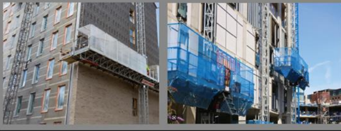
Typical mast climber protection netting to protect against material falling onto waterway
