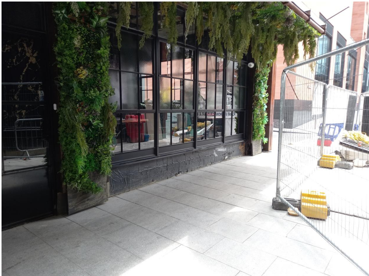
New pavings along the Avenue North
