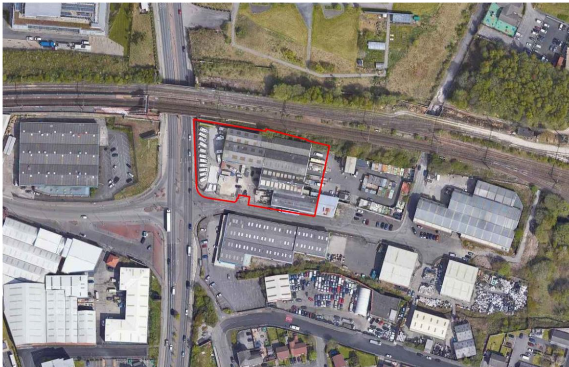
Fig. 01 Aerial Site Location Photograph
