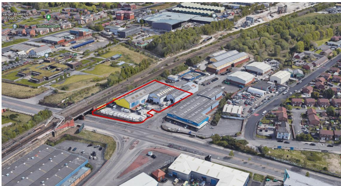
Fig. 03 Aerial Site Photograph
