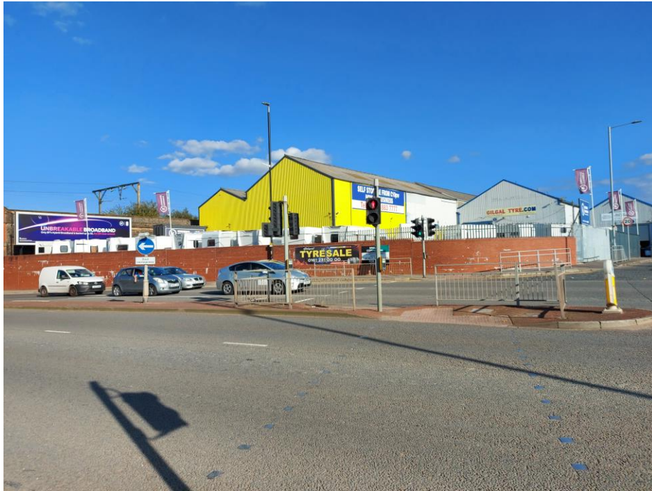
Fig. 05 Photograph from the Gorton Lane junction looking east to the site
