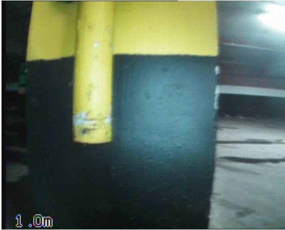
RWD7 (F3)X_d82e9535-0fad-4b1d-bd78-f495b189e8ed_20230911_085416_170.jpg, 00:00:00, 0.00 m Start node, major connection without manhole, reference: RWDP7 (F3)
