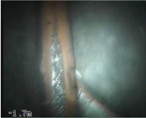
MH9X_34789c8c-97bd-430f-9579-10f4cfc413de_20230911_084558_940.jpg, 00:00:00, 0.00 m Start node, manhole, reference: MH9
