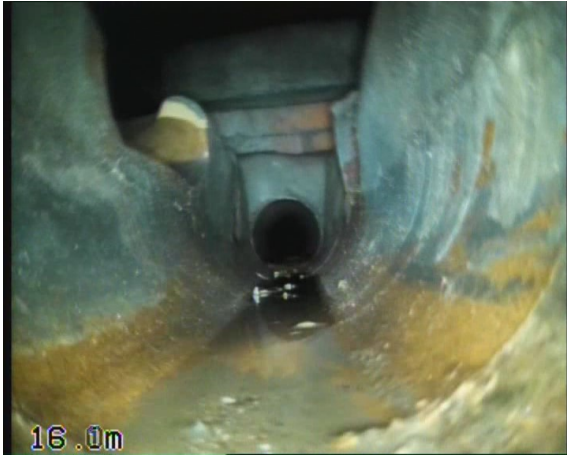
MH2X_b1c7efed-4948-4f80-81f8-34ccf8402d40_20230908_1 10716_266.jpg, 00:01:06, 16.00 m Finish node, manhole, reference: MH2
