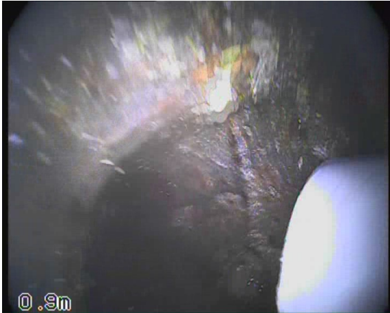
RWDP6 (L1)X_bc38c55f-aa92-4e3a-ba6f-69f6bb645067_20230908_1 02352_431.jpg, 00:00:00, 0.00 m Start node, major connection without manhole, reference: RWDP6 (F1)
