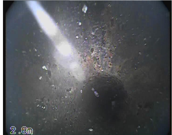
RWDP6 (L1)X_e3690cff-ba78-4c8d-b1fe-cddd9bf8a740_20230908_10 2442_700.jpg, 00:00:34, 0.00 m General photograph taken at this point
