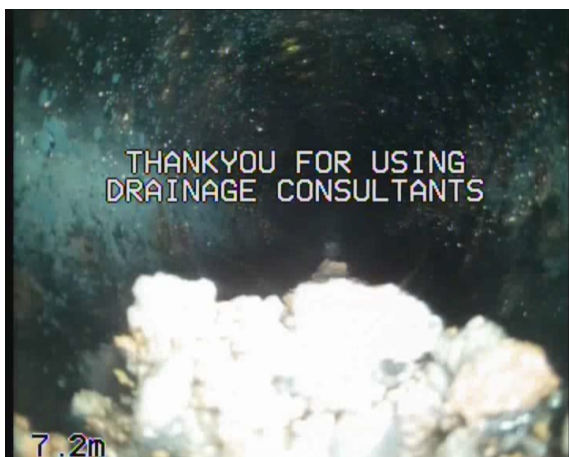
HOLX_c1eb0fe9-052f-4f62-b33a-dcf2a21ca54e_20230908_104016_325.jpg, 00:00:34, 7.20 m Survey abandoned, Unable to pass stones/rocks
