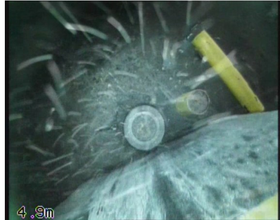
RWDP1 (F1)X_0fb32242-f7db-4981-ad34-1d9cf0192b31_20230911_090842_456.jpg, 00:00:29, 4.90 m Finish node, major connection without manhole, reference: Discharge, (Floor-3)
