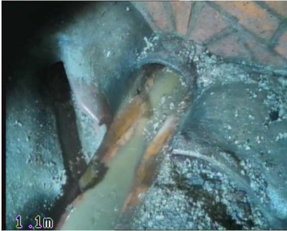
MH5X_a83e40f5-09d1-4353-960f-f334f38e4df2_20230911_082225_893.jpg, 00:00:00, 0.00 m Start node, manhole, reference: MH6
