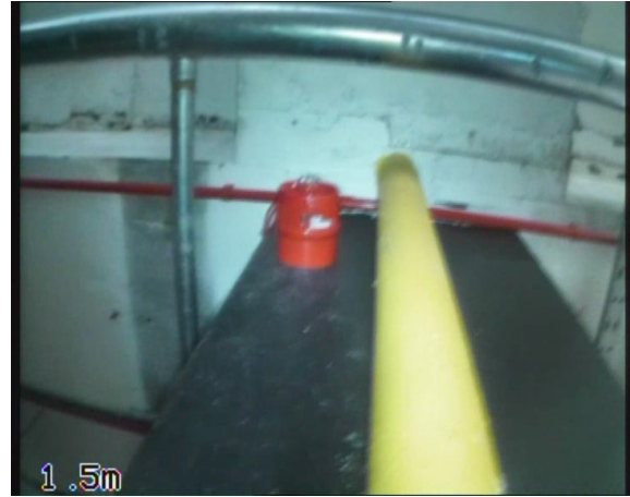
HOLX_70a65193-43e0-47e6-9d45-4201420a63f1_20230911_085500_314.jpg, 00:00:00, 0.00 m Start node, major connection without manhole, reference: RWDP7 (F3)
