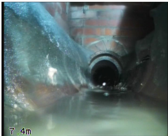
MH8X_cb36dcc5-5a76-4fbc-97af-5f6b69628376_20230911_084007_387.jpg, 00:00:35, 7.50 m Finish node, manhole, reference: MH9
