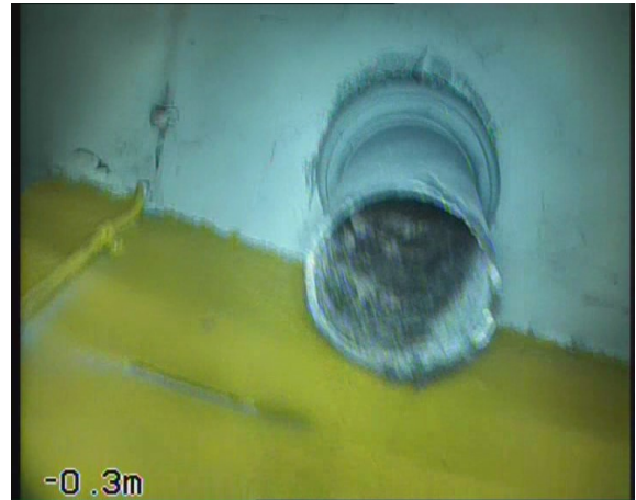
HOLX_9e8fd359-af53-491b-af22-db7decb8ccaf_20230911_092207_567.jpg, 00:00:00, 0.00 m Start node, major connection without manhole, reference: RWDP2 (F1)
