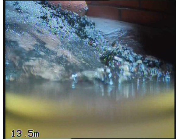
MH9X_3832b18c-5303-4e09-b496-48c025d230f1_20230911_084833_530.jpg, 00:01:09, 13.50 m Finish node, manhole, reference: MH10
