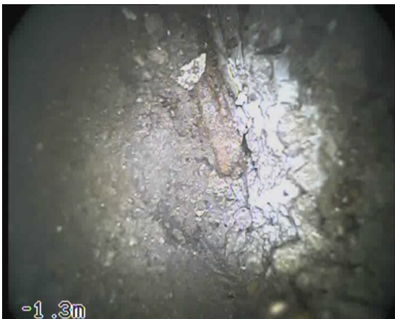
RWDP5 (L1)X_e966202c-af31-431e-998c-c26020799a07_20230908_101750_530.jpg, 00:00:12, 0.00 m Settled deposits, fine, 100% cross-sectional area loss
