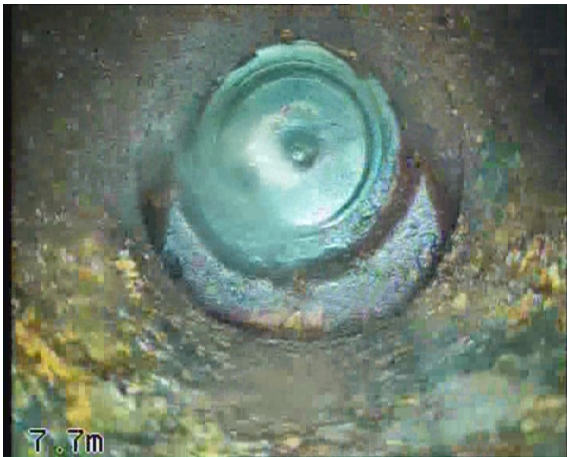
RWDP-7X_c633b9e4-4f45-4081-8d6a-77aa8a96dea0_20230911_081644_639.jpg, 00:01:02, 7.70 m Finish node, gully, reference: RWDP-7
