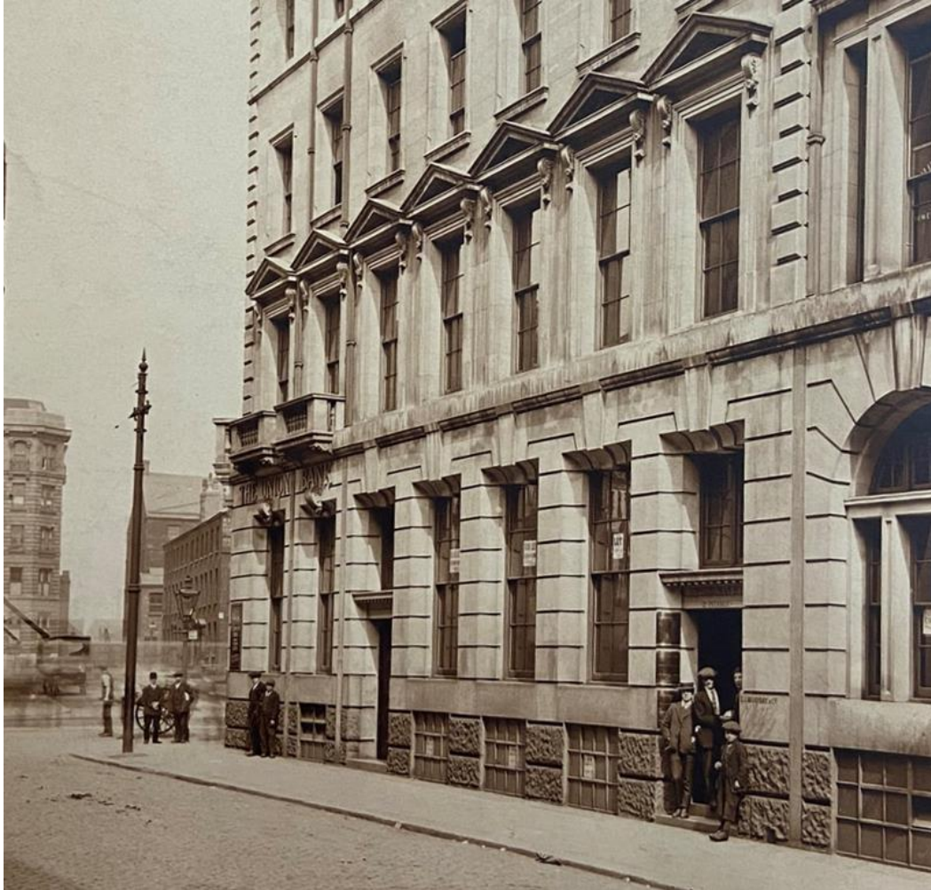
Early 20 th Century photograph of the Chatham Street elevation. Note the two entrances shown on this elevation have subsequently been lost and truncated to form windows matching the others at this level. The four-over-three glazed windows at basement level have also since been removed and infilled with blockwork to match the plinth
