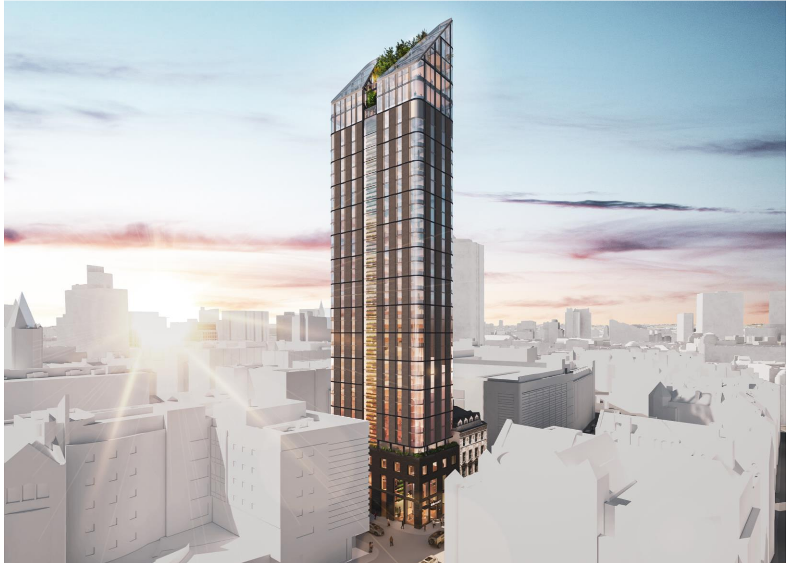
Aerial perspective view from the east capturing the full height of the building in context, with views of Manchester City Centre beyond.
