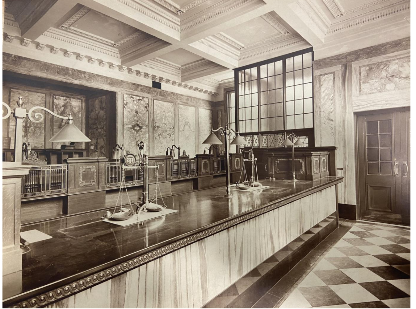
Early 20 th Century photograph of the banking chamber at ground floor level. Very little of this interior survives with the exception of deteriorated areas of moulded coffered plaster ceiling.
