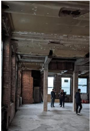
Recent interior views of the Banking Hall, showing condition following soft strip out works
