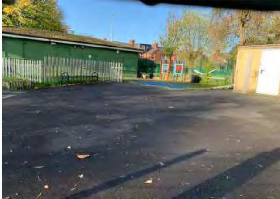
Disused park building and outdoor space
