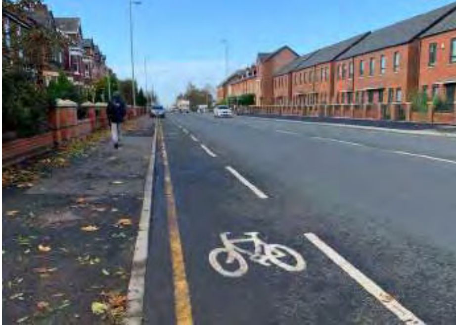
Looking west along Ashton Old Road
