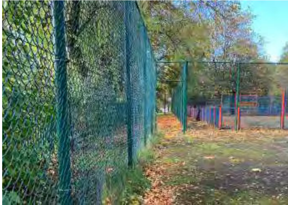
Looking south down the side of the MUGA
