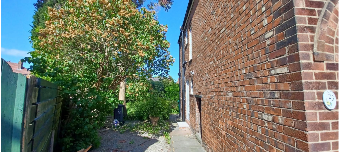
Figure 2. View along the side of property.
