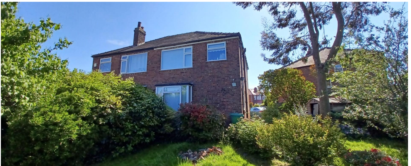
Figure 4. Rear view of property.
