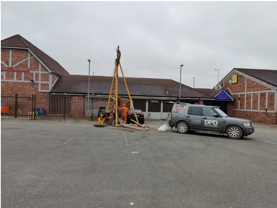
Figure 3 View Facing South Showing the Cable Percussive Borehole Rig Setup
