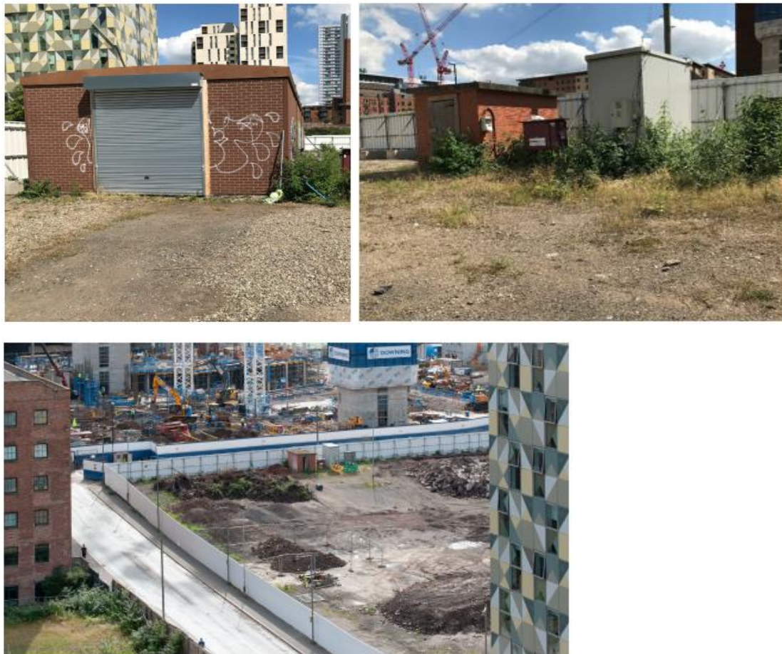
Figure 5.5 Images of the existing structures on the existing site.
