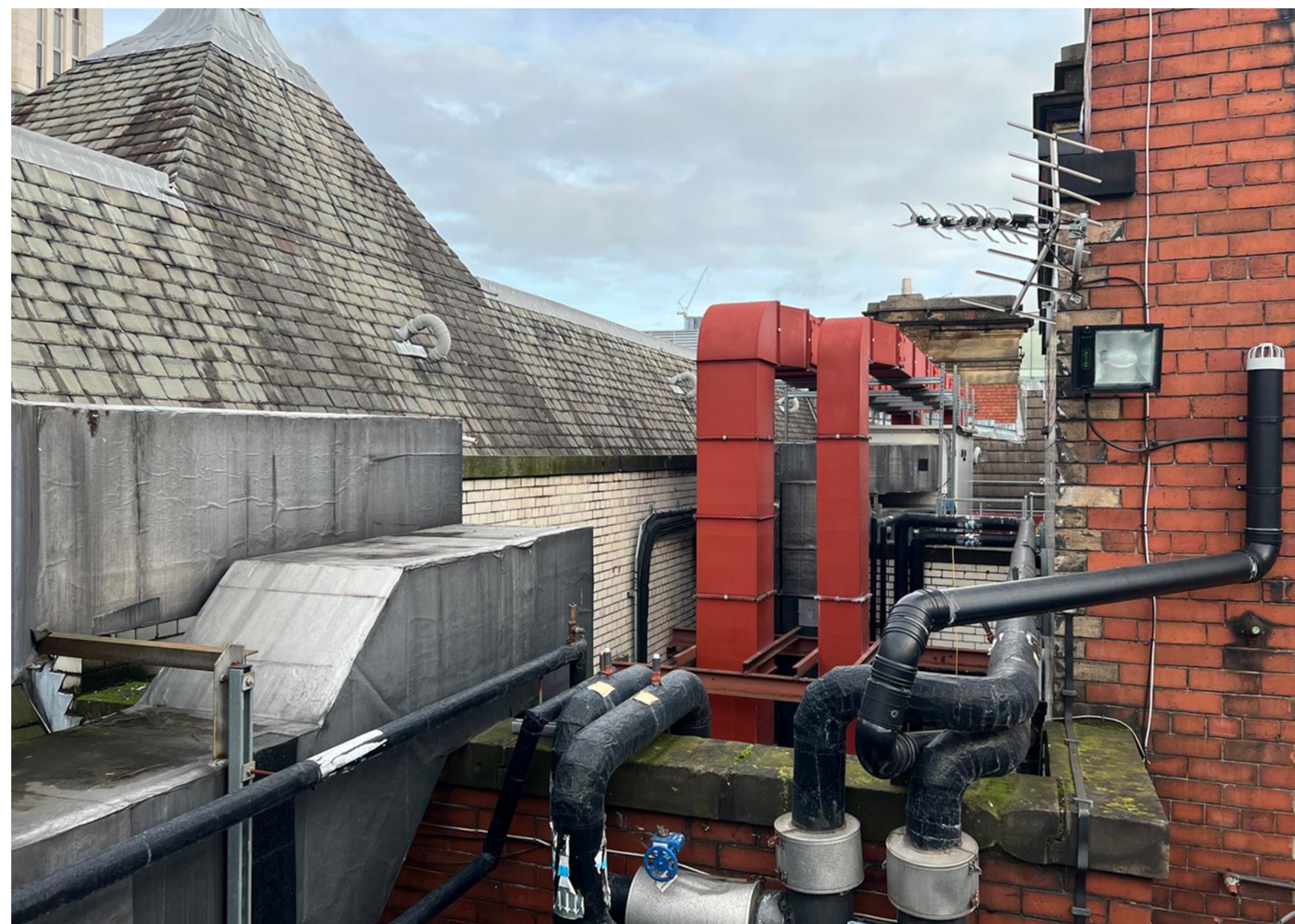
Roof Existing View Photograph 003
