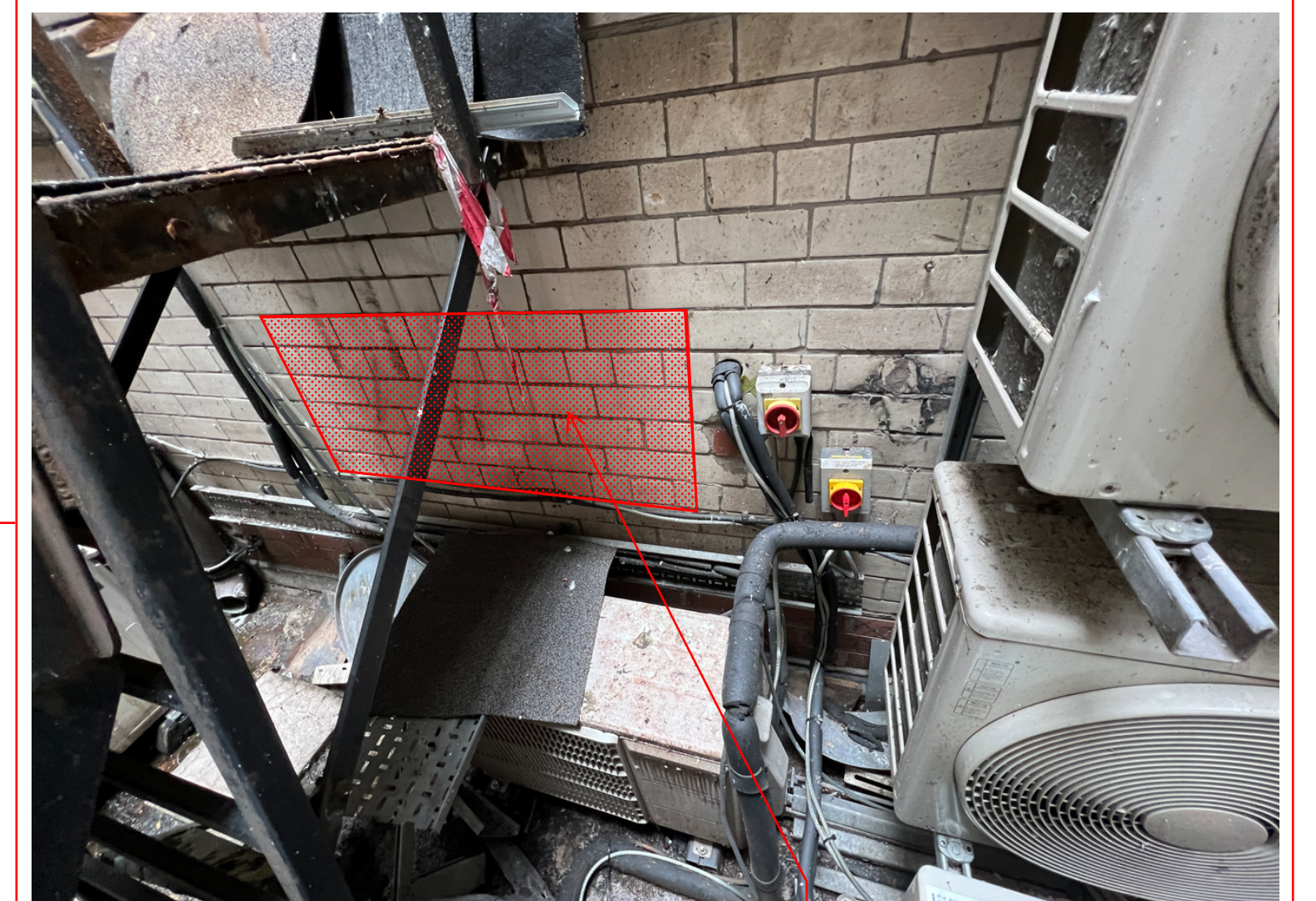
Section A-A (Side View) Existing View Photograph 002
