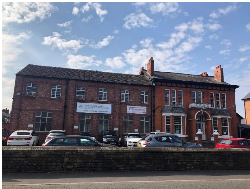
PLATE 9 SHOWING NORTHERN ASPECT OF BUILDING 2
