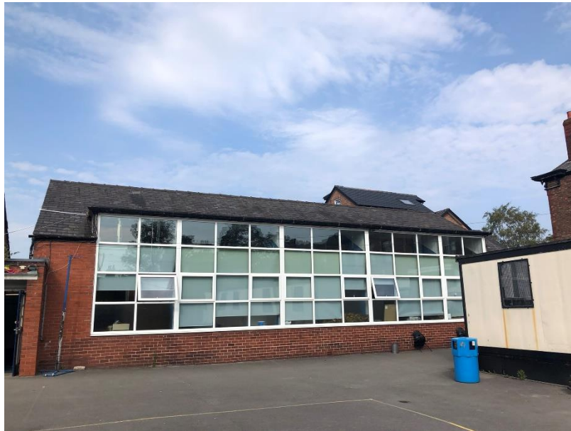
PLATE 6 SHOWING SCHOOL HALL SECTION OF BUILDING 1
