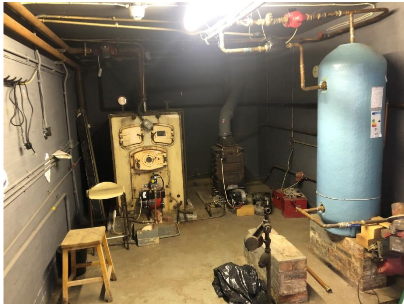
PLATE 16 SHOWING CELLAR INSIDE BUILDING 1
