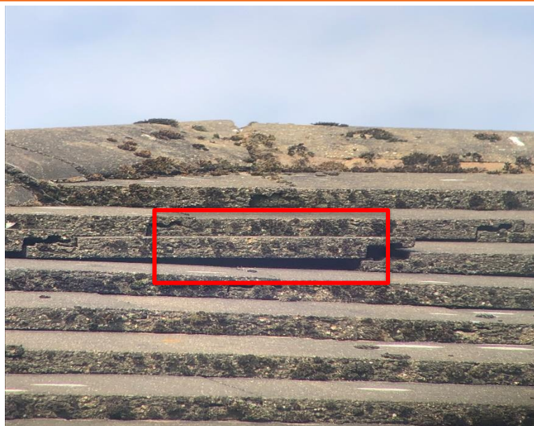
PLATE 5 SHOWING GAP UNDER TILE AT SOUTHERN END OF BUILDING 1
