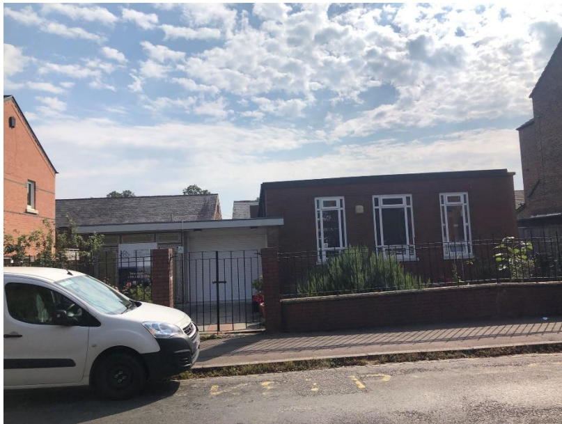
PLATE 1 SHOWING ENTRANCE ON WESTERN ASPECT OF BUILDING 1
