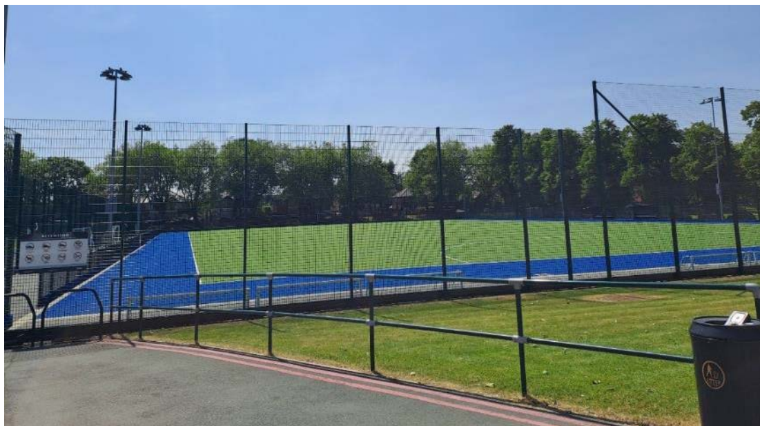
Figure 7: Sports pitch on site
