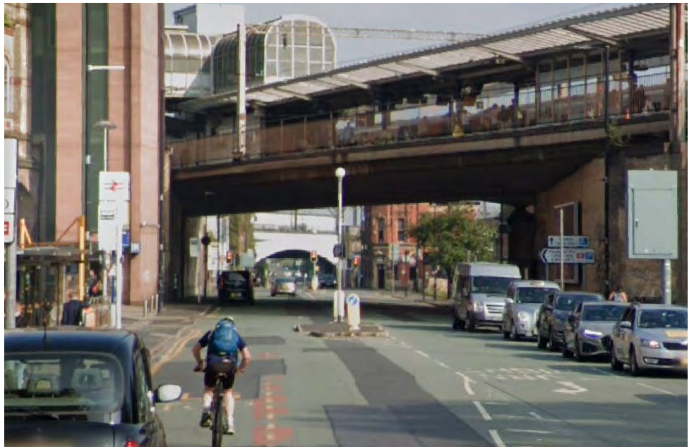
Plate 8 Star and Garter Public House viewed from Fairfield Street in vicinity of the Whitworth Street Conservation Area boundary (Source: Google Street View)
