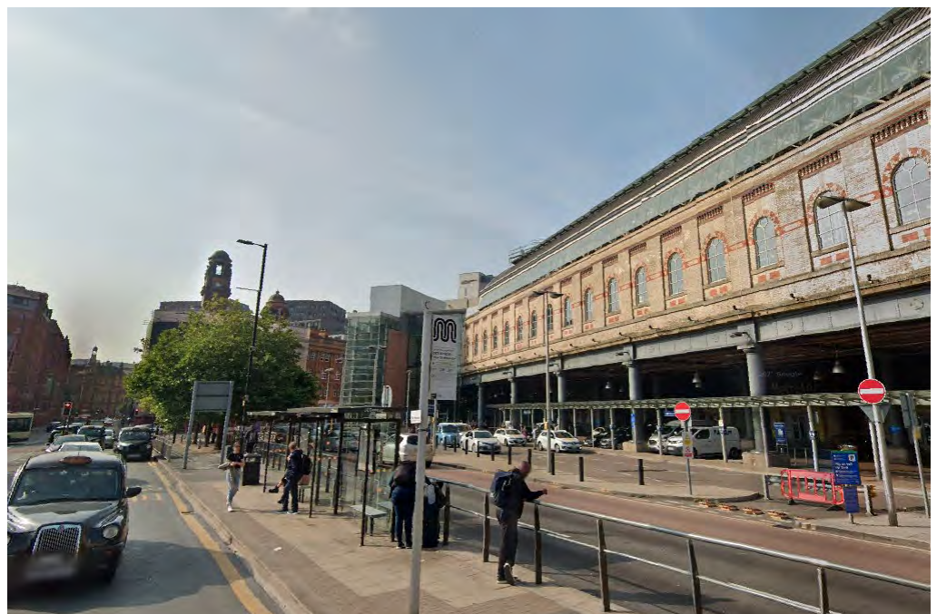
Plate 5 Grade II listed Train Shed and Undercroft viewed from Fairfield Street (Source: Google Street View)
