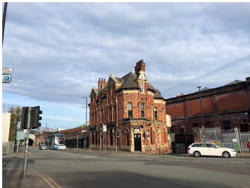
Plate 1 View of western elevation of the Star and Garter from Fairfield Road
