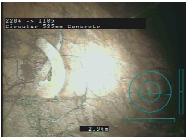
2204X_dced5df7-3818-4aeb-a04b-da4ec2573895_20191218_220723_457.jpg, 00:05:51, 2.94 m Roots, tap
