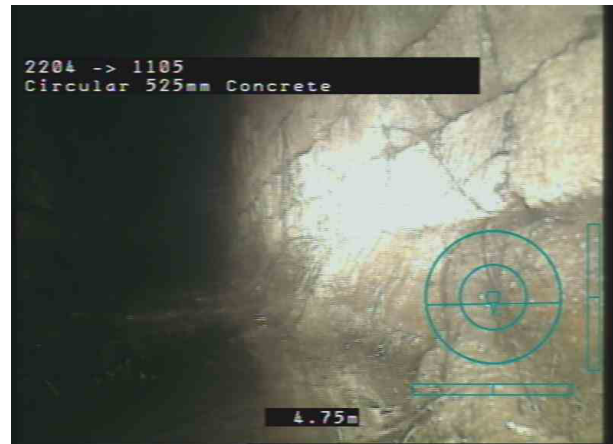
2204X_f012e500-f0fc-481b-b5e8-7461bc6394bf_20191218_220904_498.jpg, 00:07:33, 4.75 m Roots, tap
