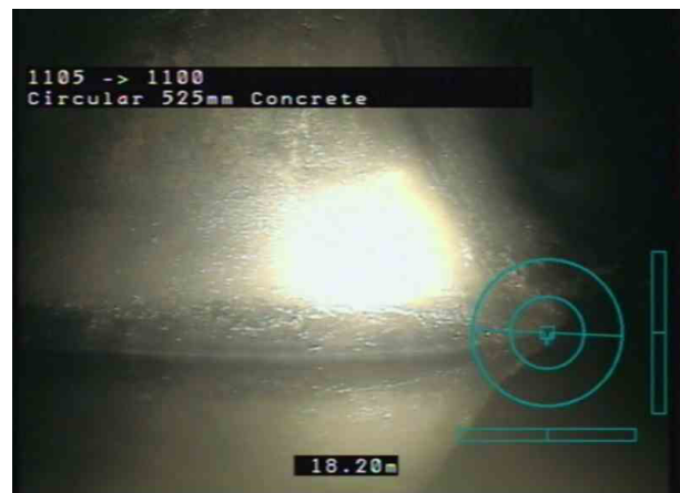
1105X_b4718763-4329-4ae5-8267-61e07a194c70_20200109_082429_832.jpg, 00:11:56, 18.20 m Settled deposits, coarse, 15% cross-sectional area loss, finish
