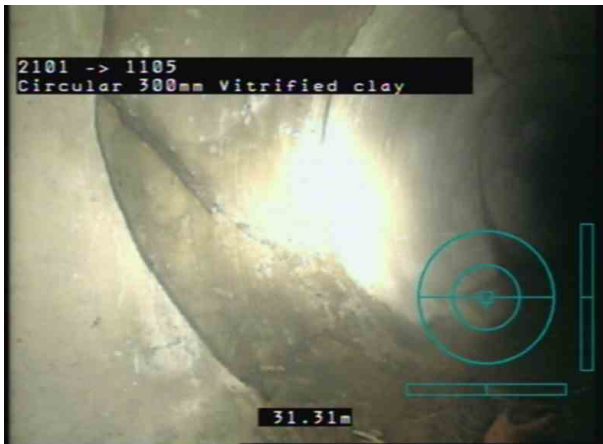
2101X_02b31859-62bb-4581-8431-ace2bb5bf4cd_20200109_082900_567.jpg, 00:14:31, 31.31 m Roots, fine
