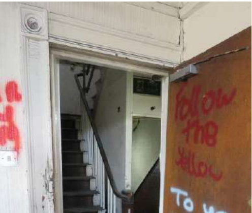
The original decorative architrave surrounding the door to be used as reference for other areas.
