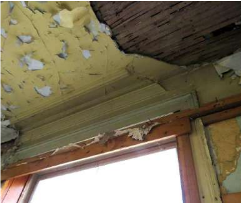
An area of newly uncovered original moulded timber window surround and plaster cornice above one of the windows to be used as a template.
