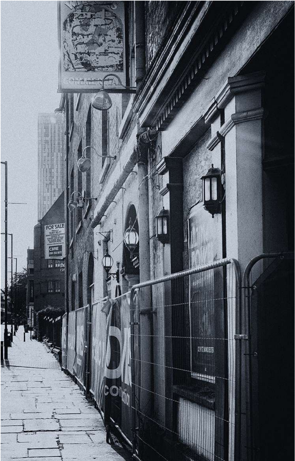
Current condition of the existing
