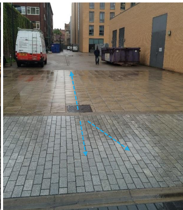
Image 2 - estimated overland flow paths for Manhole 5 (viewed south)
