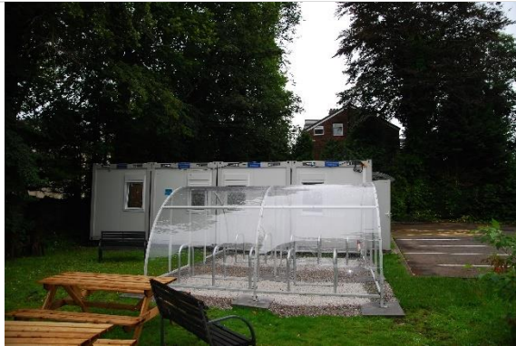
9. Internal view towards Eastern site boundary
