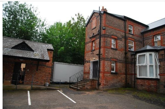
6. View from within site looking towards Southwest corner and main building.
