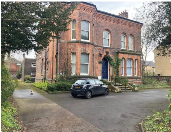
View of existing villa fronting Palatine Road
