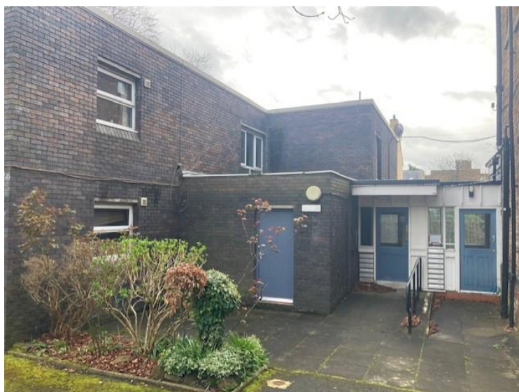
View looking southwards of the rear extension proposed to be demolished
