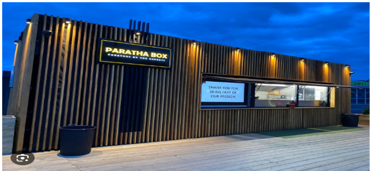
Image of a 40 feet shipping container clad in timber with serving window
