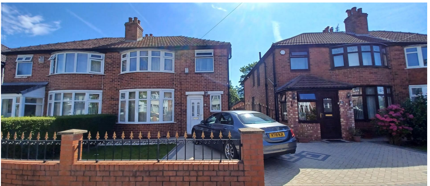
Figure 4. Principal elevation of No.11 Shireoak Road.
