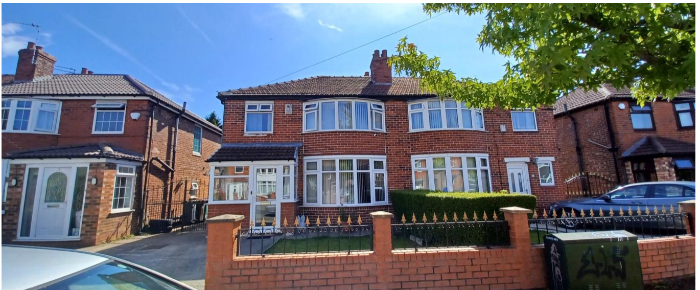
Figure 3. Principal elevation of No.9 Shireoak Road.
