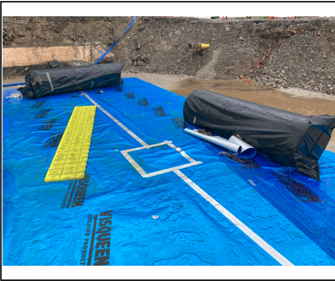
Patch repair- square of membrane
