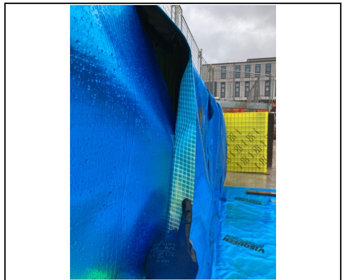
Visqueen pro jointing tape up the
