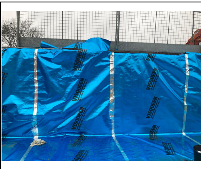
Dual taped lap joints up the pecafiled
