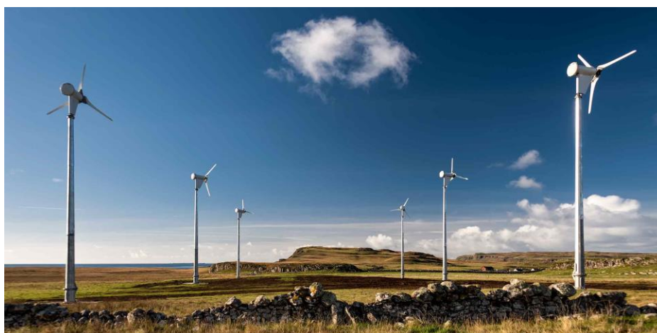
Figure 7: Typical Small Scale 6kW Wind Turbine
