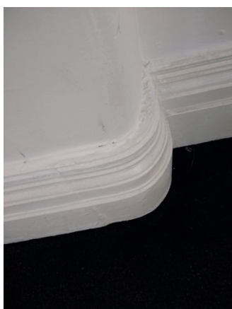
Images 22, 23, 24: Showing original door with recessed panels; modern replica door flush face with added frames; detail of typical deep and high skirting.
