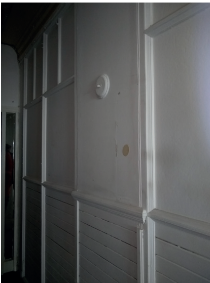
Images 16, 17, 18: Typical ceiling cornicing, evidencing historic room layout; typical examples of partitions with timber panels and painted glass, forming internal corridors.
