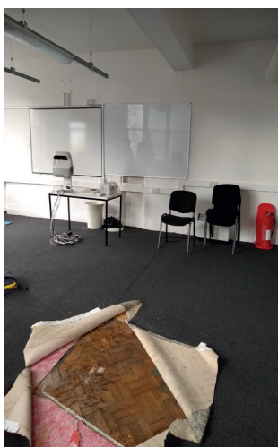
Images 14, 15: Showing modern carpet removed to expose parquet flooring to third floor and typical timber floorboards (second floor).
