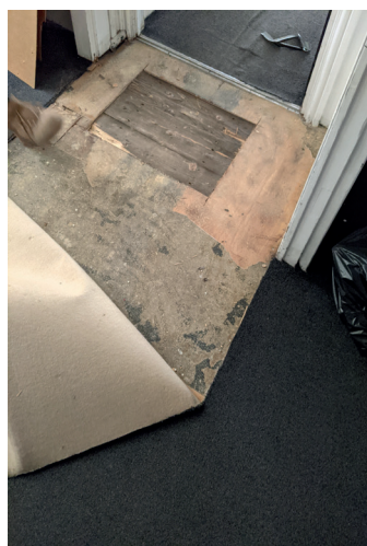
Images 14, 15: Showing modern carpet removed to expose parquet flooring to third floor and typical timber floorboards (second floor).
