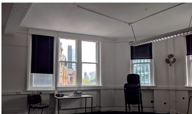
Image 13: Showing typical original sash one over one window forms, second floor. All sashes to be retained, repaired and secondary glazing fitted if required.
