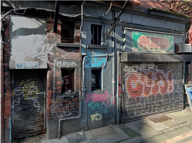
Image 28: Showing part of Back Piccadilly elevation, with two small lower windows to be removed to allow for new bin access doors.
