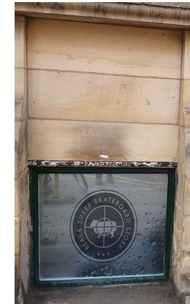
Photo of stonework at No.16 Newton Street to be replicated on the facade of No.14
