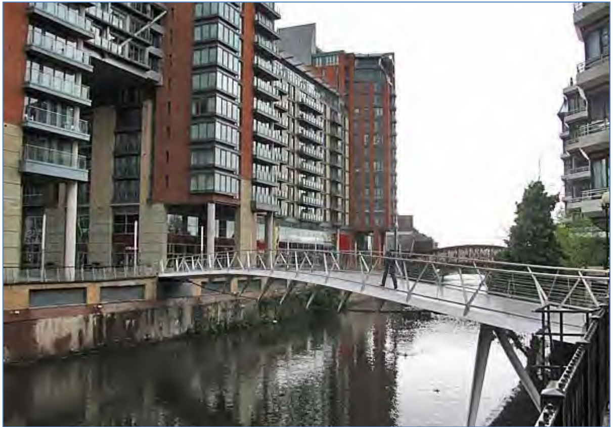
Figure 3.2 Irwell Pedestrian Footbridge
