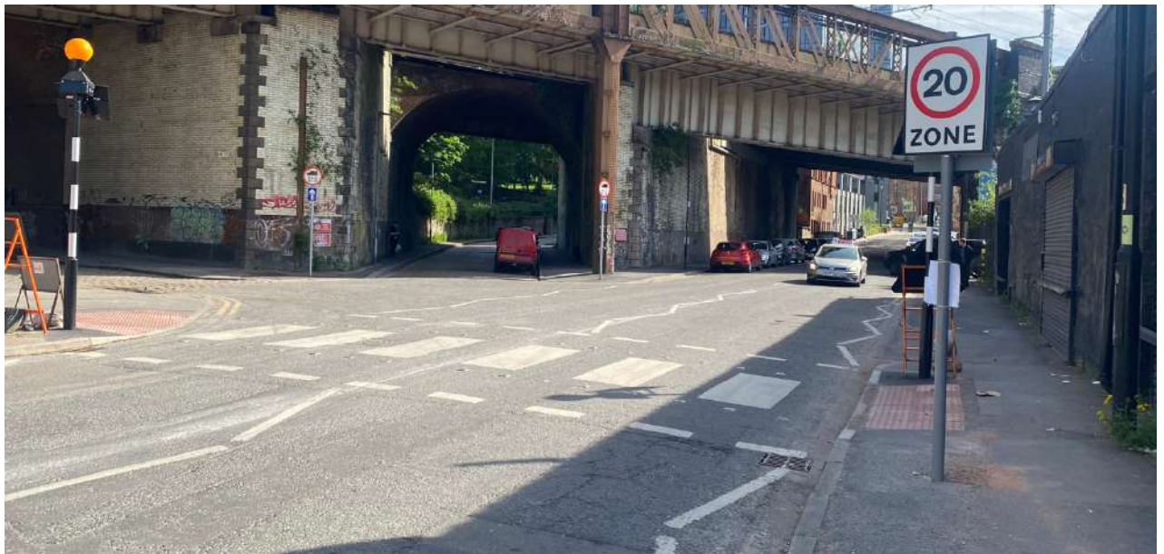
Photograph 2.5 : Dantzic Street - Southbound
