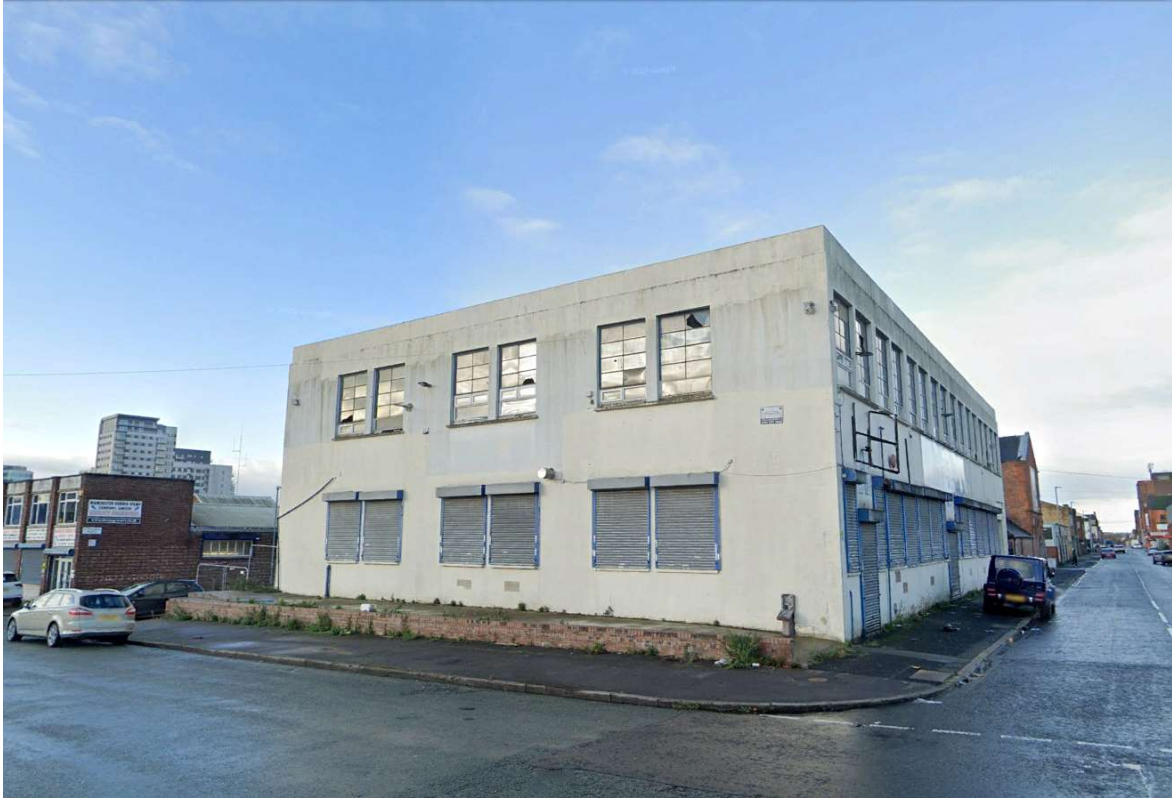
Figure 3 Red Bank Road - Derby Street corner
