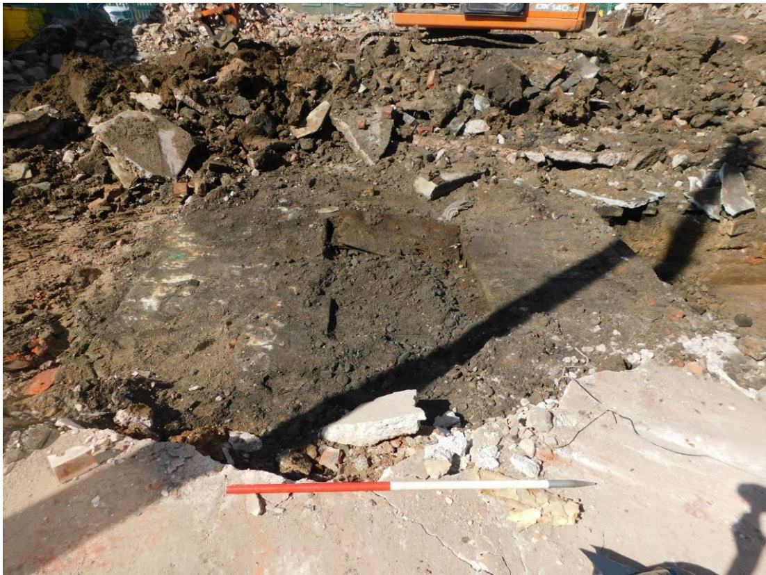
Plate 4: Trench 1 showing structural remains, looking south-west, scale: 1m.
