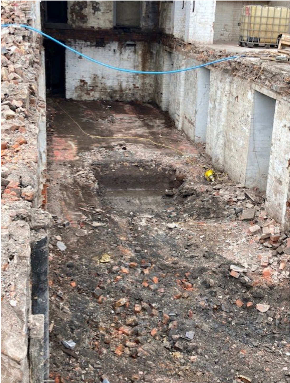
Plate 9: Monitored excavation of open basement, looking north-west .
