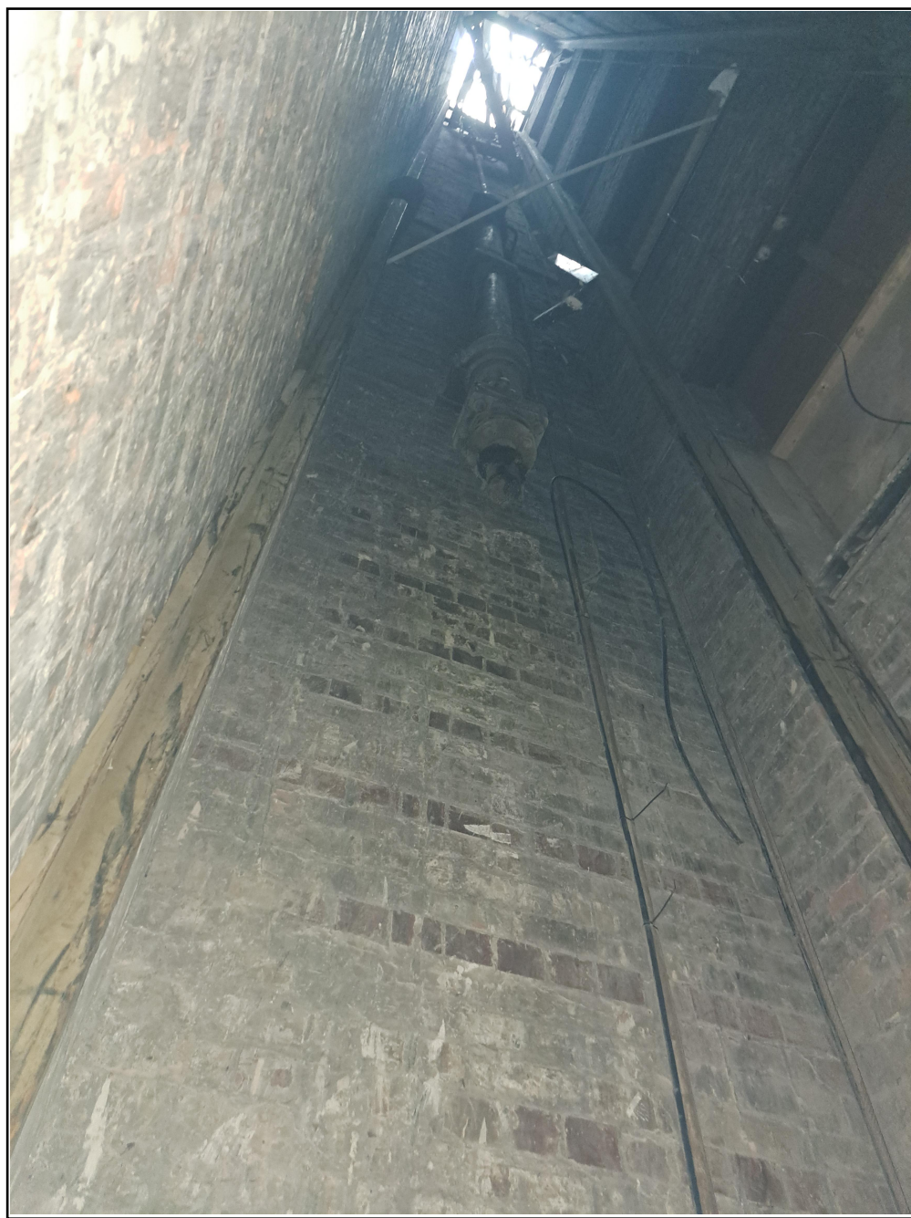
Image 1 Existing dis-used lift riser - existing landing entrances blocked in and redundant services will need to be stripped out
