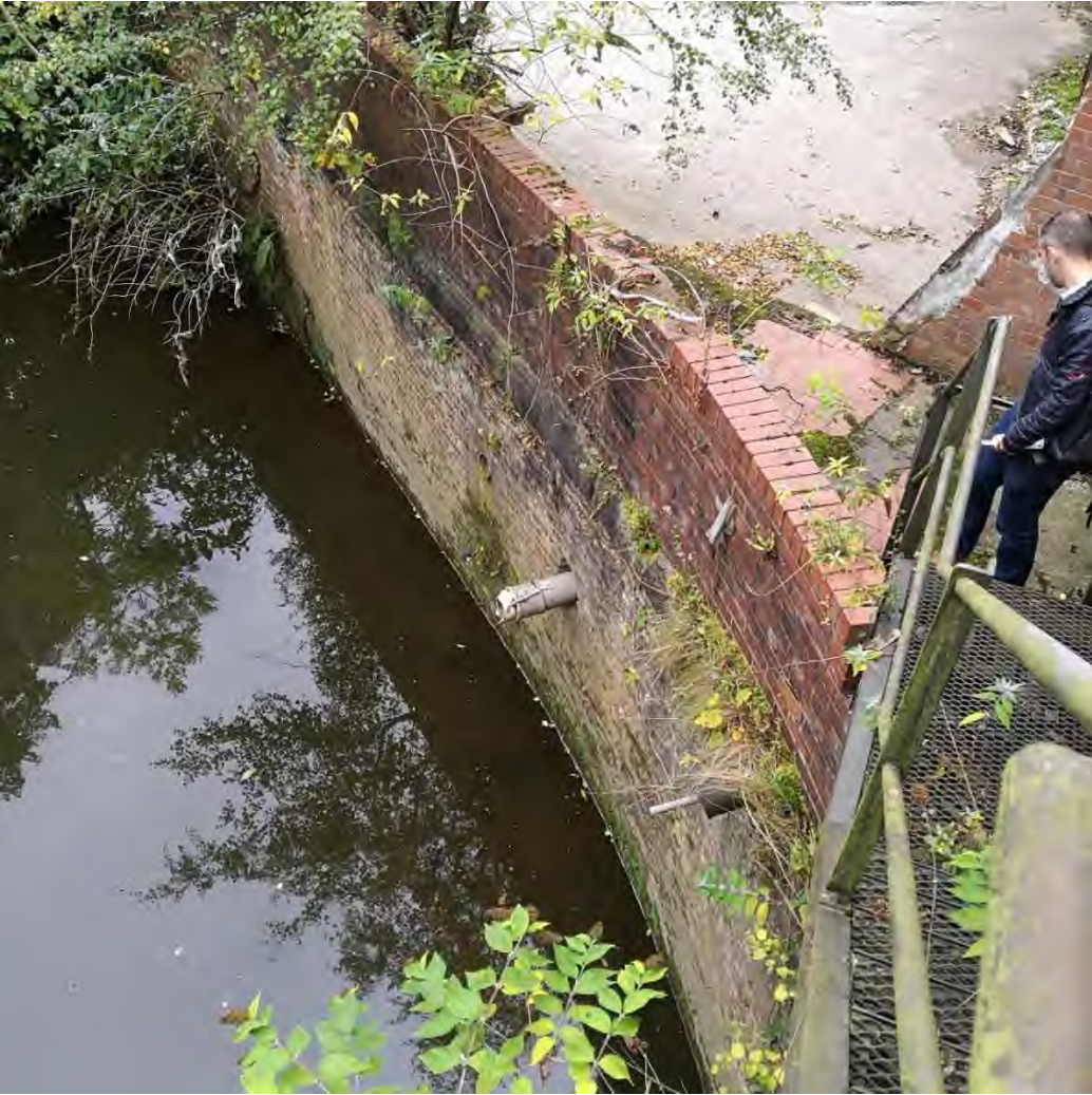
Figure 5-1 Existing Outfall Observed During Site Visit
