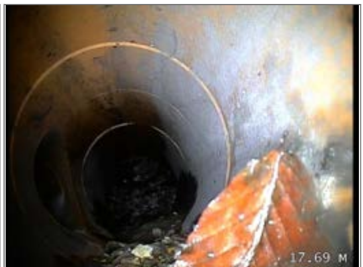
Junction at 9 o'clock, diameter 100mm
