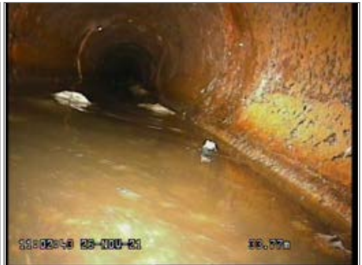
Survey abandoned - Remark: UNABLE TO PASS DUE TO FOUL AND SILT DEPOSITS
