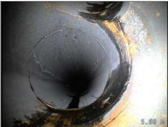
Junction at 1 o'clock, diameter 100mm
