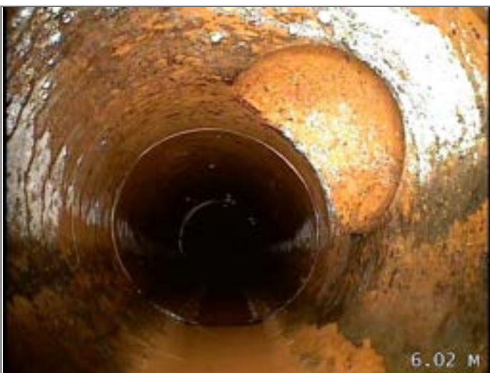
Junction at 2 o'clock, diameter 100mm
