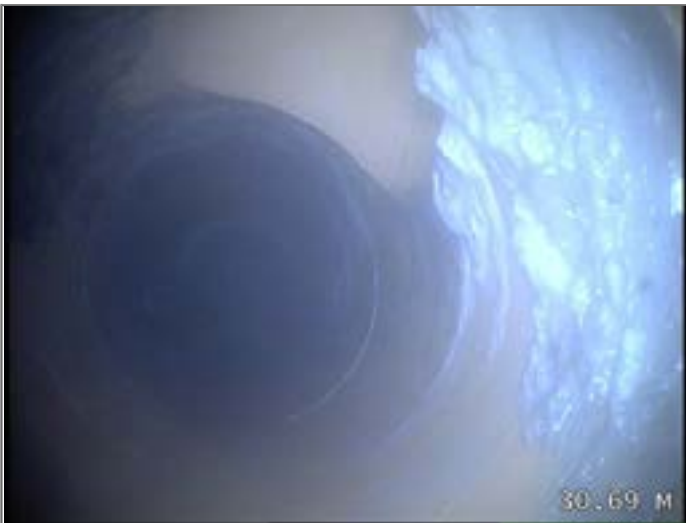
Junction at 1 o'clock, diameter 100mm
