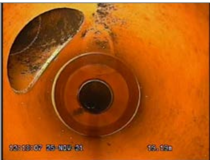
Junction at 10 o'clock, diameter 100mm
