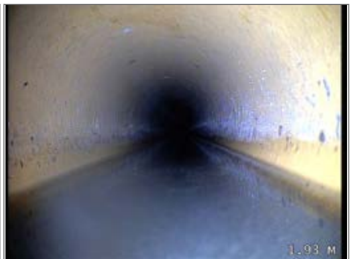
Water level 10% height/diameter
