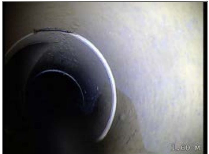
Junction at 9 o'clock, diameter 100mm
