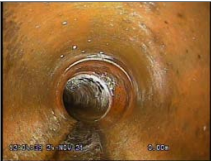
Start node type, manhole, reference MH F8
