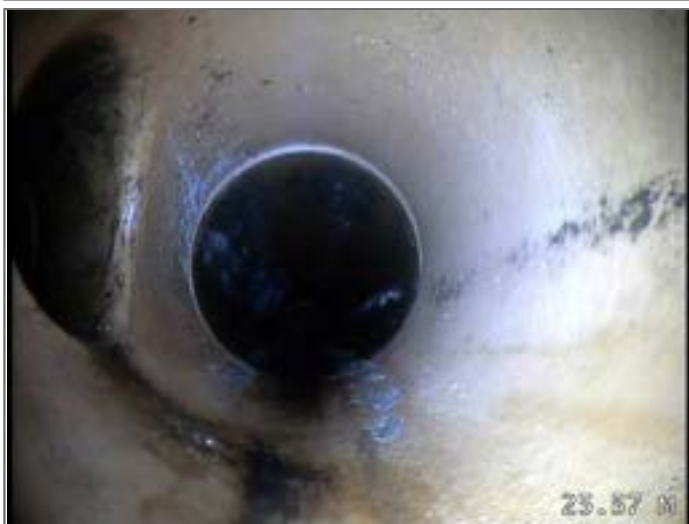
Junction at 9 o'clock, diameter 100mm
