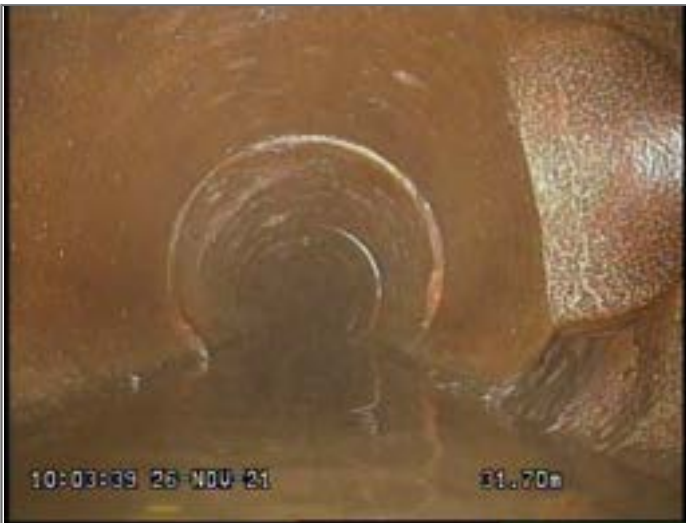
Junction at 3 o'clock, diameter 150mm
