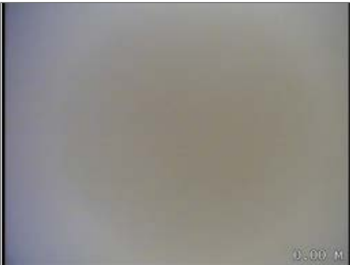
Loss of vision, camera under water - Remark: HOLDING WATER DIP IN PIPE
