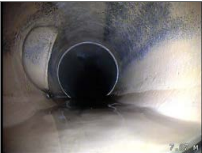
Junction at 9 o'clock, diameter 100mm
