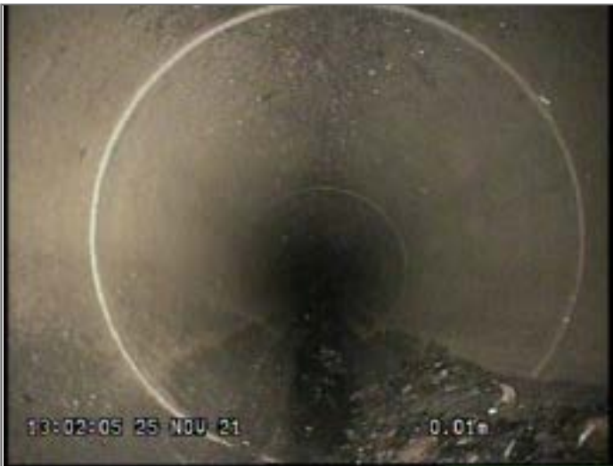
Start node type, manhole, reference MH S12
