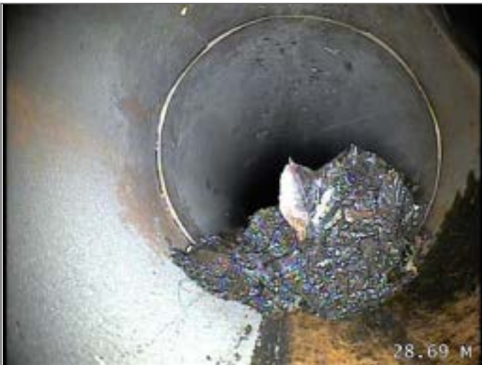
Junction at 2 o'clock, diameter 100mm
