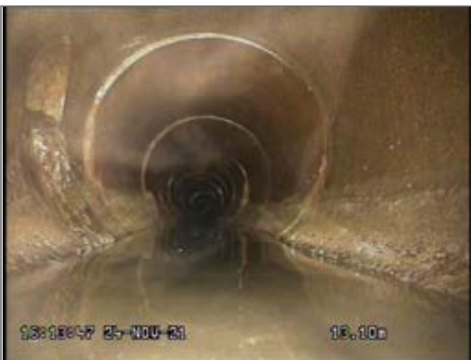
Junction at 10 o'clock, diameter 150mm
