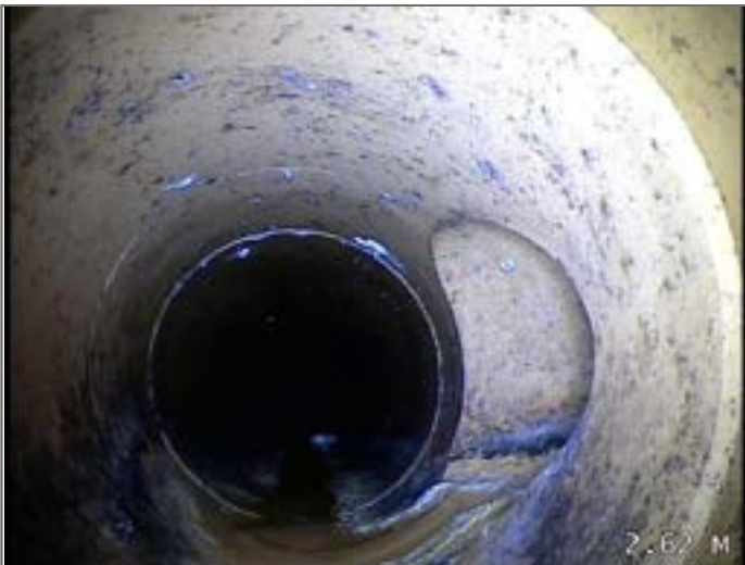
Junction at 3 o'clock, diameter 100mm
