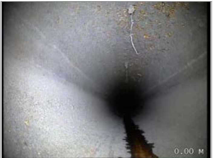
Water level 5% height/diameter
