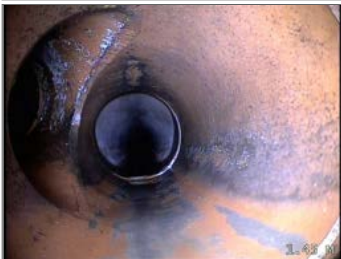
Junction at 10 o'clock, diameter 100mm
