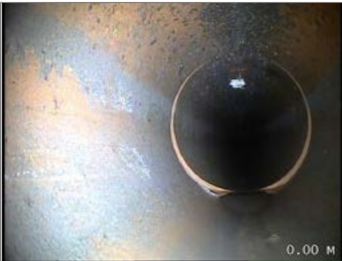
Start node type, manhole, reference MH S15
