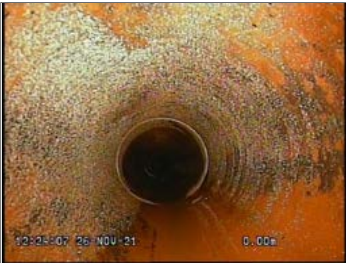
Start node type, manhole, reference MH S3
