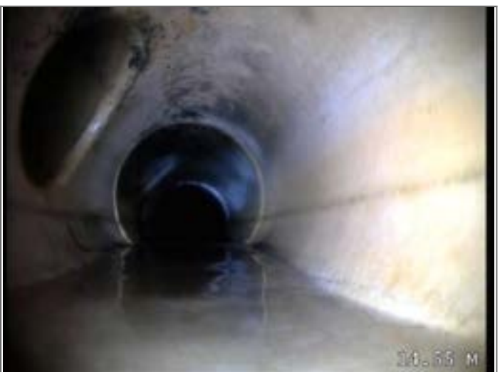
Junction at 10 o'clock, diameter 100mm
