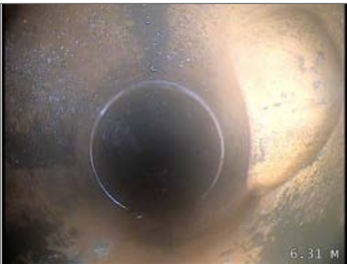
Junction at 3 o'clock, diameter 100mm
