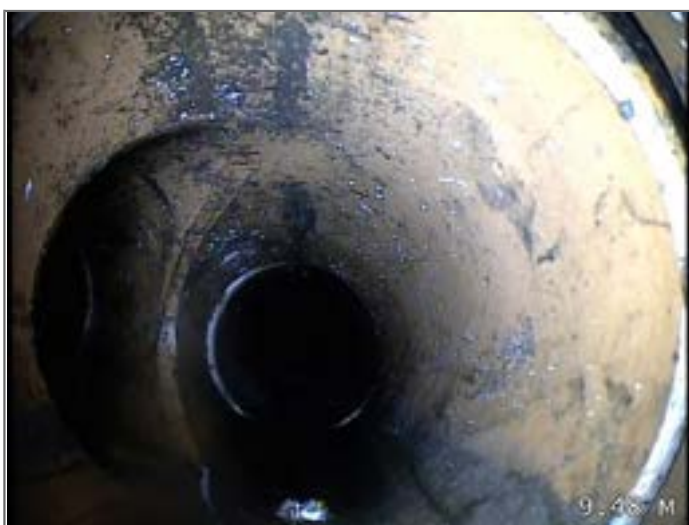
Junction at 9 o'clock, diameter 100mm
