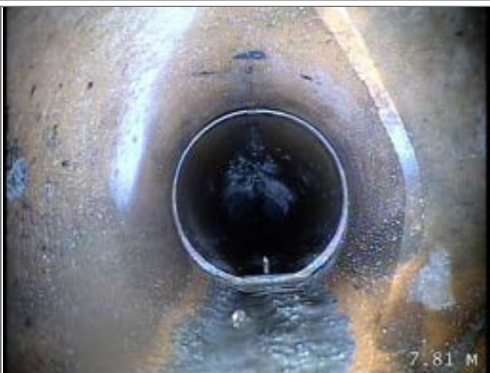
Junction at 3 o'clock, diameter 100mm
