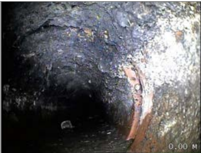
Start node type, manhole, reference MH S3
