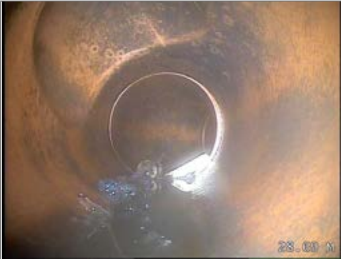
Junction at 11 o'clock, diameter 150mm
