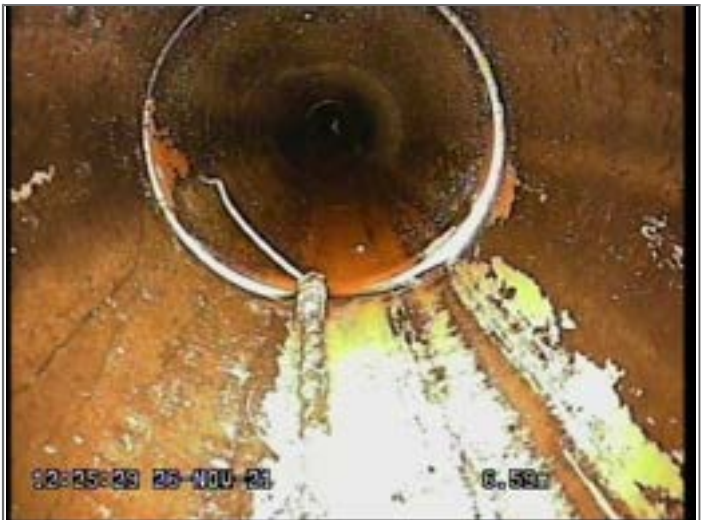
Other settled deposits 5% cross-sectional area loss - Remark: METAL OBJECT
