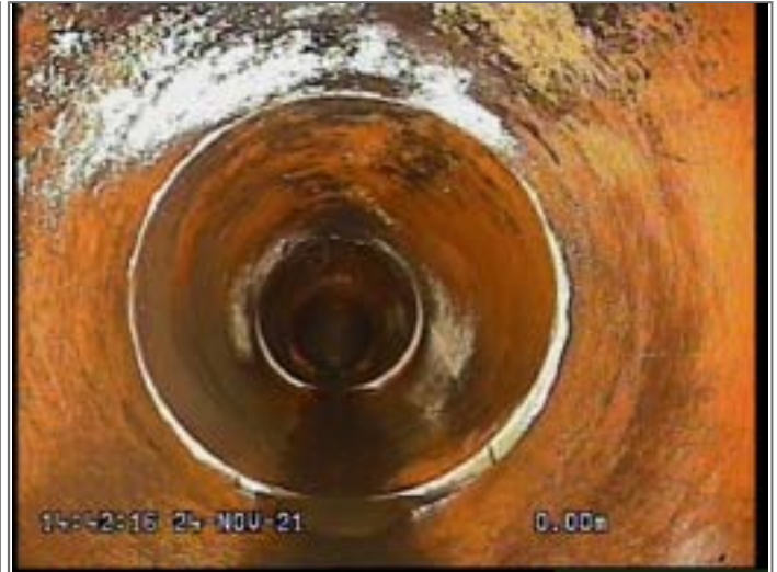
Water level 5% height/diameter
