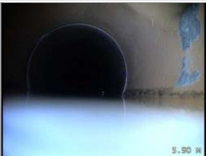
Junction at 2 o'clock, diameter 100mm
