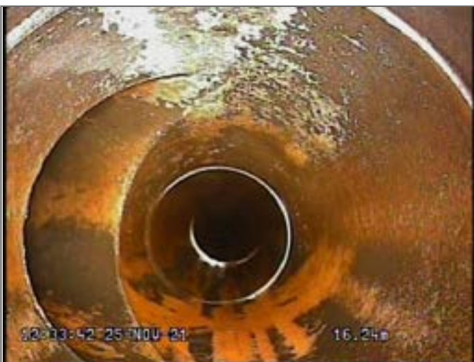
Junction at 9 o'clock, diameter 150mm
