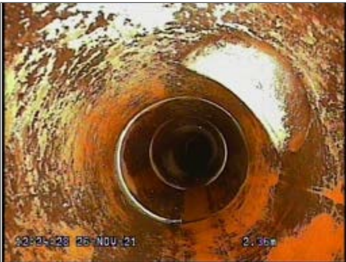
Junction at 2 o'clock, diameter 100mm
