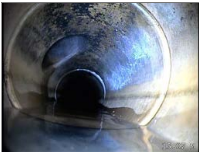
Junction at 10 o'clock, diameter 100mm
