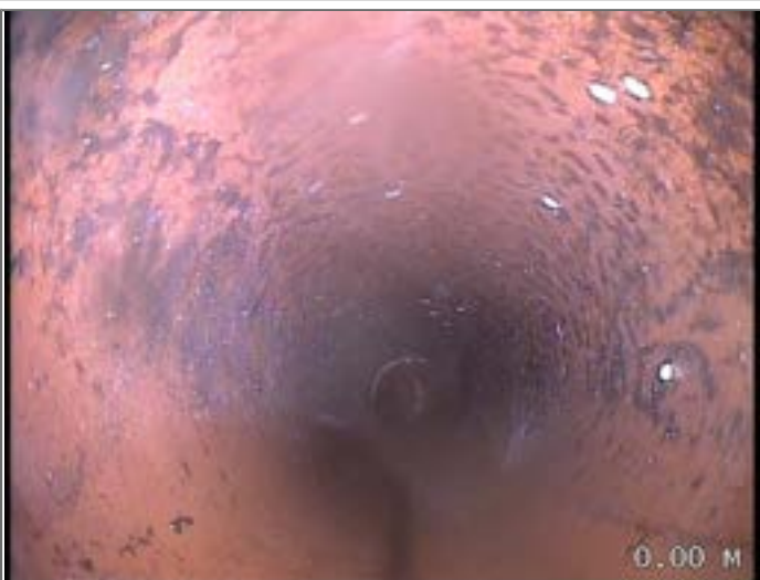
Water level 5% height/diameter
