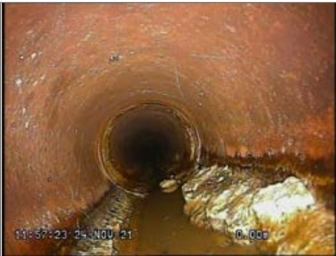
Start node type, manhole, reference MH F5
