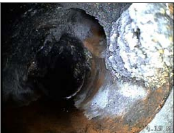
Junction at 1 o'clock, diameter 100mm
