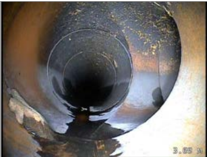
Junction at 3 o'clock, diameter 150mm
