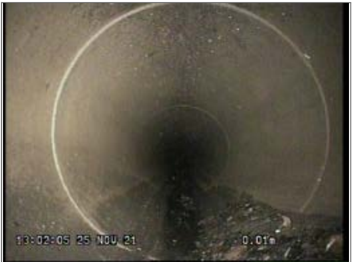
Water level 5% height/diameter
