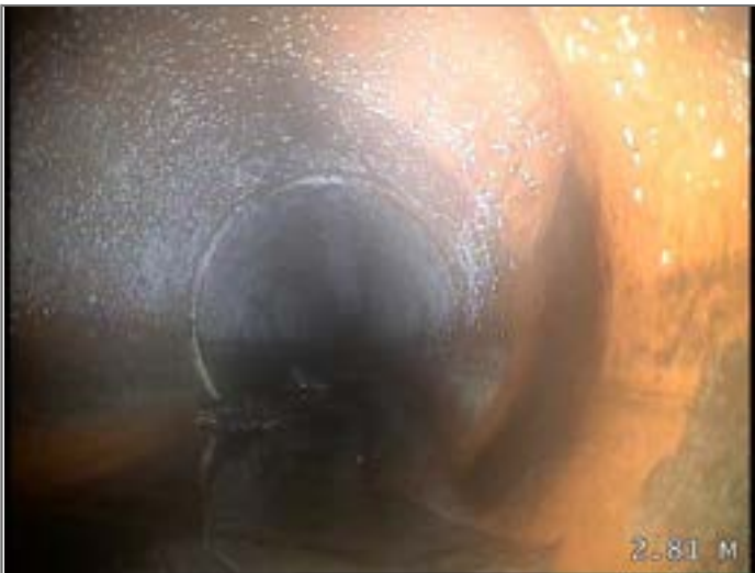
Junction at 1 o'clock, diameter 100mm
