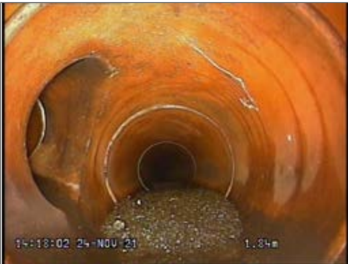
Junction at 9 o'clock, diameter 150mm
