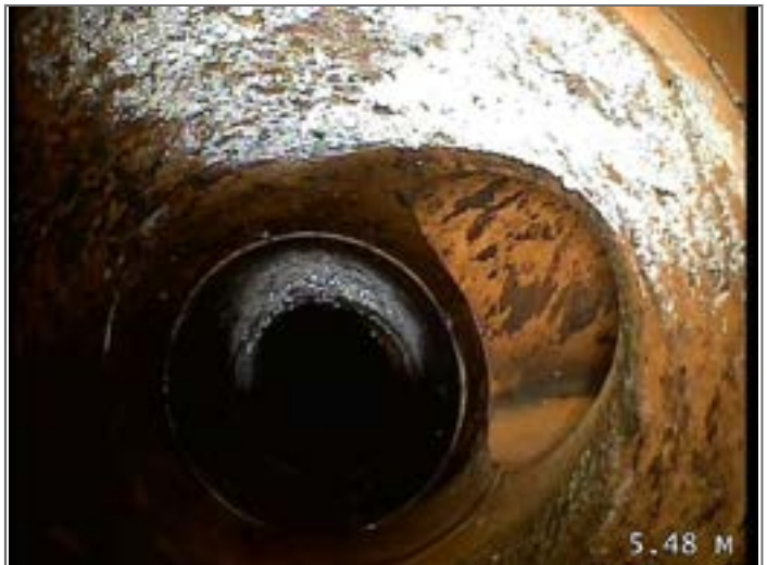
Junction at 3 o'clock, diameter 100mm
