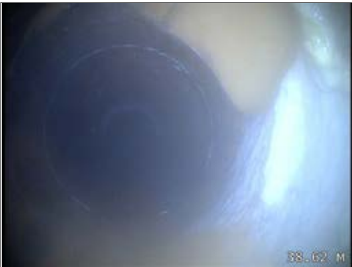
Junction at 1 o'clock, diameter 100mm
