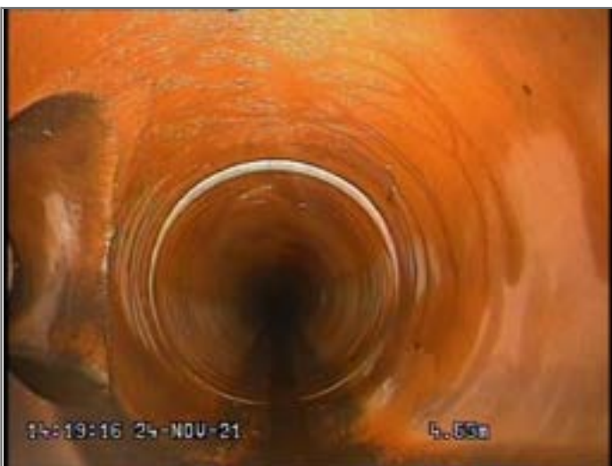
Junction at 9 o'clock, diameter 150mm
