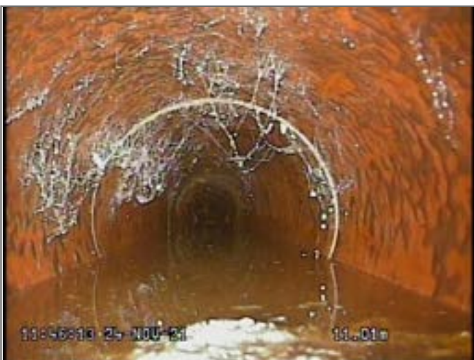
Other settled deposits 10% cross-sectional area loss - Remark: FOUL WASTE
