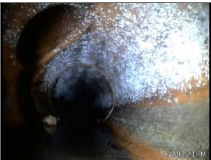
Junction at 10 o'clock, diameter 100mm
