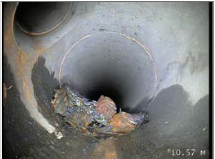
Junction at 11 o'clock, diameter 100mm
