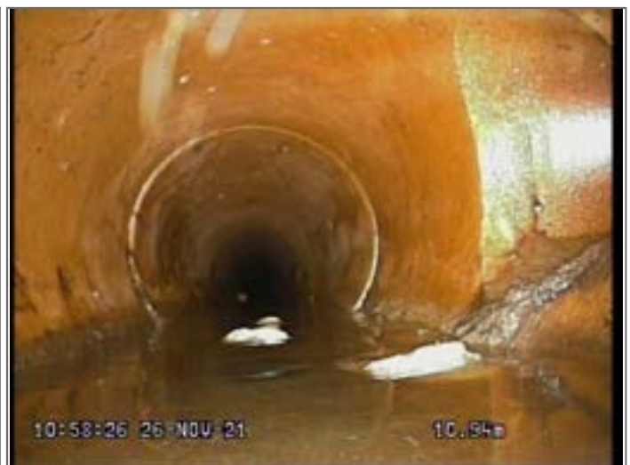
Junction at 3 o'clock, diameter 150mm
