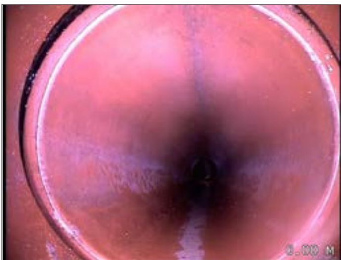
Start node type, manhole, reference MH S6
