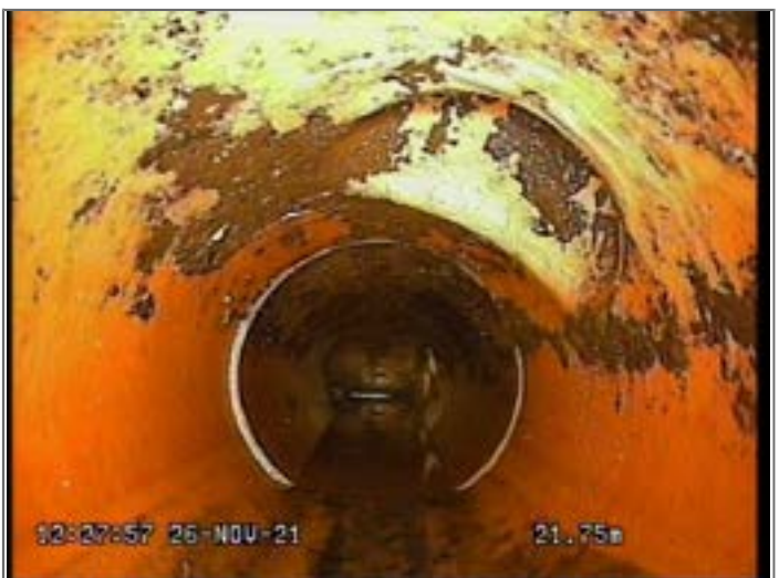
Junction at 1 o'clock, diameter 100mm
