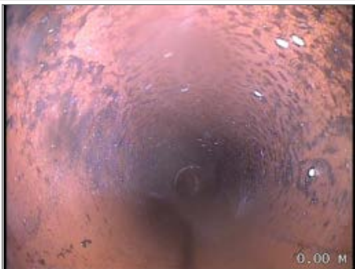
Start node type, manhole, reference MH F1
