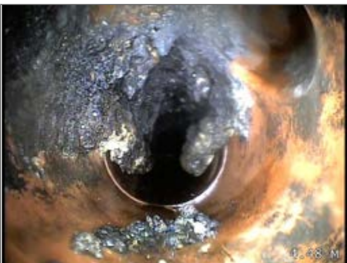
Junction at 2 o'clock, diameter 100mm
