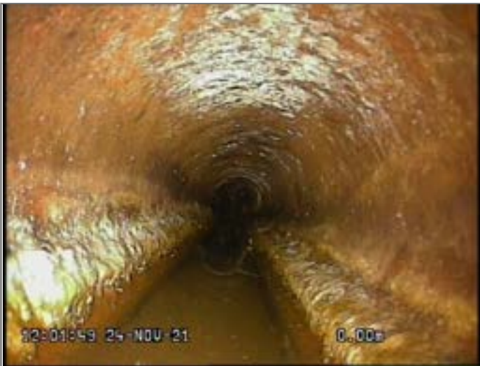
Start node type, manhole, reference MH F7
