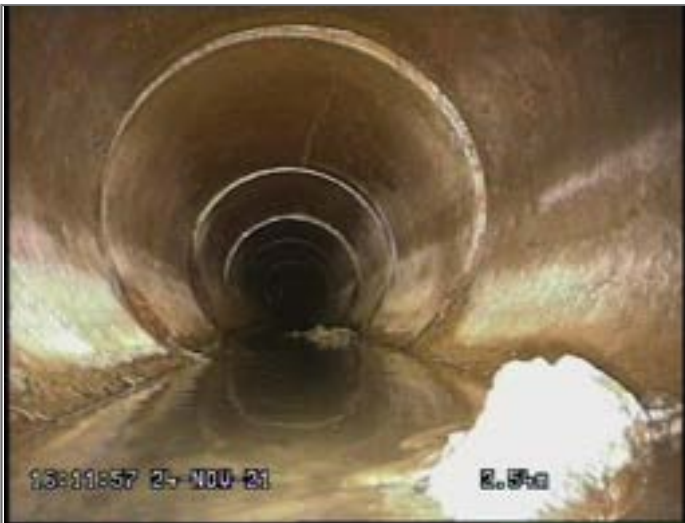
Start node type, manhole, reference UU 2301
