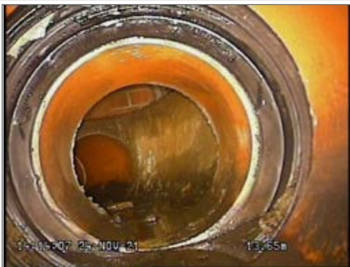
Open joint large
