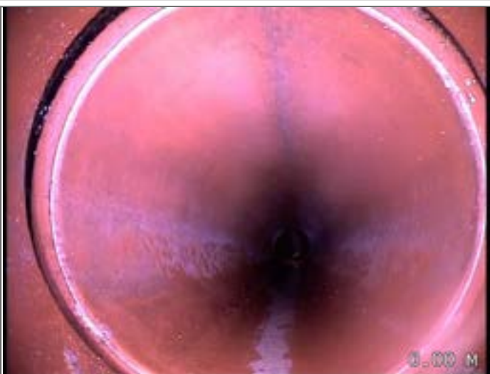
Water level 5% height/diameter
