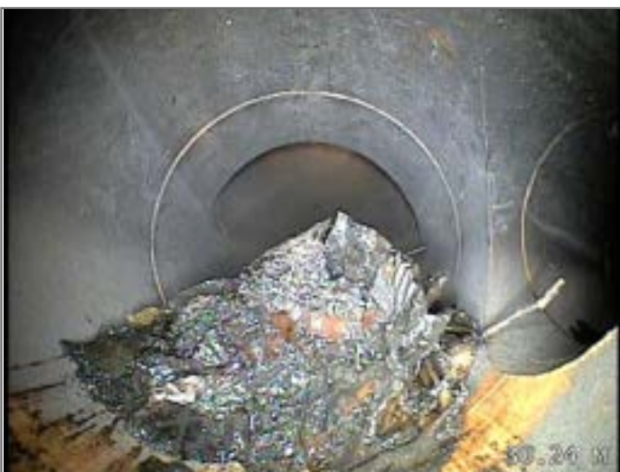
Junction at 3 o'clock, diameter 100mm
