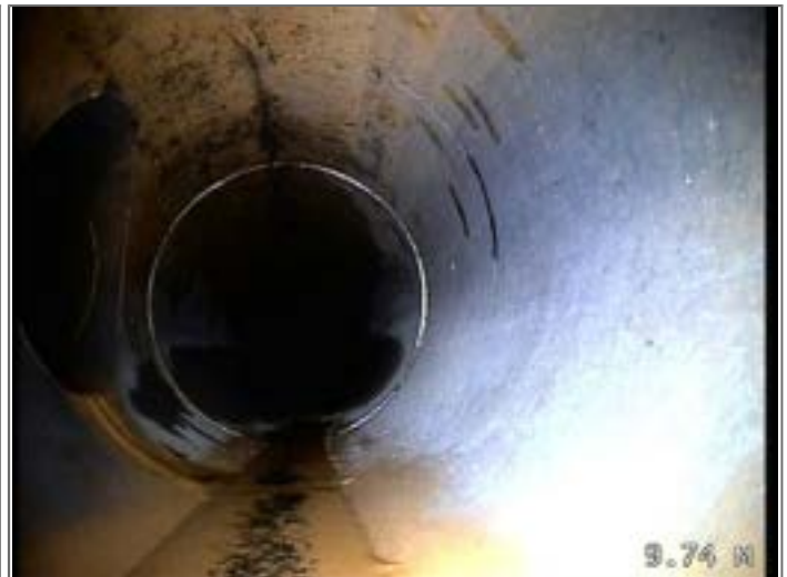
Junction at 9 o'clock, diameter 100mm
