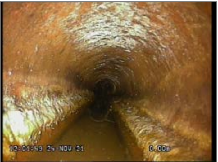
Water level 5% height/diameter
