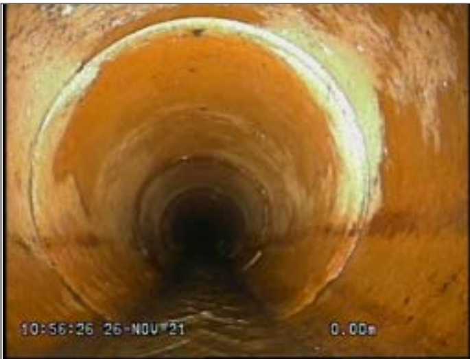
Start node type, manhole, reference UU 0402
