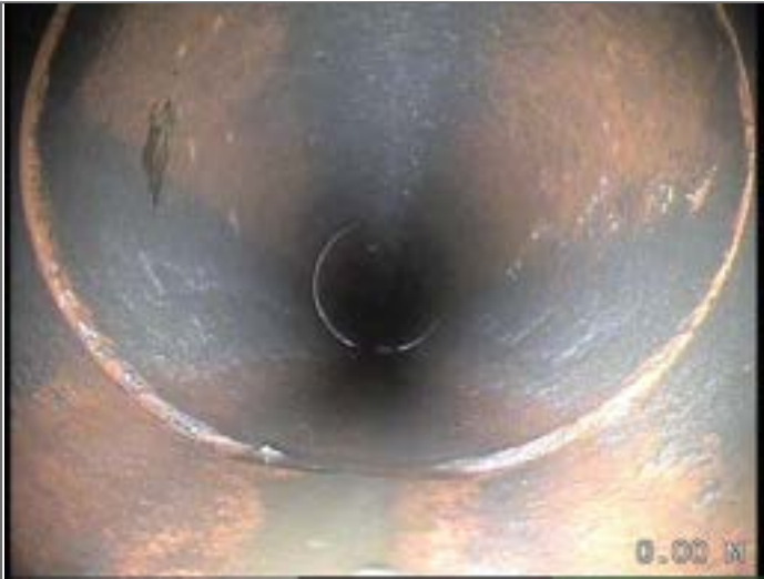
Water level 5% height/diameter
