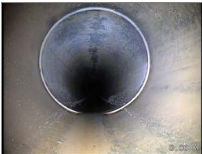
Start node type, manhole, reference MH S5
