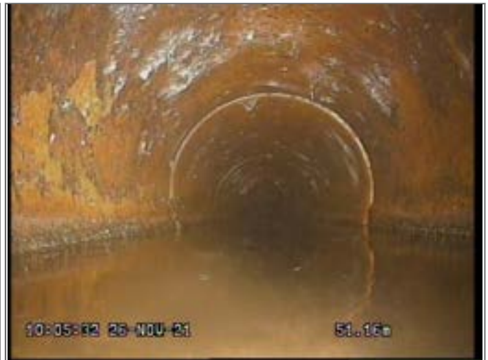
Water level 25% height/diameter
