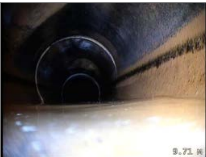
Junction at 11 o'clock, diameter 100mm
