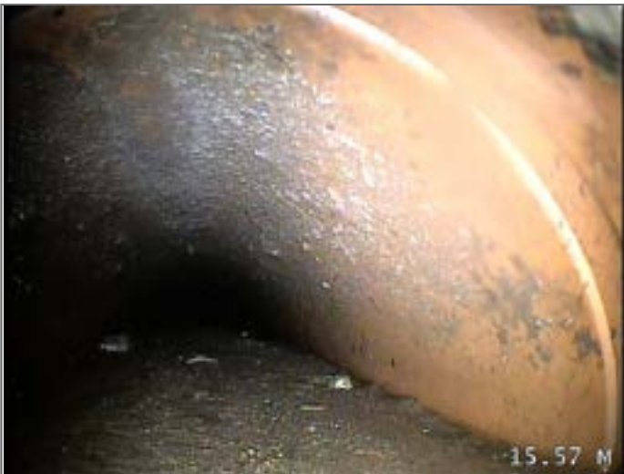
Survey abandoned - Remark: UNABLE TO PASS DUE TO HIGH SILT DEPOSITS
