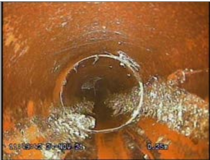
Start node type, manhole, reference MH F3
