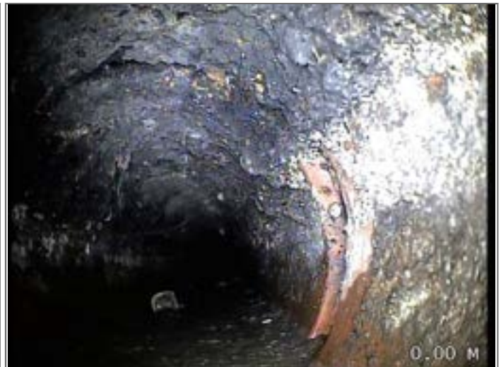
Other attached deposits from 8 to 4 o'clock 5% cross-sectional area loss - Remark SILT
