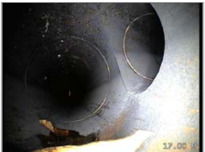
Junction at 2 o'clock, diameter 100mm
