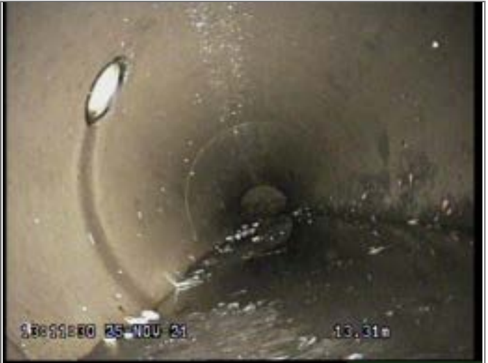
Survey abandoned - Remark: UNABLE TO PASS DUE TO HIGH SILT DEPOSITS - CLEANING REQUIRED
