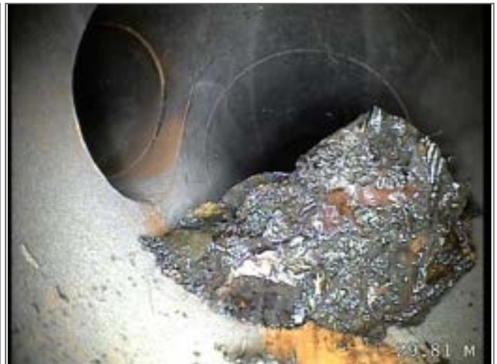
Junction at 10 o'clock, diameter 100mm
