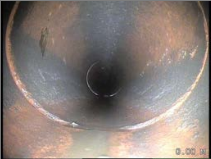
Start node type, manhole, reference MH S16
