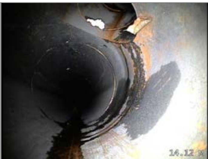
Junction at 1 o'clock, diameter 100mm
