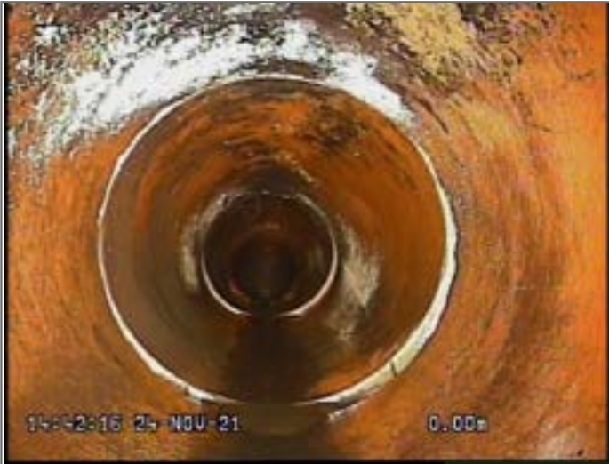
Start node type, manhole, reference MH S7
