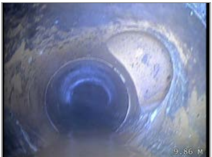
Junction at 2 o'clock, diameter 100mm
