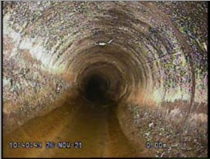
Start node type, manhole, reference UU 1303
