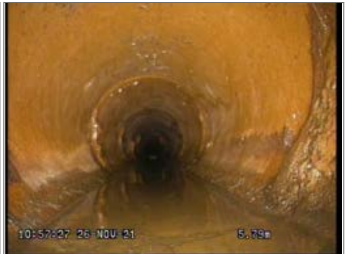
Attached deposits, encrustation from 12 to 12 o'clock 5% cross-sectional area loss, Start
