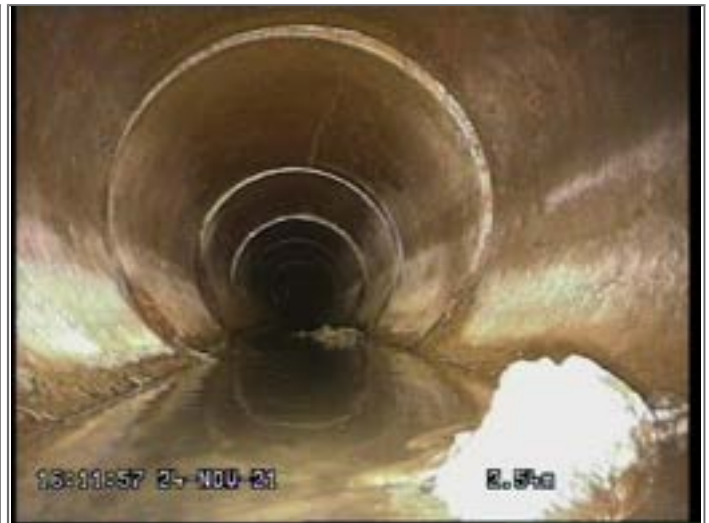
Water level 10% height/diameter
