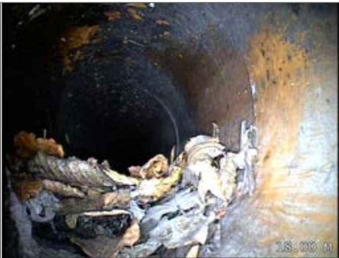
Other settled deposits 10% cross-sectional area loss - Remark: DEBRIS
