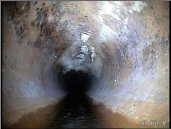
Start node type, manhole, reference MH F1
