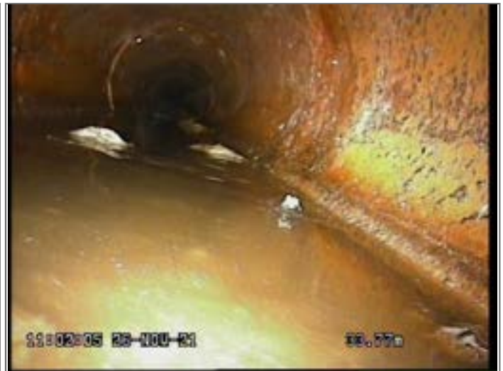
Attached deposits, encrustation from 12 to 12 o'clock 5% cross-sectional area loss, Finished
