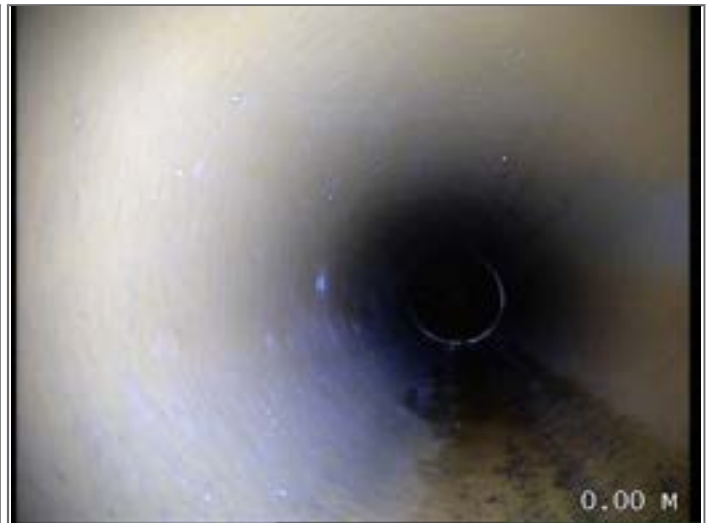
Water level 5% height/diameter
