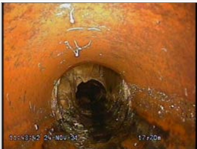
Start node type, manhole, reference MH F4
