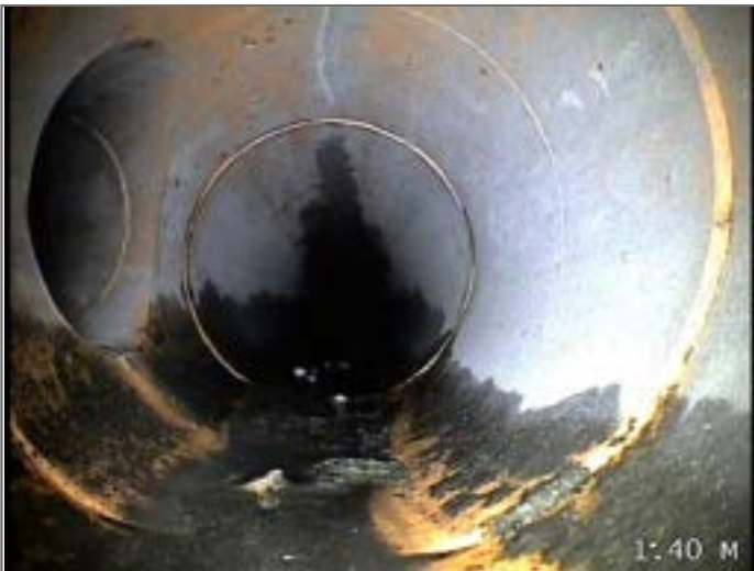
Junction at 9 o'clock, diameter 100mm
