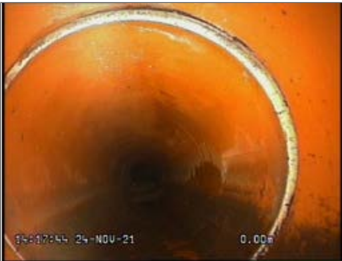
Start node type, manhole, reference MH S8
