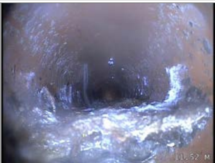
Attached deposits, encrustation from 4 to 8 o'clock 20% cross-sectional area loss
