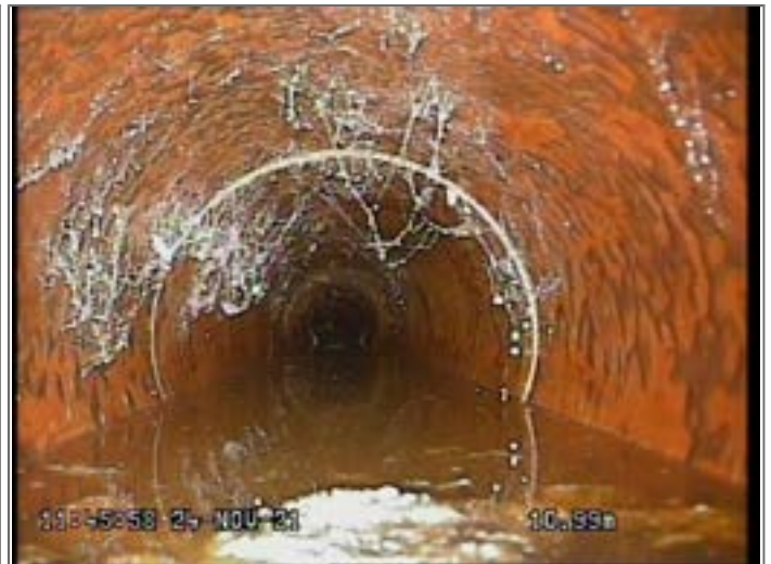
Water level 25% height/diameter
