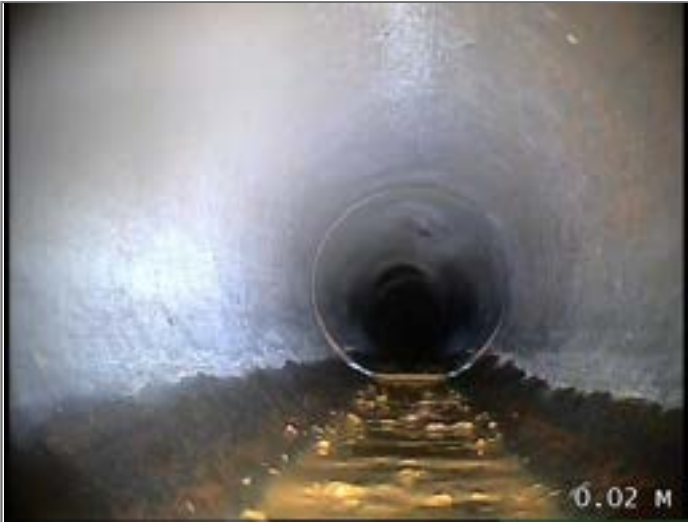
Start node type, manhole, reference UU 2301
