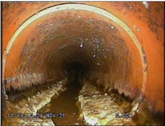
Start node type, manhole, reference MH F5
