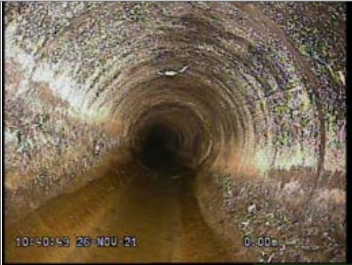
Water level 5% height/diameter
