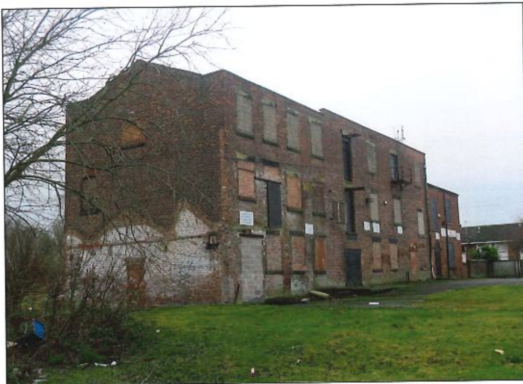
Plate 13: Remains of Daisy Bank Mill, 2017. Note the 'ghost' of a former 'saw-toothed' structure against the east elevation, which is likely to have been the site of the weaving shed.
