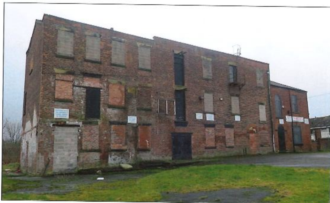
Plate 15: 2017 image of the warehouse, with attached dwelling at western end.
