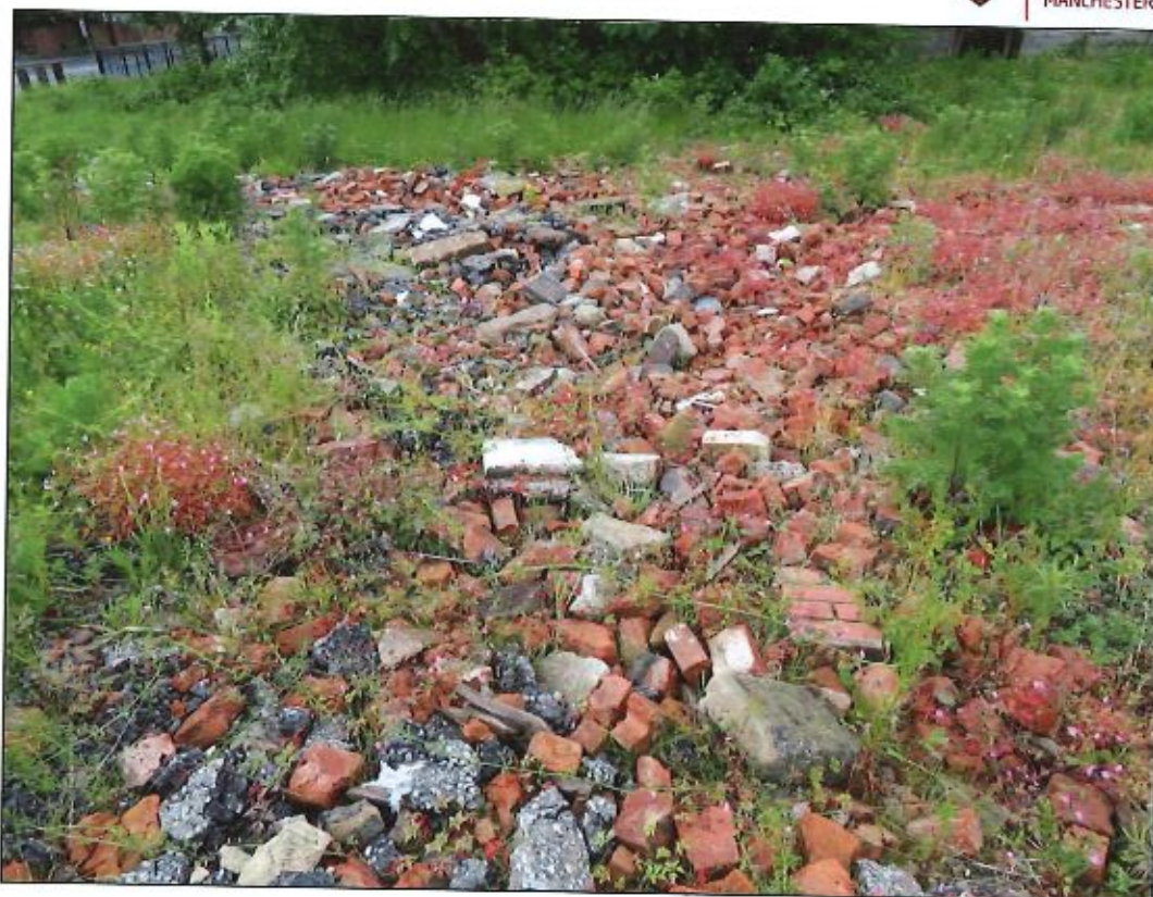
Plate 17: Demolition rubble at the site of Daisy Bank Mill, June 2019
