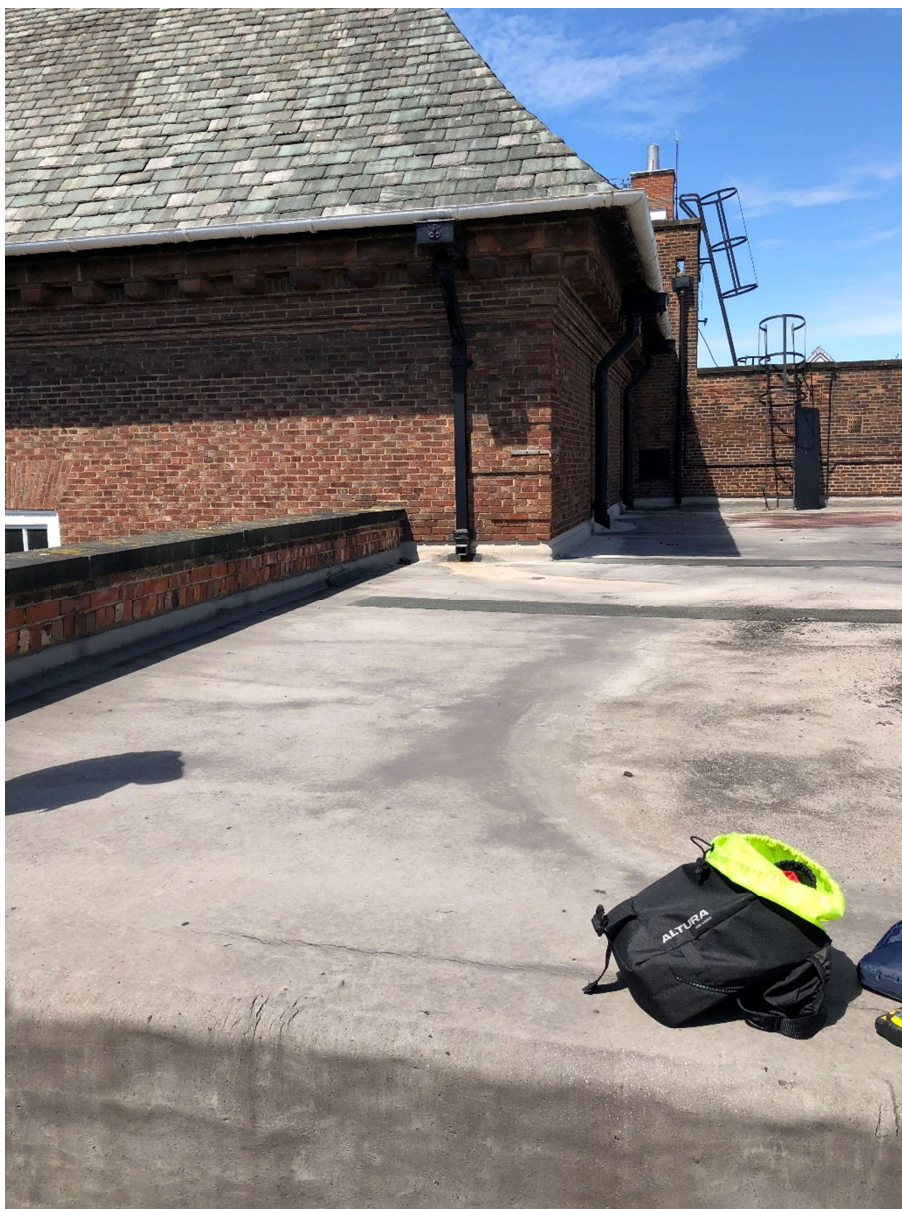
Photo 7: View of roof 5 towards roof 4 parapet and hooped ladder. Note RWPs discharging onto flat, altered to suit raised flat roof level.
