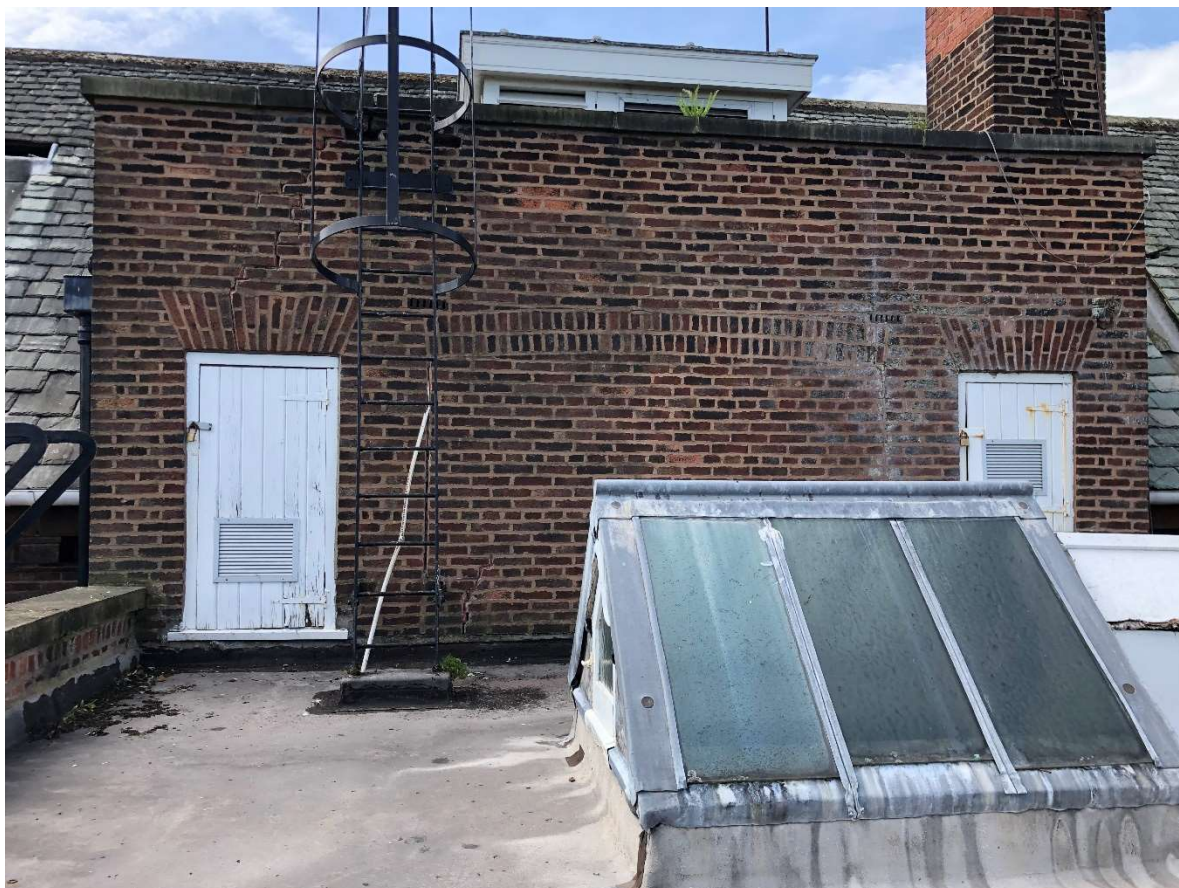
Photo 5: View of roof 4 showing glass lantern light over stairwell.
