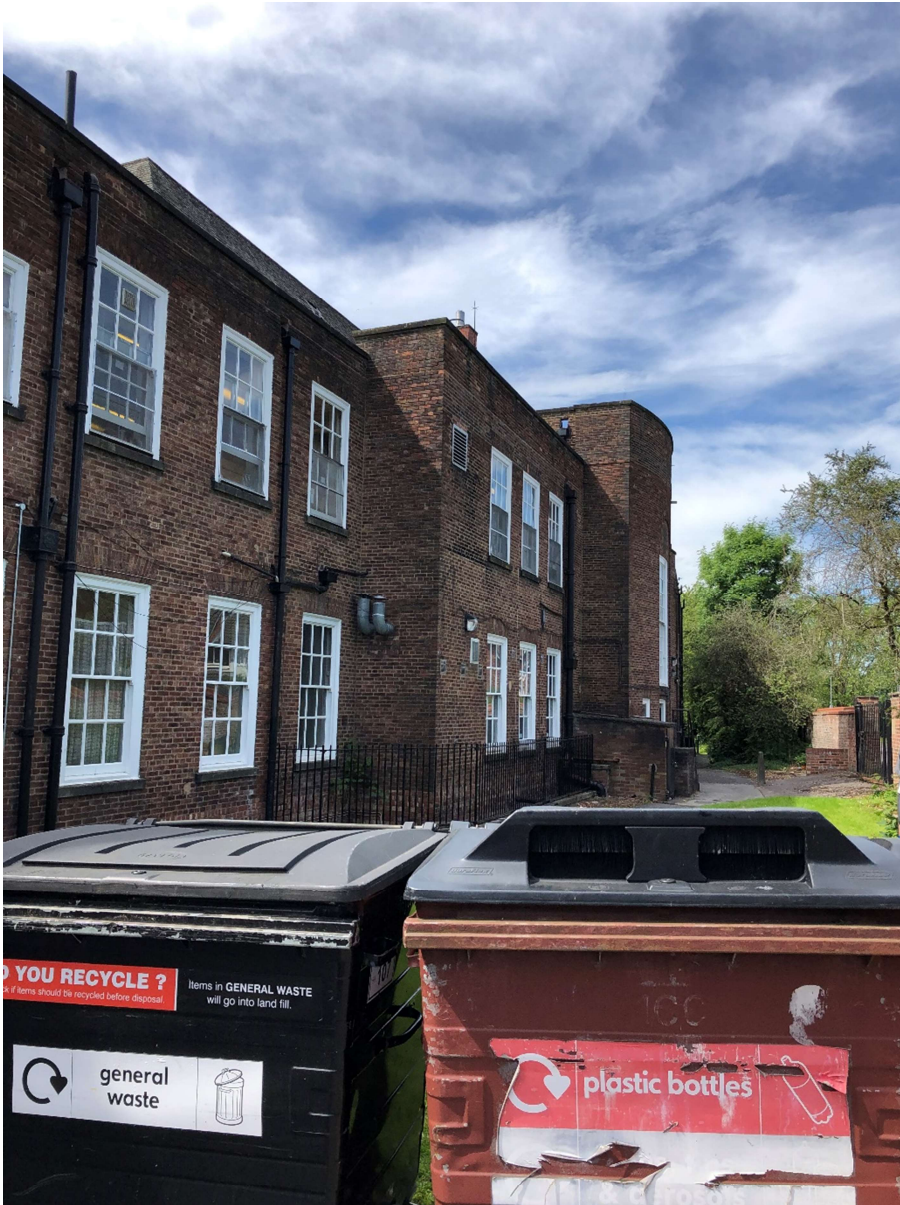
Photo 1: Rear view showing parapet walls to asphalt flat roofs.
