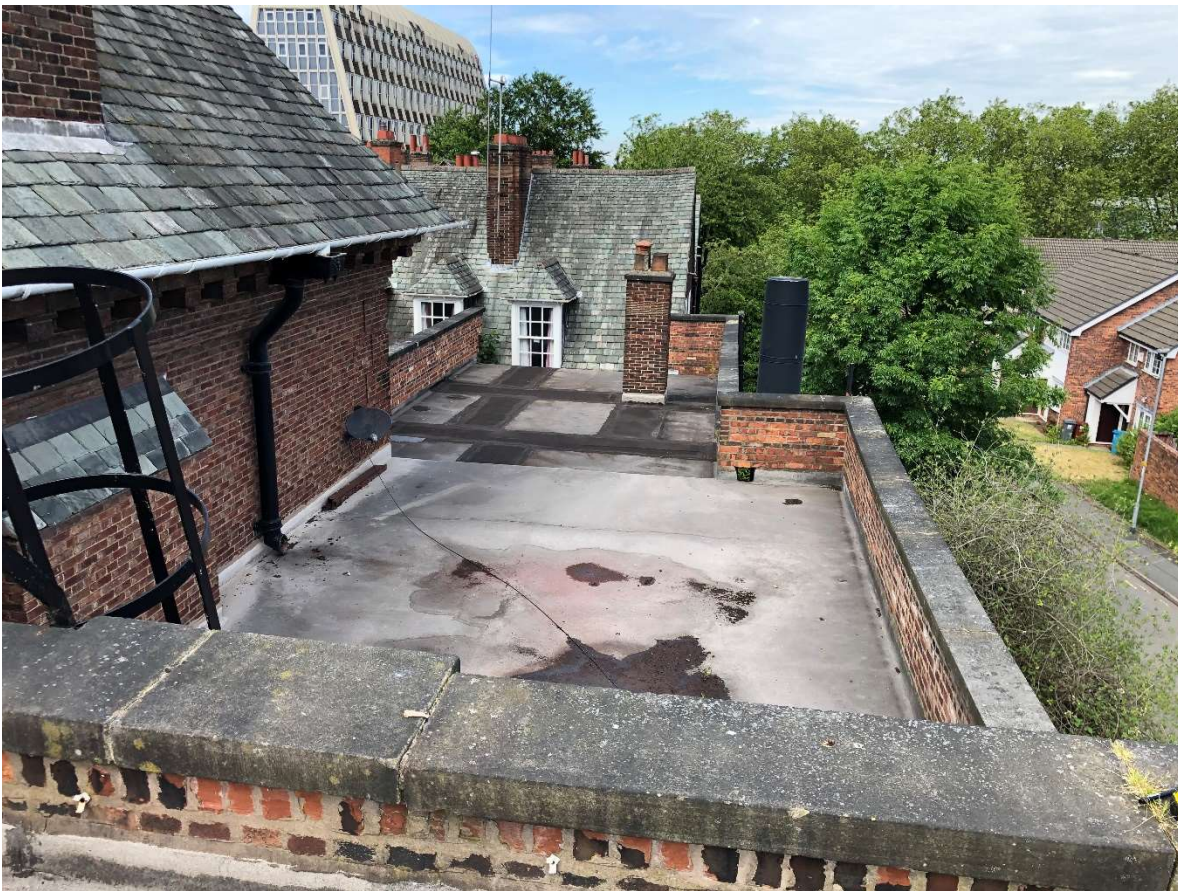
Photo 3: View of roofs 1, 2 & 3, showing slate pitched roof and asphalt flat roofs with patch repairs.
