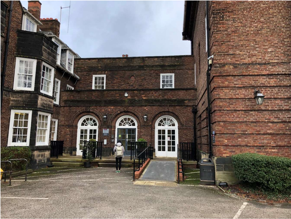
Photo 2: Front elevation showing parapet walls.
