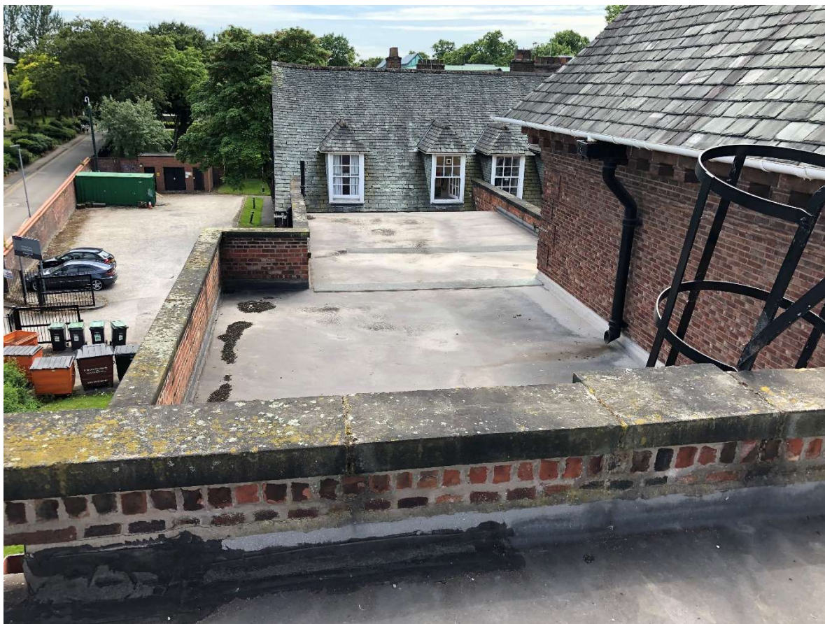
Photo 4: View of roofs 5, 6 & 7. Showing slate pitched roof and asphalt flat roofs with patch repairs.
