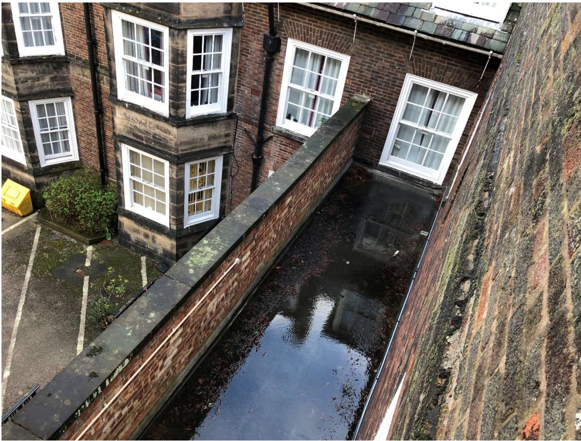
Photo 8: View of roof 9.
