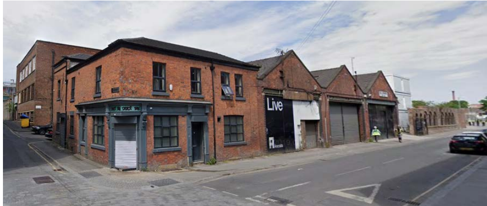
Figure 16: the Cross Keys public house, Jersey Street with the site to the right as seen today
