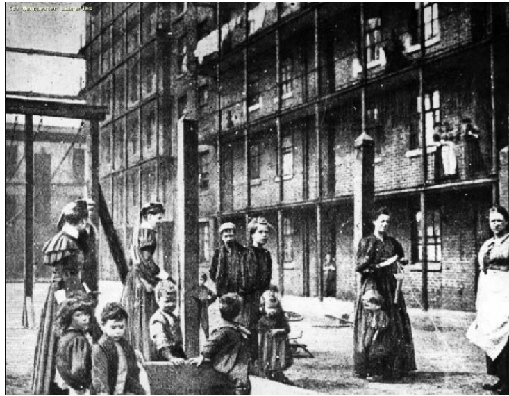
Figure 6: Jersey Street dwellings, close to the Site
