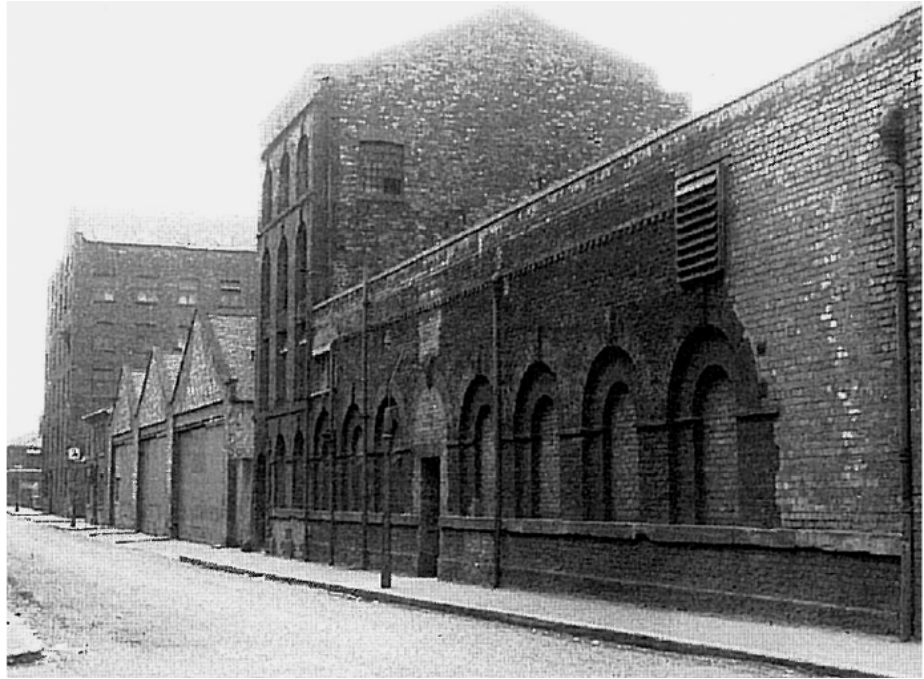
Figure 14: the single-storey perimeter wall and 4-story office building, Jersey Street, 1962
