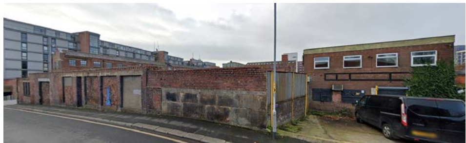
Figure 20: Site boundary wall, Poland Street (2020), showing white stone blocks of old canal bridge in centre of image
