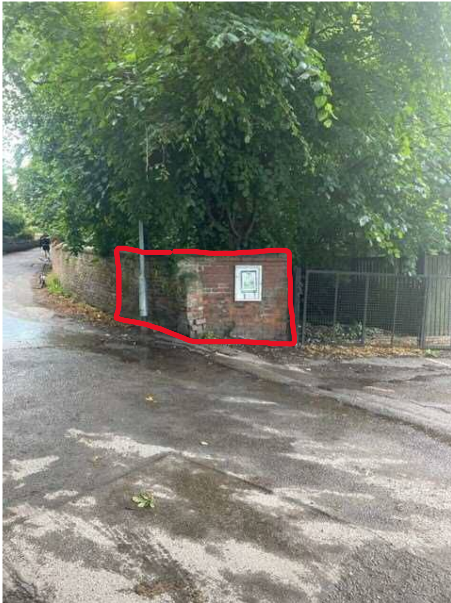
Photo 3. Red outline shows the proposed wall section to be removed
