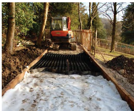
Fallbarrow Park, Windermere: CellWeb TRP® Installation
