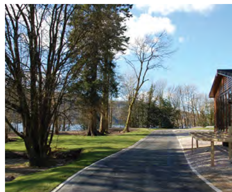
Fallbarrow Park, Windermere: Completed CellWeb TRP® Installation
